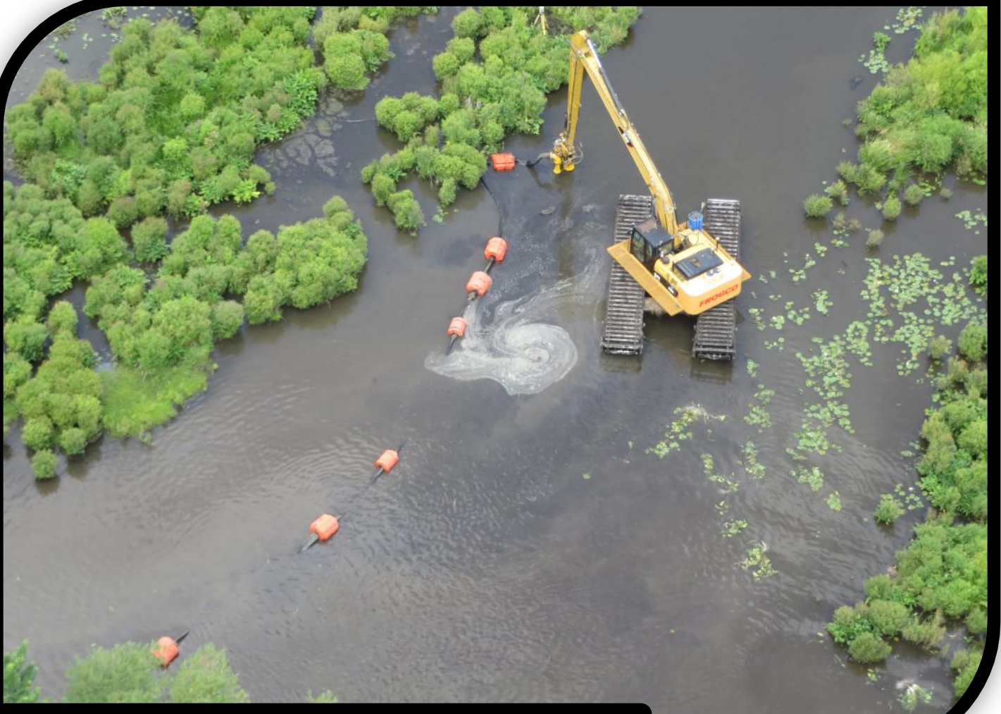
Dredging Operations in the Morrow Lake Delta (07/16/2014)
