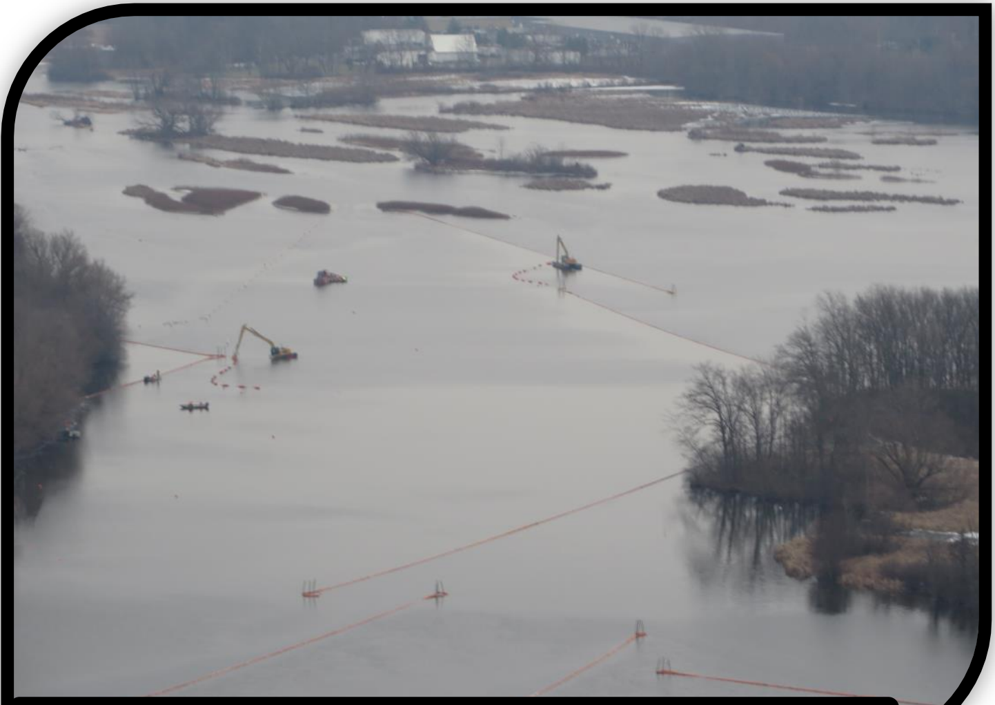
Morrow Lake Delta E4.0 Containment Removal Dredging Activities (11/26/2013)
