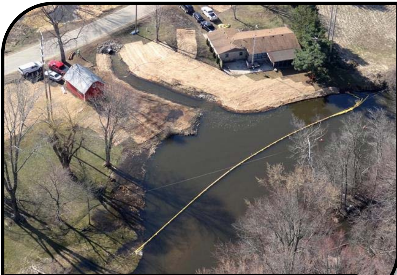
Confluence Excavation and Restoration Activities Completed
