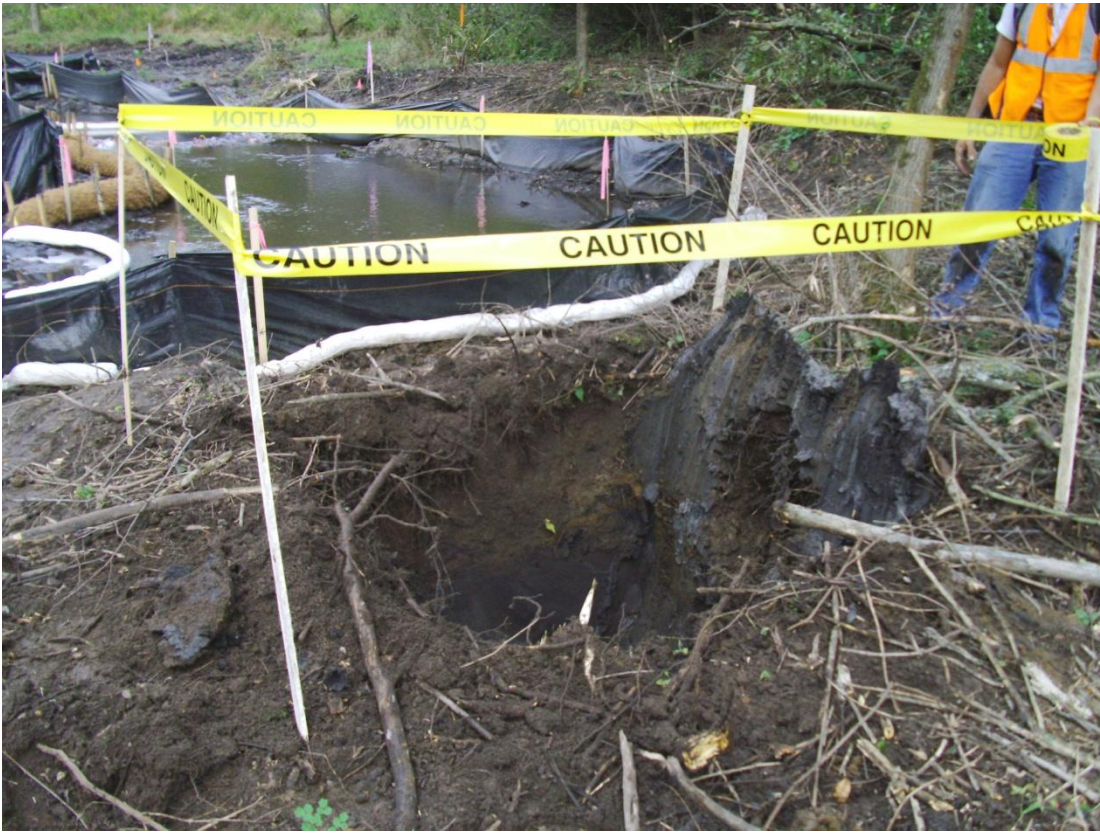
76+50R – 77+00R: Looking downstream (September 20, 2010)
