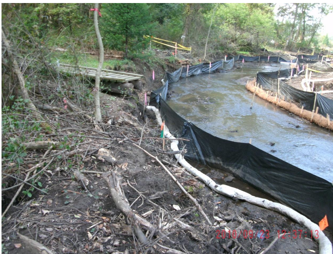
80+50L – 81+00L: Looking downstream (September 23, 2010)
