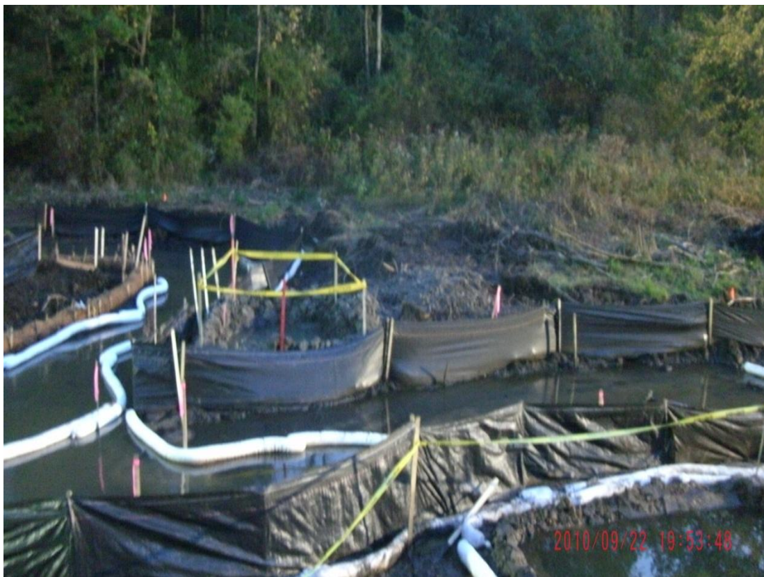
75+00L – 75+50L: Looking across Talmadge Creek (September 22, 2010)
