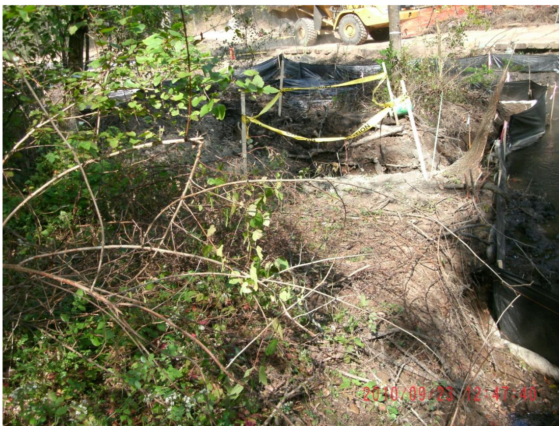
82+50L – 83+00L: Looking downstream (September 23, 2010)
