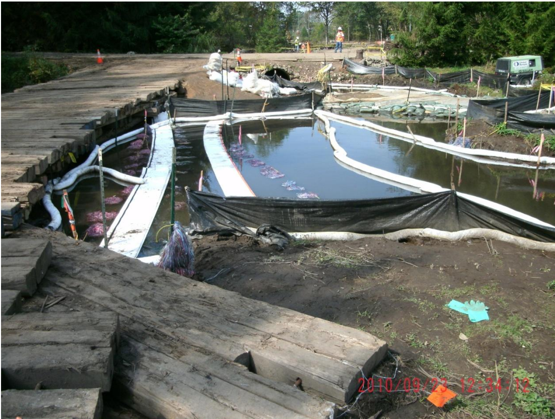
79+00L – 79+50L: Looking downstream (September 23, 2010)
