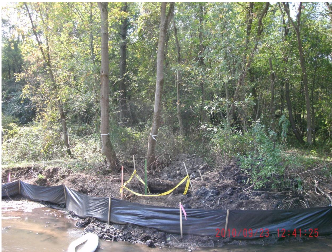
82+00L – 82+50L: Looking across Talmadge Creek (September 23, 2010)
