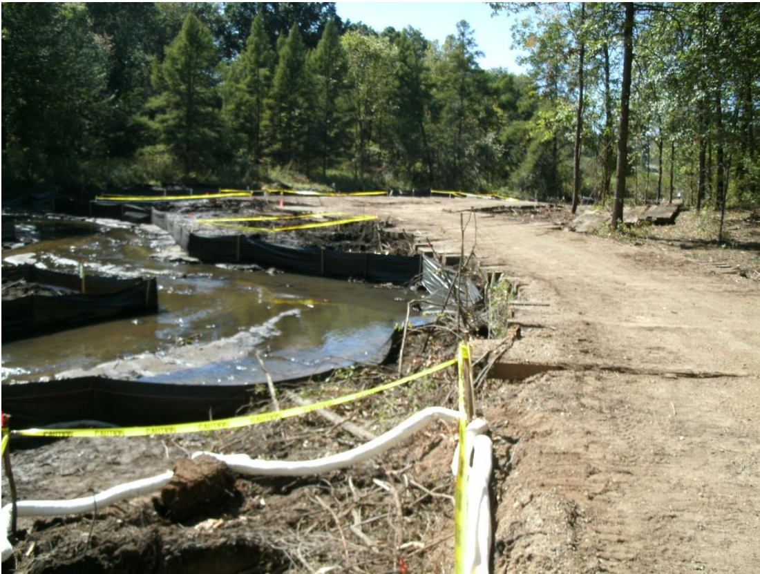
80+50R – 81+00R: Looking downstream (September 13, 2010)
