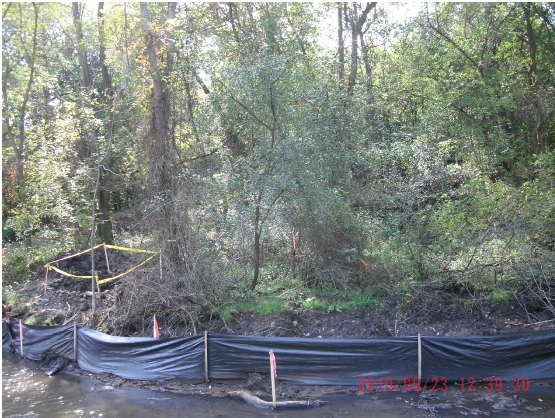
81+00L – 81+50L: Looking across Talmadge Creek (September 23, 2010)
