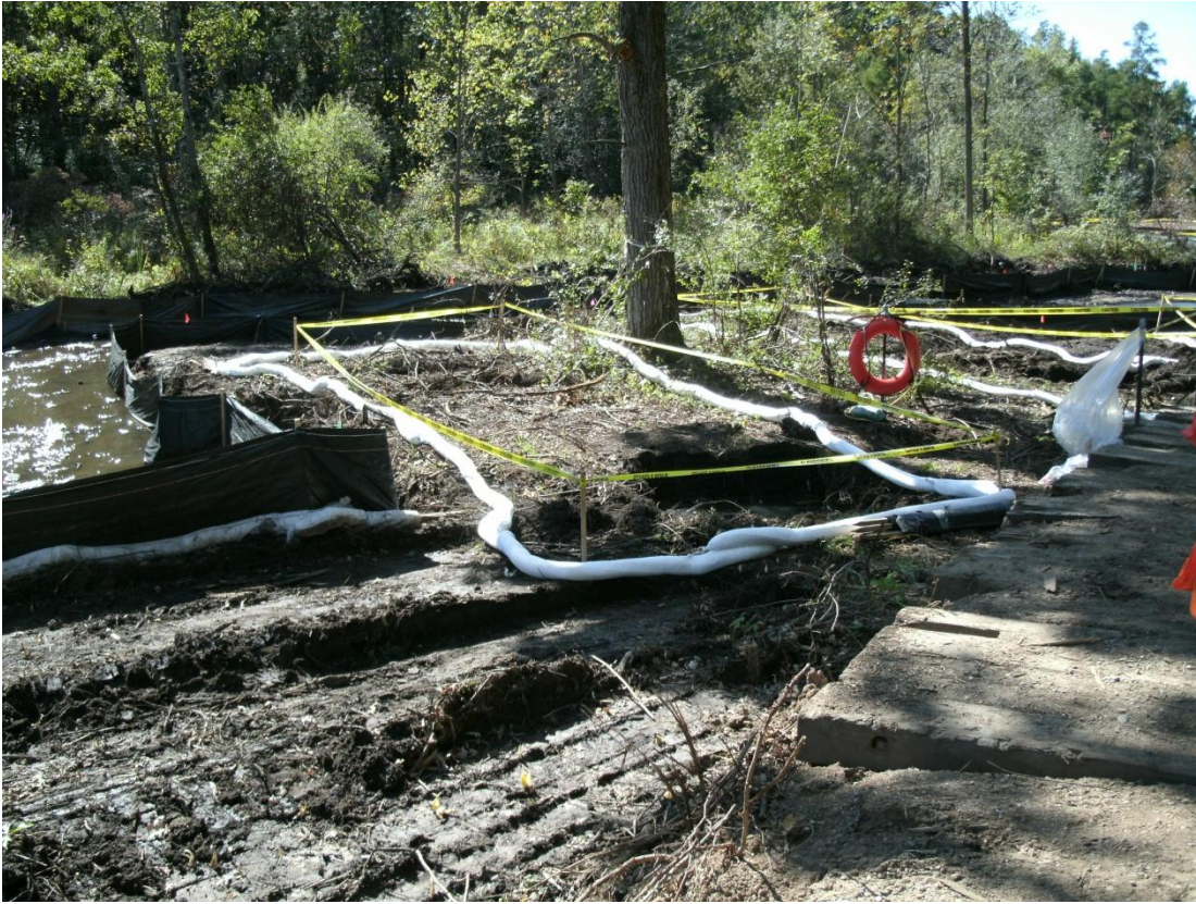
79+50R – 80+00R: Looking downstream (September 13, 2010)
