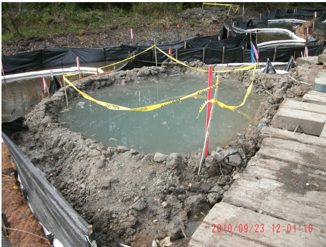
73+50R – 74+00R: Looking downstream (September 23, 2010)
