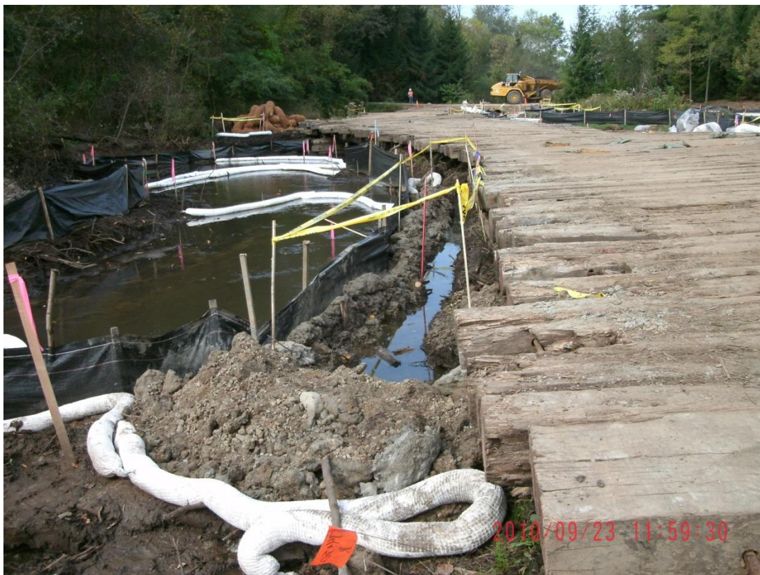
74+50R – 75+00R: Looking downstream (September 23, 2010)
