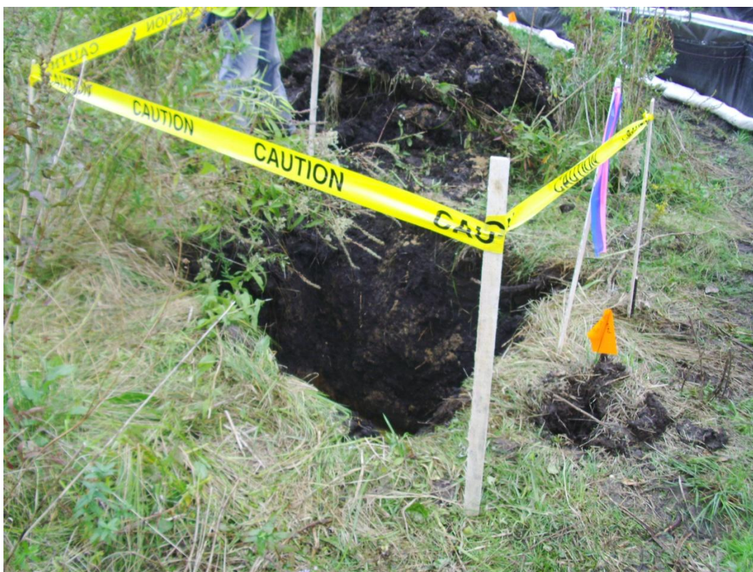
76+00R - 76+50R: Looking toward Talmadge Creek (September 20, 2010)
