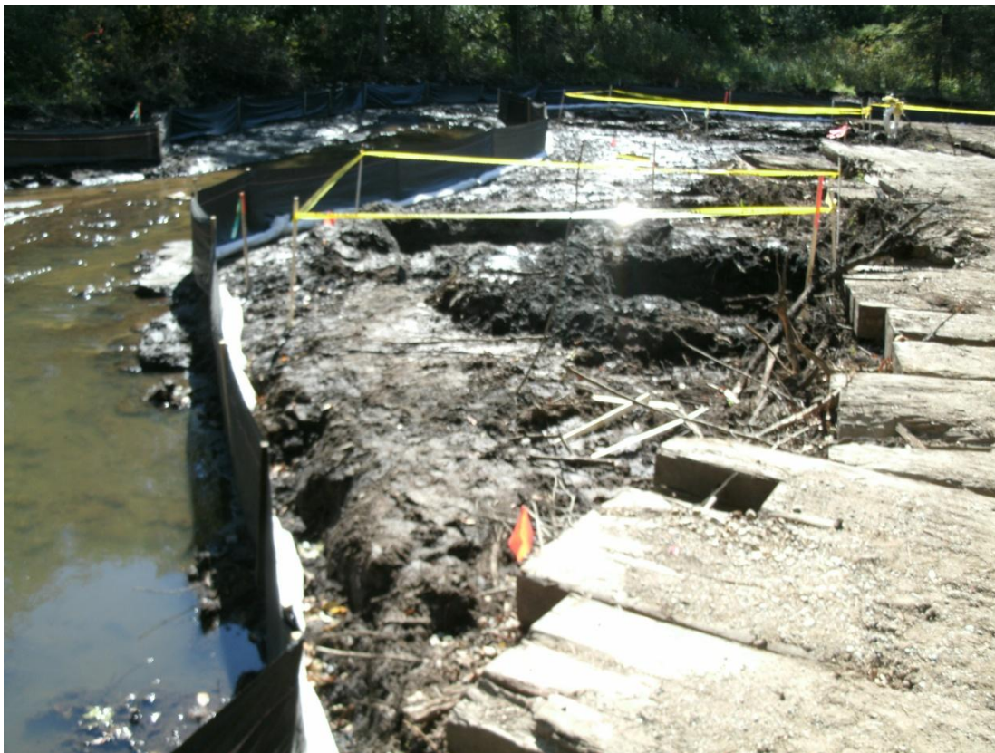
81+50R – 82+00R: Looking downstream (September 13, 2010)
