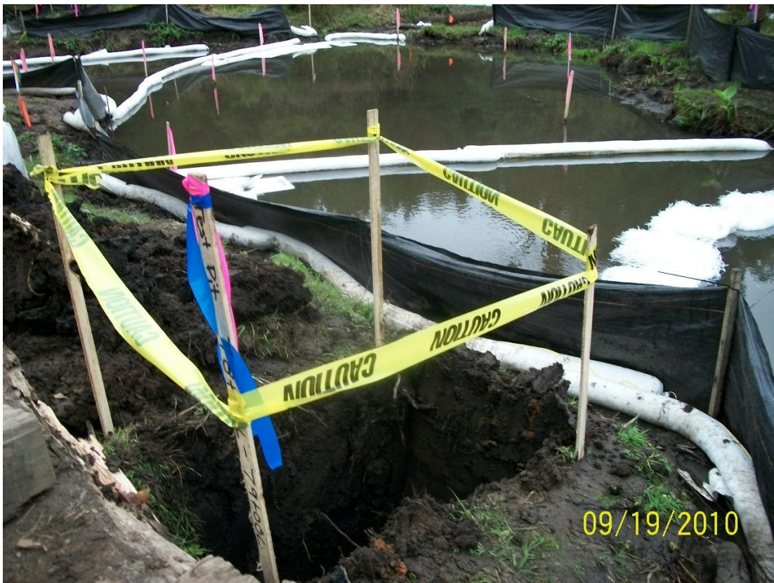
78+50L – 79+00L: Looking downstream (September 19, 2010)
