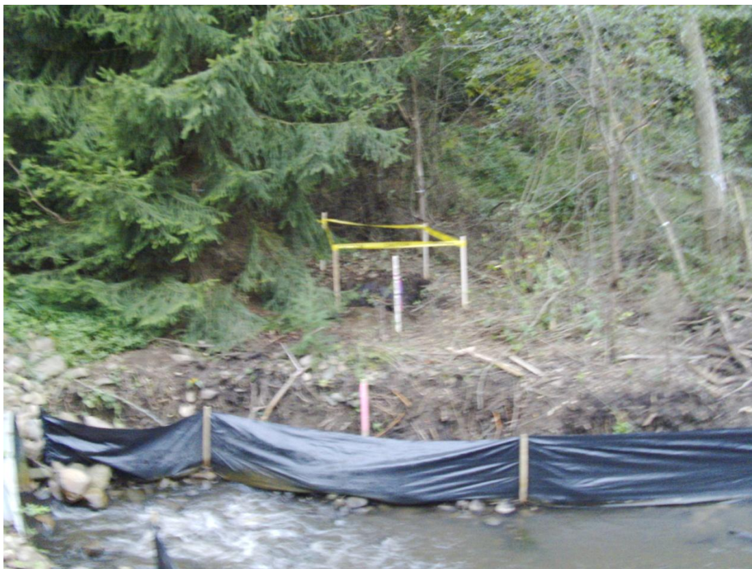
80+00L – 80+50L: Looking across Talmadge Creek (September 20, 2010)
