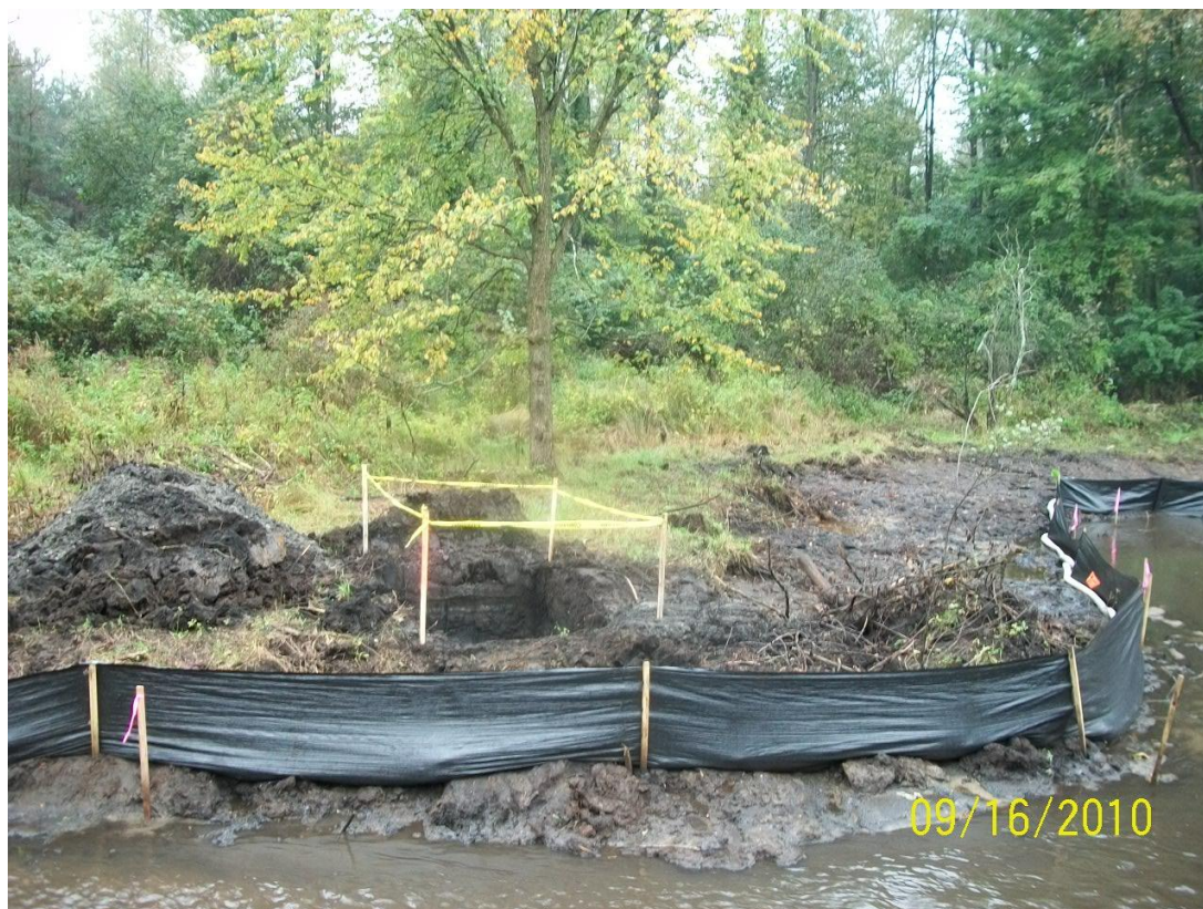
75+50L – 76+00L: Looking across Talmadge Creek (September 16, 2010)
