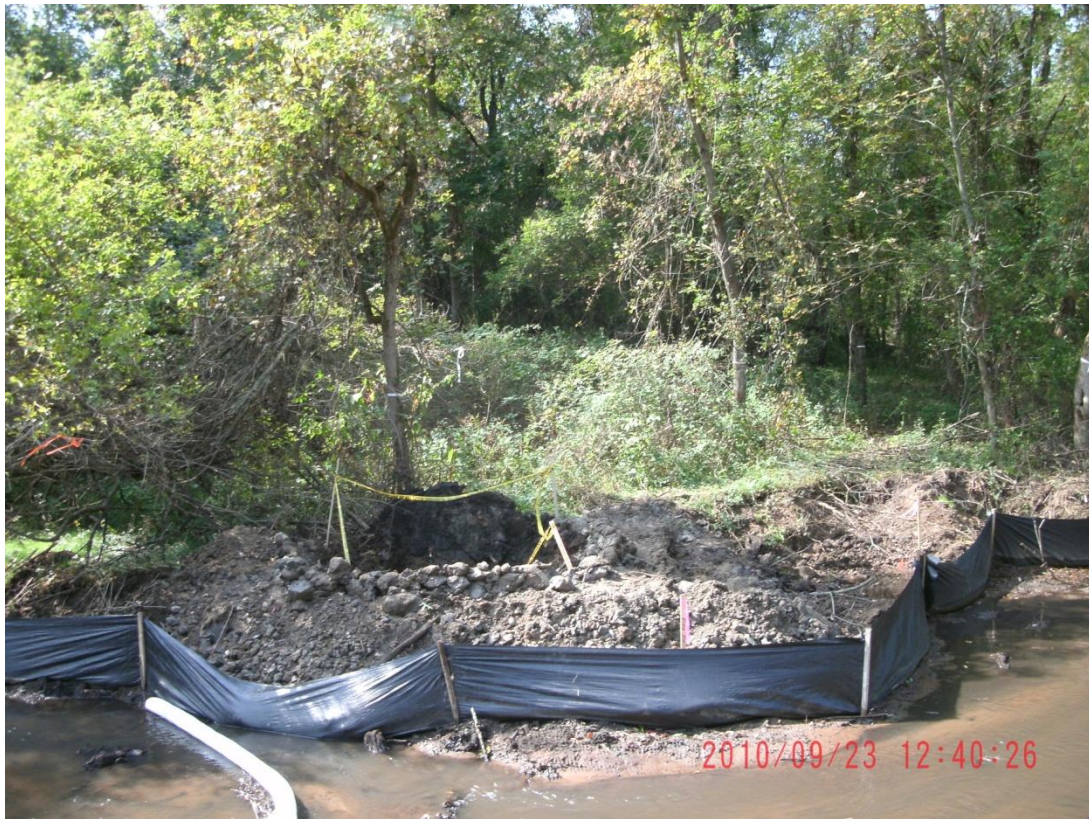
81+50L – 82+00L: Looking across Talmadge Creek (September 23, 2010)
