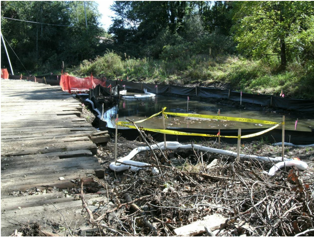
64+50R – 65+00R: Looking upstream (September 13, 2010)
