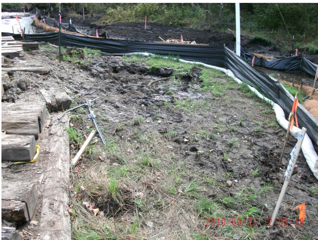
64+00R – 64+50R: Looking upstream (September 23, 2010)
