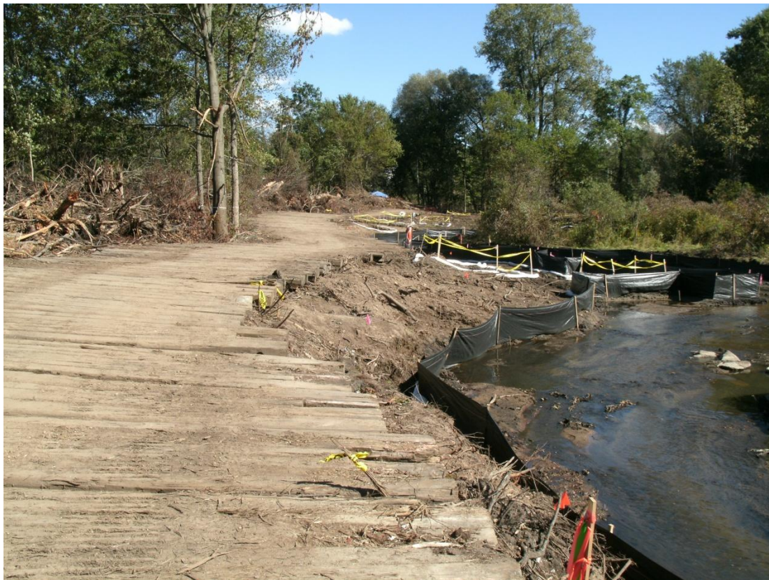
68+50R – 69+00R: Looking upstream (September 13, 2010)
