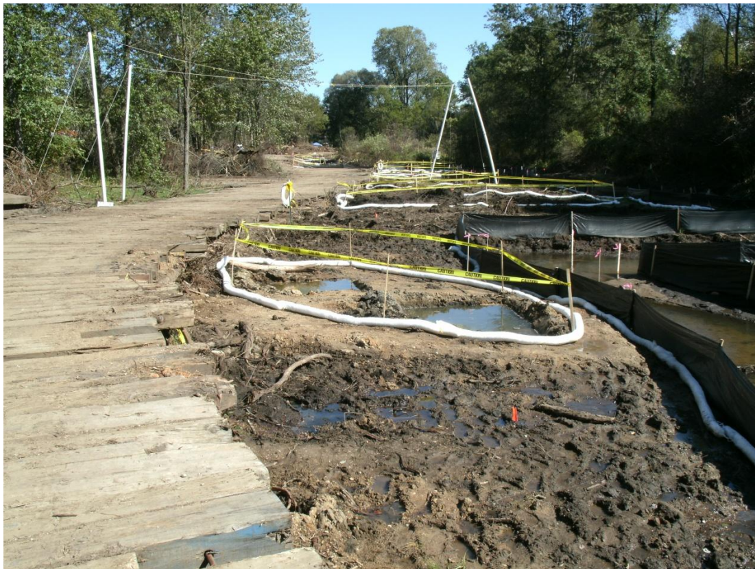
71+50R - 72+00R: Looking upstream (September 13, 2010)
