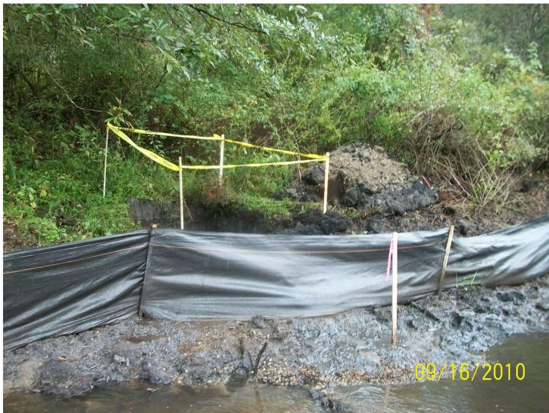
73+00L – 73+50L: Looking across Talmadge Creek (September 16, 2010)
