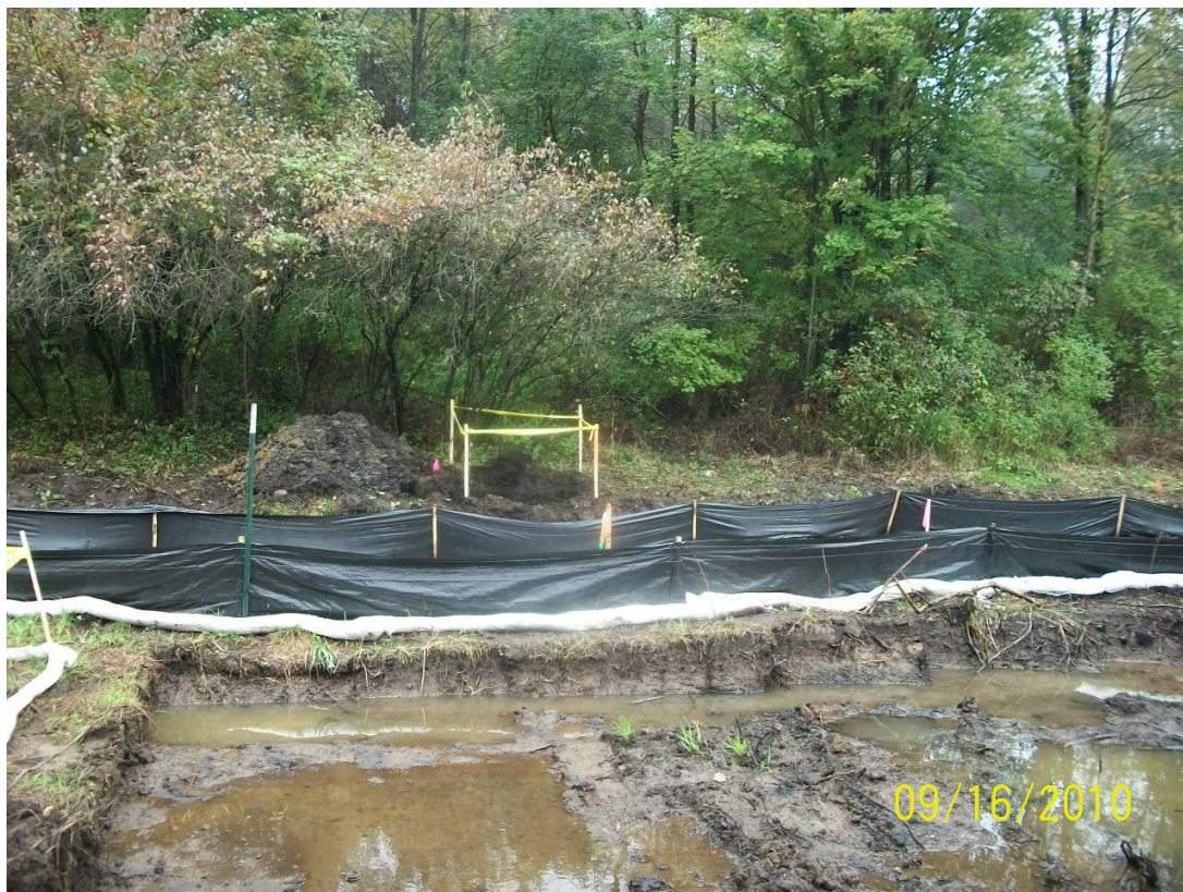
74+50L – 75+00L: Looking toward Talmadge Creek (September 16, 2010)
