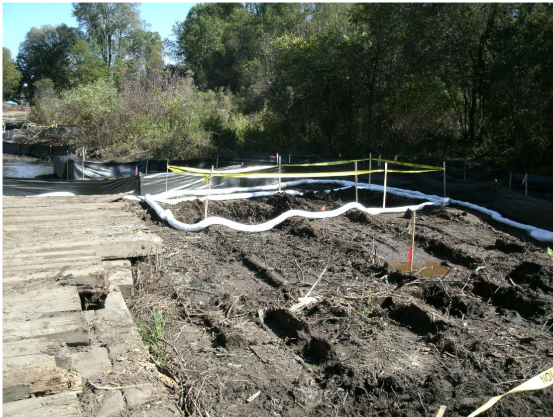
69+50R - 70+00R: Looking upstream (September 13, 2010)
