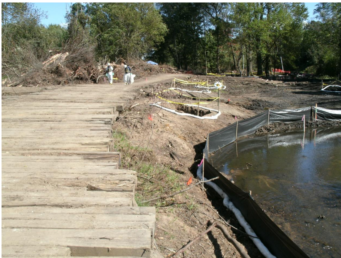
67+00R – 67+50R: Looking upstream (September 13, 2010)
