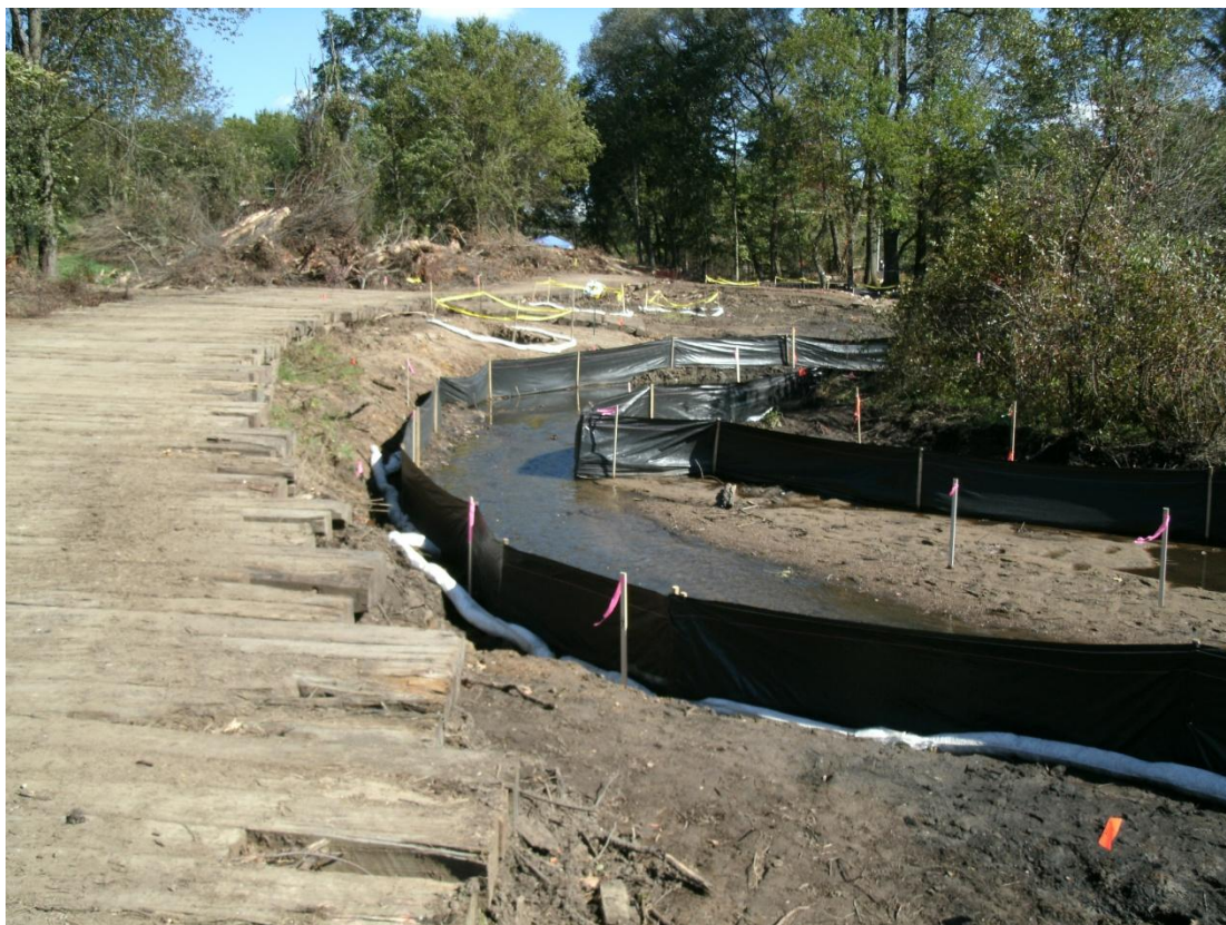
67+50R - 68+00R: Looking upstream (September 13, 2010)
