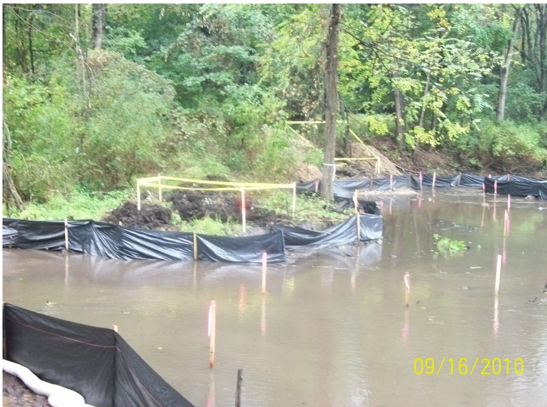
68+00L – 68+50L: Looking across Talmadge Creek (September 16, 2010)
