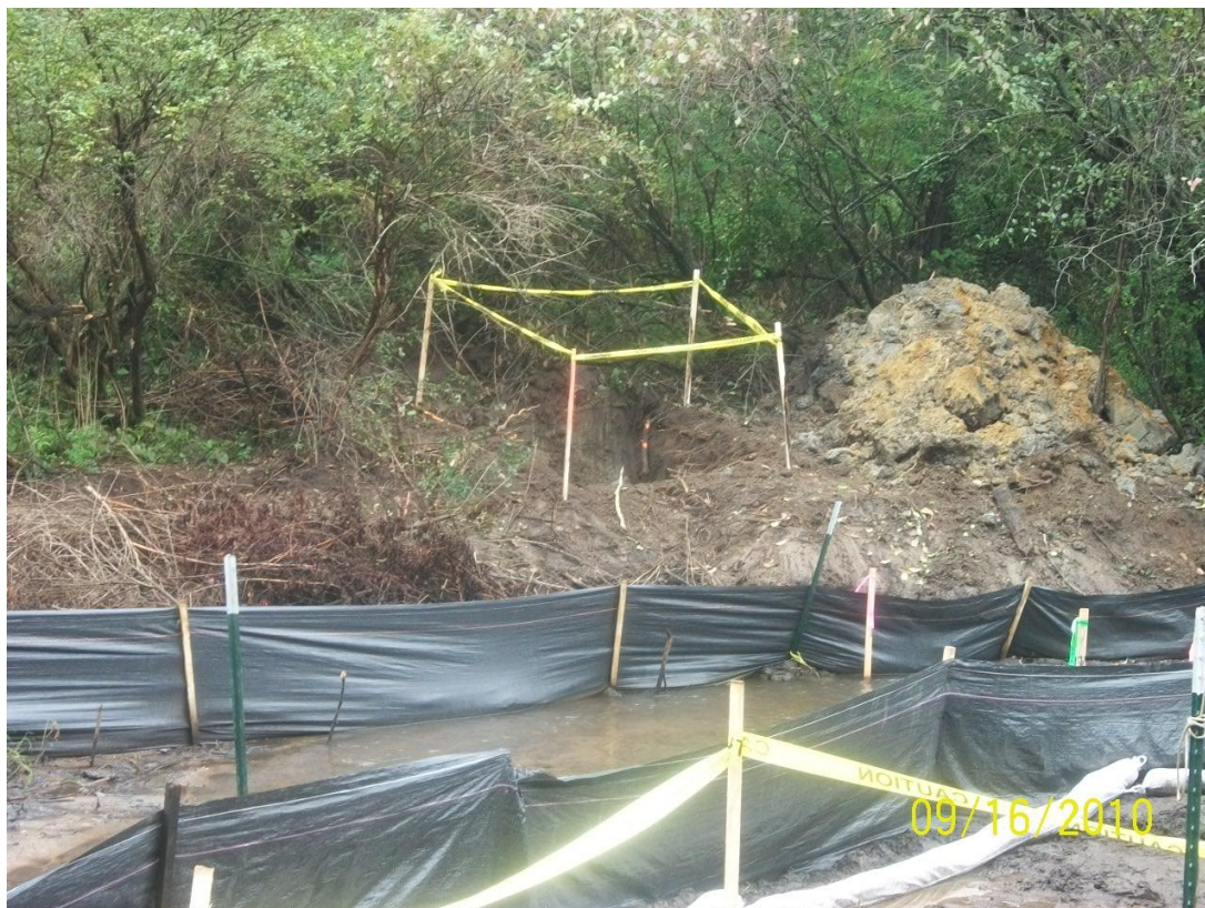
74+00L – 74+50L: Looking across Talmadge Creek (September 16, 2010)
