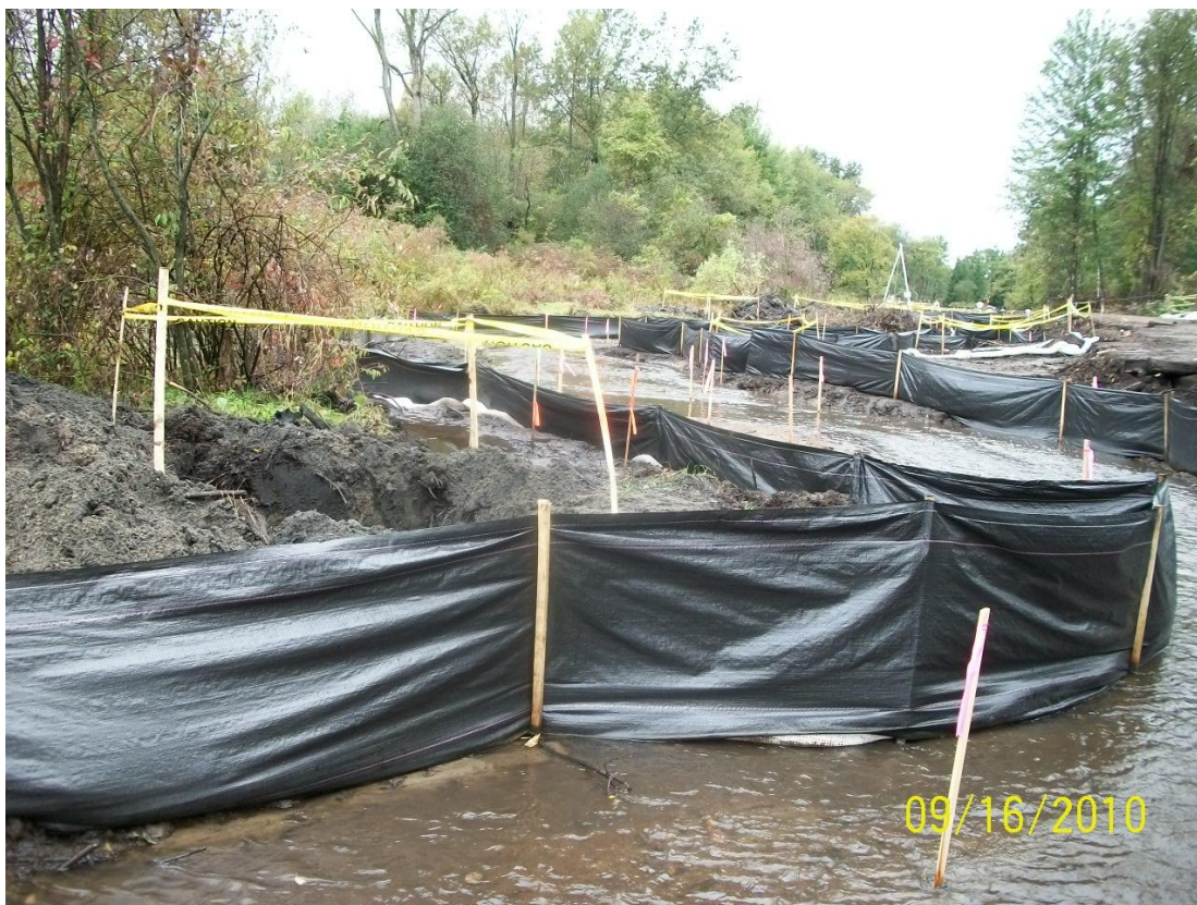
70+50L – 71+00L: Looking downstream (September 16, 2010)
