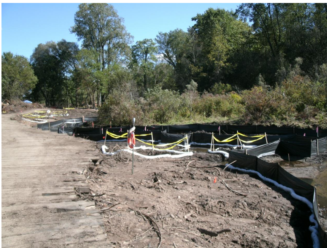
68+00R - 68+50R: Looking upstream (September 13, 2010)
