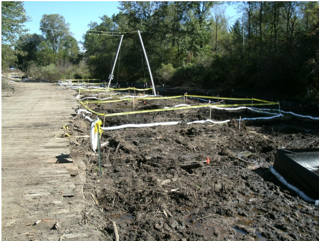
71+00R – 71+50R: Looking upstream (September 13, 2010)
