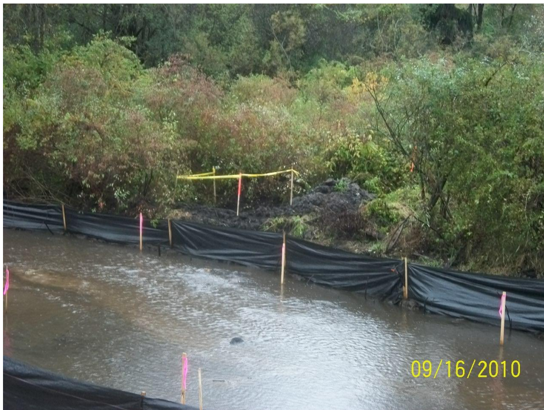
70+00L – 70+50L: Looking across Talmadge Creek (September 16, 2010)
