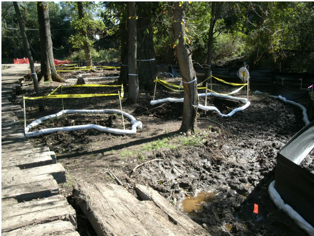
65+50R - 66+00R: Looking upstream (September 13, 2010)
