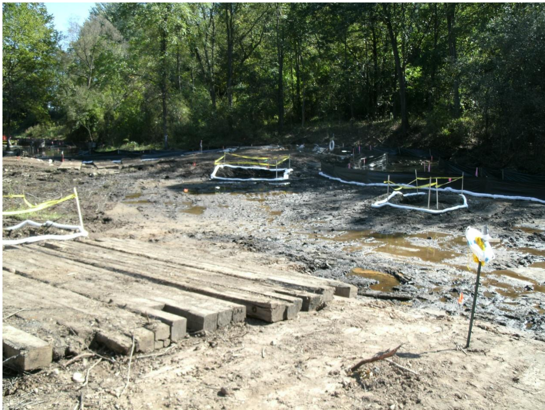
66+50R – 67+00R: Looking upstream (September 13, 2010)
