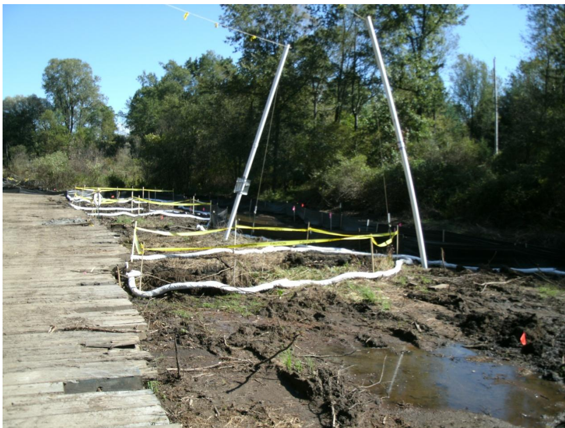
70+50R – 71+00R: Looking upstream (September 13, 2010)
