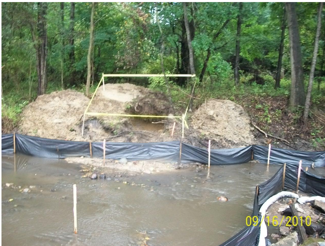
68+50L – 69+00L: Looking across Talmadge Creek (September 16, 2010)
