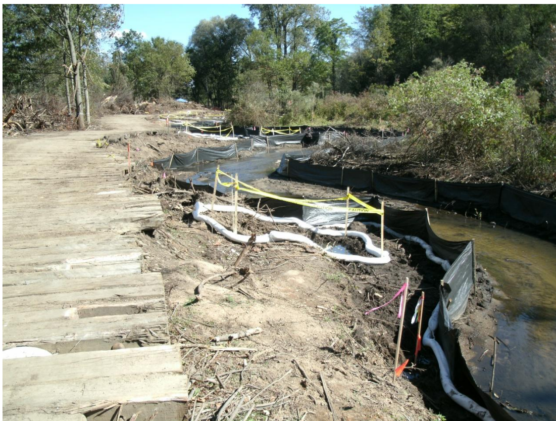
69+00R - 69+50R: Looking upstream (September 13, 2010)
