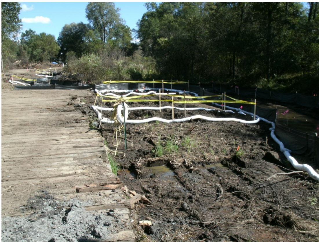
70+00R – 70+50R: Looking upstream (September 13, 2010)
