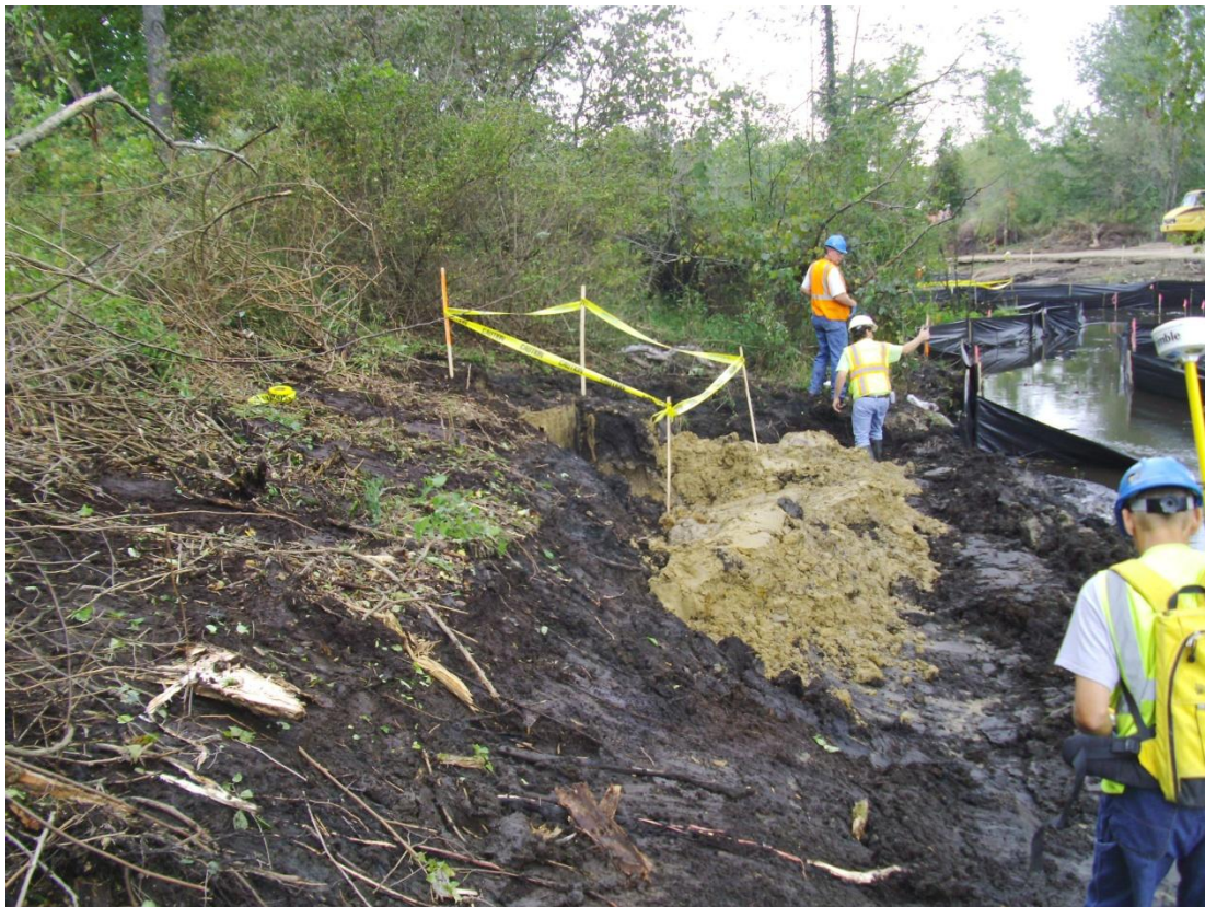
67+00L – 67+50L: Looking downstream (September 20, 2010)
