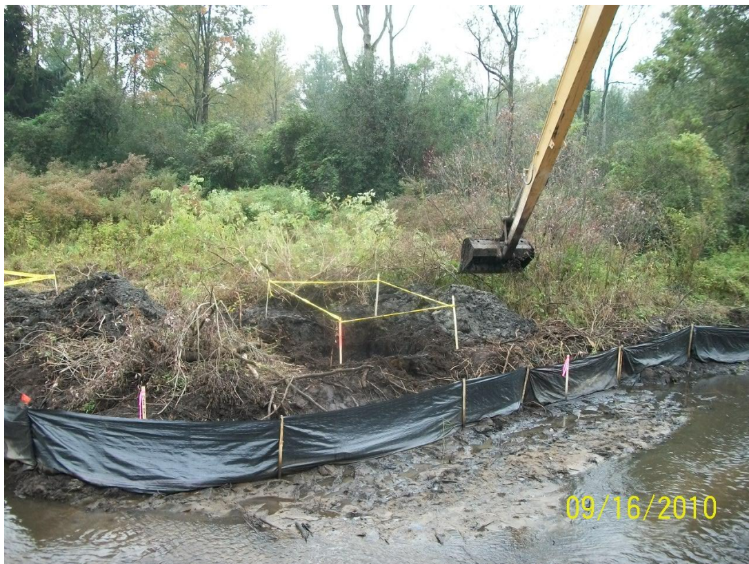
72+00L – 72+50L: Looking across Talmadge Creek (September 16, 2010)
