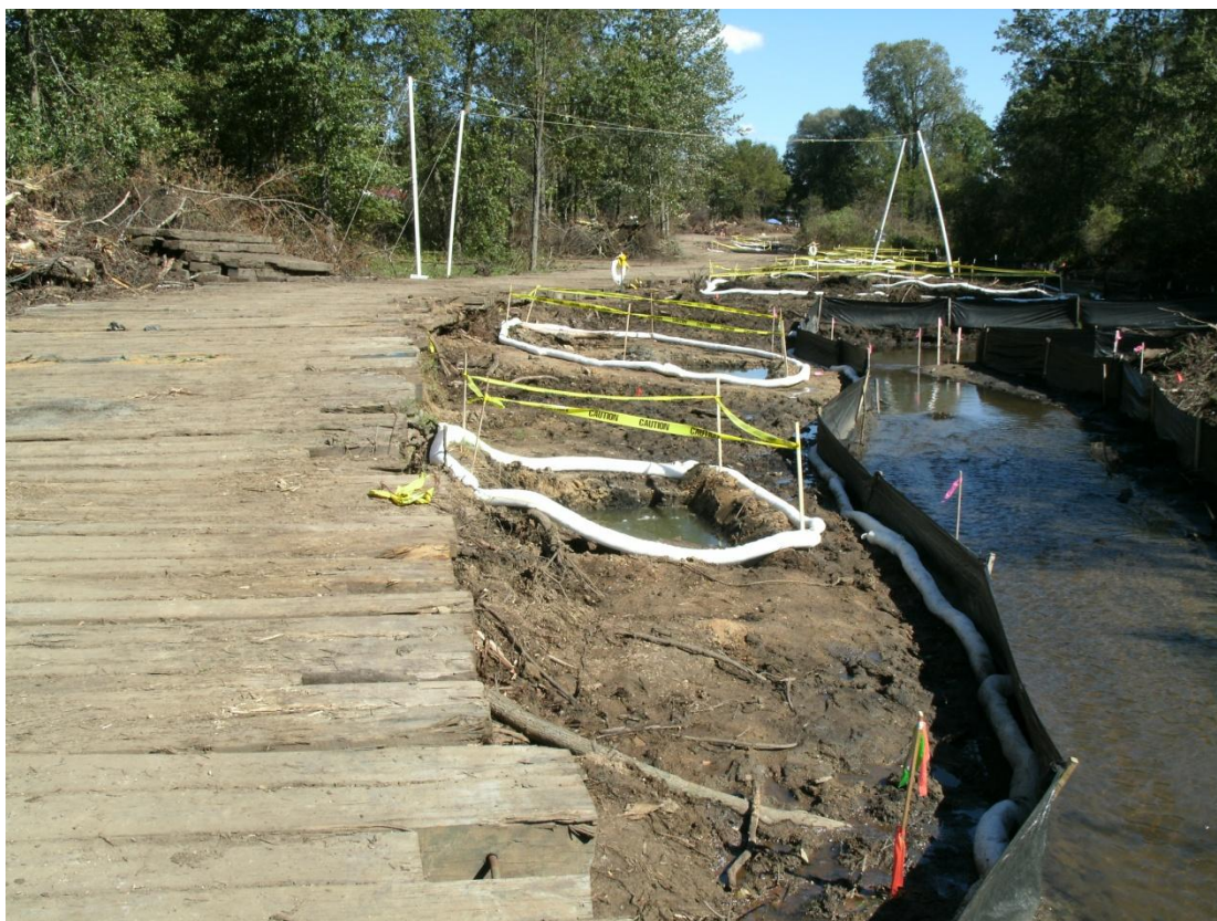
72+00R - 72+50R: Looking upstream (September 13, 2010)
