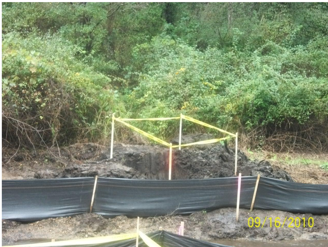
73+50L – 74+00L: Looking across Talmadge Creek (September 16, 2010)
