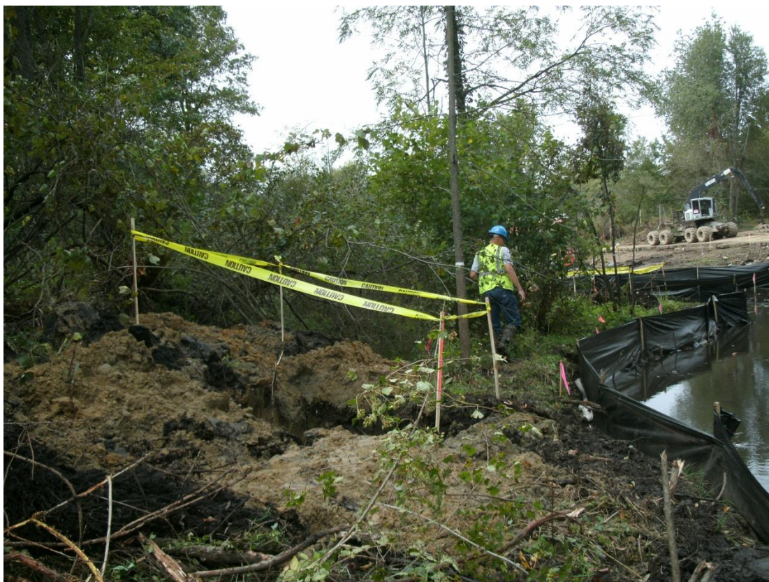
67+50L – 68+00L: Looking downstream (September 20, 2010)
