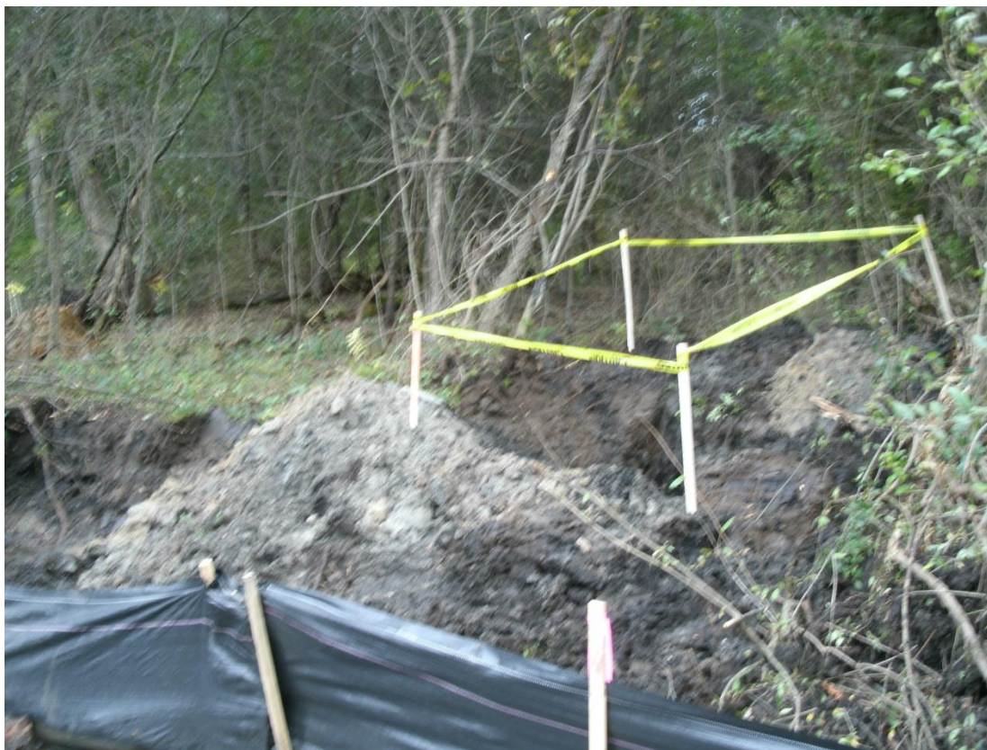
69+50L – 70+00L: Looking across Talmadge Creek (September 20, 2010)
