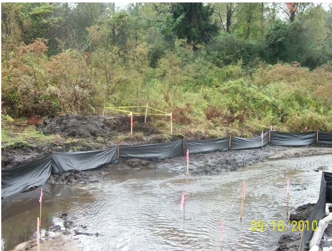
71+00L – 71+50L: Looking across Talmadge Creek (September 16, 2010)
