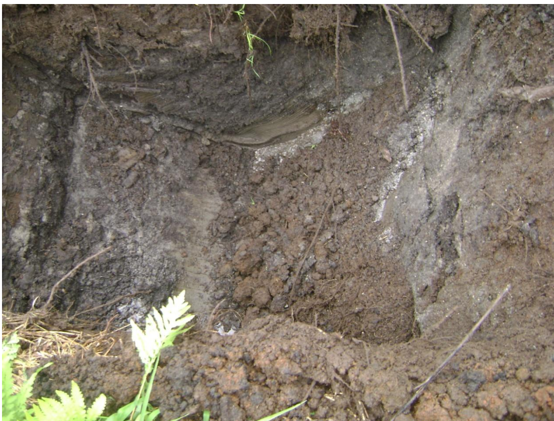
41+50R – 42+00R: Looking at 6-hour test pit (September 11, 2010)
