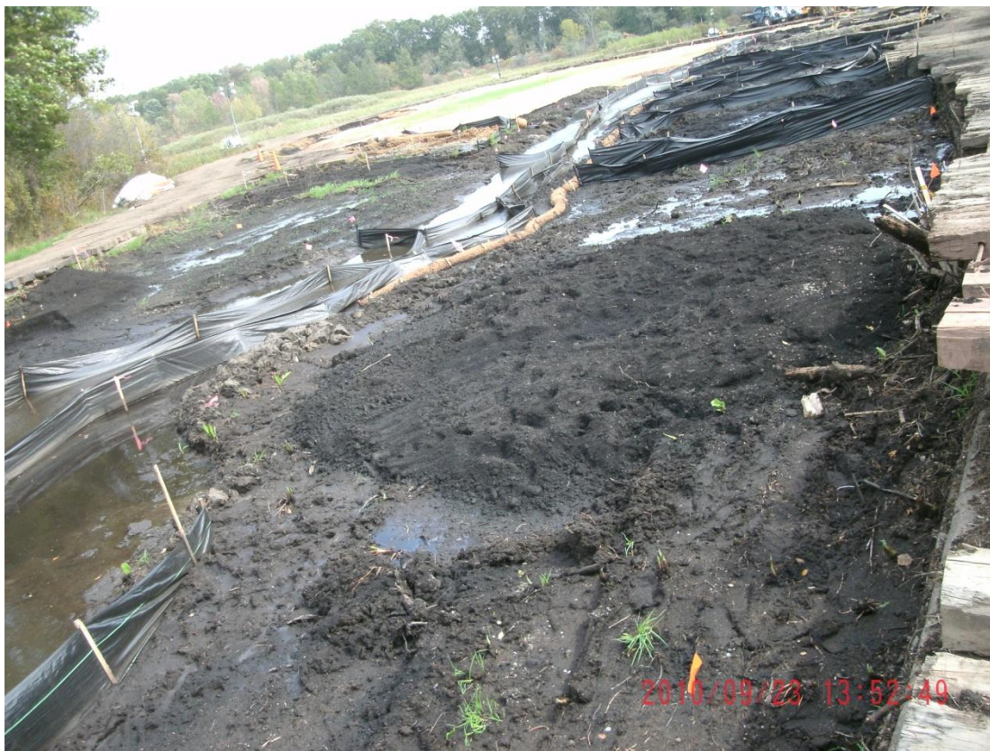
48+50L – 49+00L: Looking upstream (September 23, 2010)
