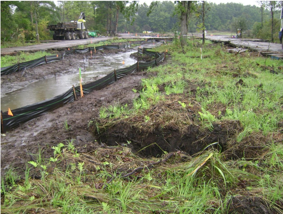
40+00R – 40+50R: Looking downstream (September 11, 2010)
