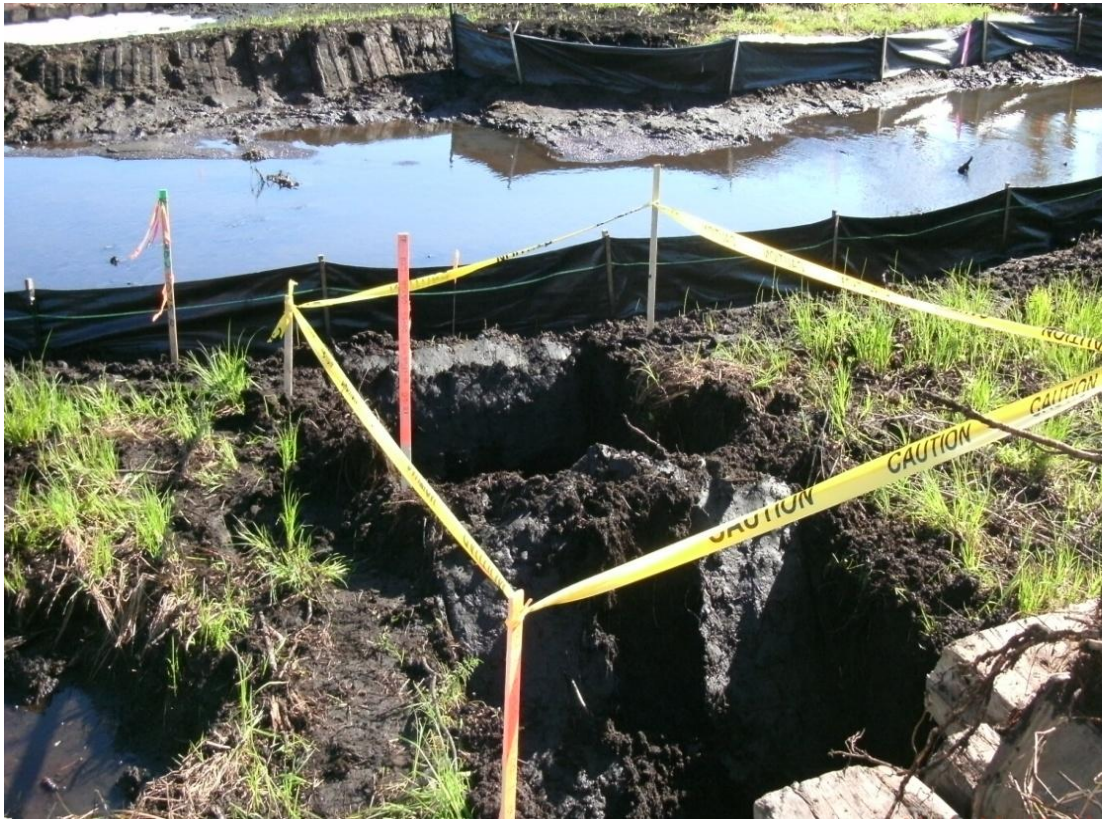
45+00L – 45+50L: Looking toward Talmadge Creek at 6-hour test pit (September 13, 2010)
