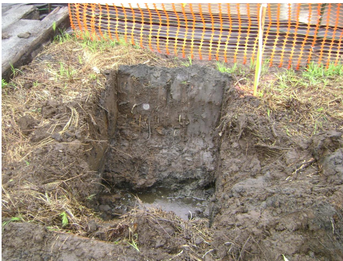
42+50R - 43+00R: Looking toward Talmadge Creek at 6-hour test pit (September 11, 2010)
