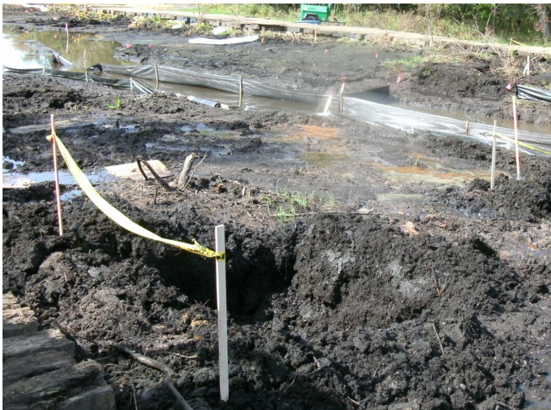
48+00L – 48+50L: Looking downstream (September 15, 2010)
