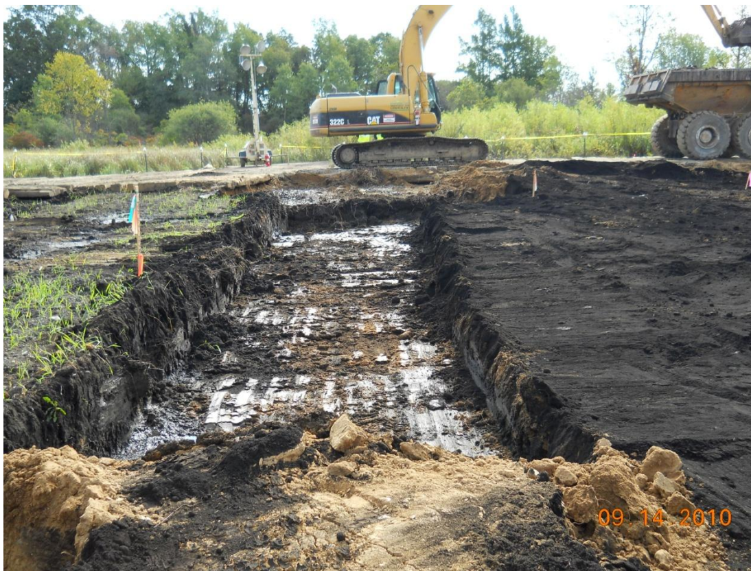
47+50R - 48+00R: Looking away from Talmadge Creek (September 14, 2010)
