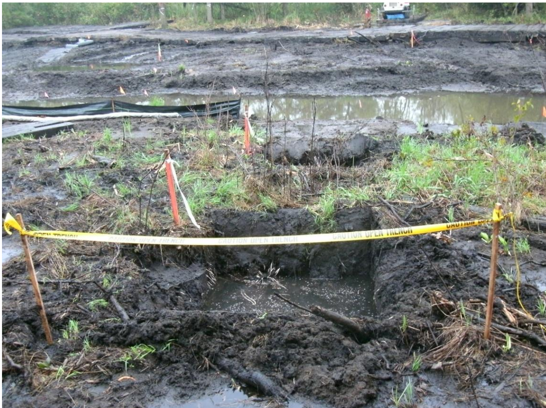
48+00R – 48+50R: Looking toward Talmadge Creek at 6-hour test pit (September 11, 2010)
