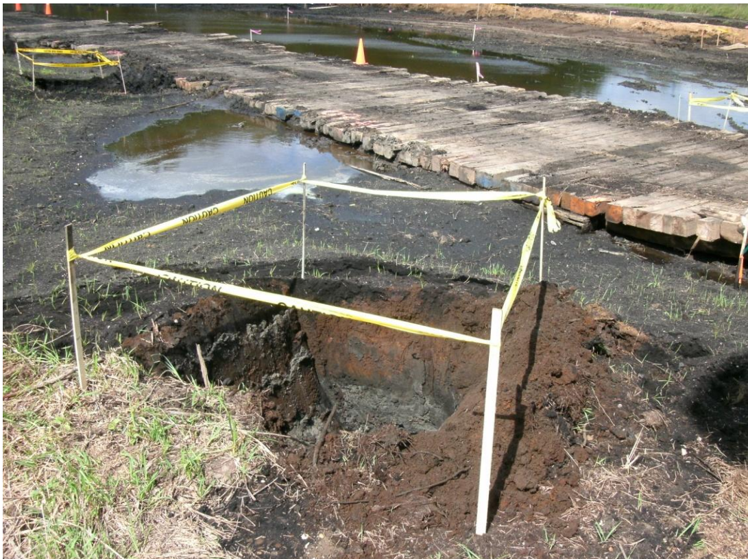
44+00R – 44+50R: Looking upstream (September 12, 2010)
