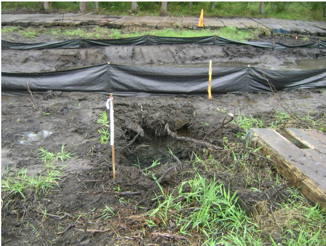
43+00R – 43+50R: Looking toward Talmadge Creek at 6-hour test pit (September 11, 2010)
