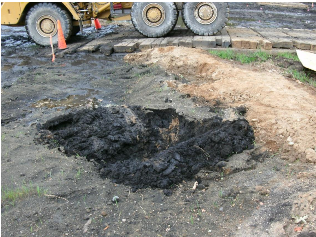
47+00R – 47+50R: Looking toward mat road at 6-hour test pit (September 11, 2010)
