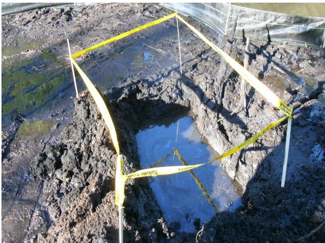
49+50L – 50+00L: Looking upstream (September 12, 2010)
