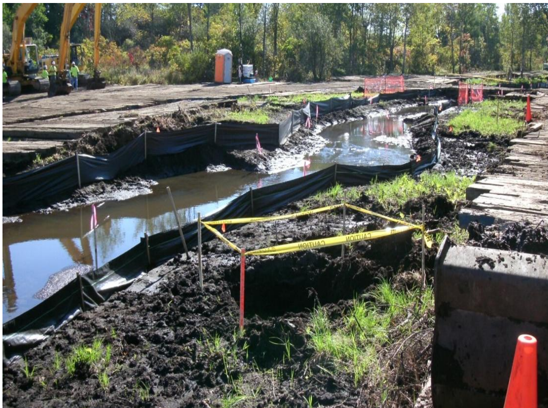
44+50L – 45+00L: Looking upstream (September 13, 2010)
