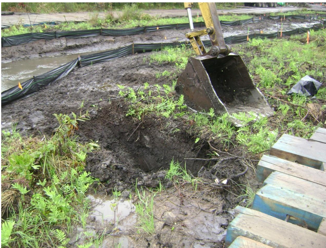
39+50R – 40+00R: Looking downstream (September 11, 2010)
