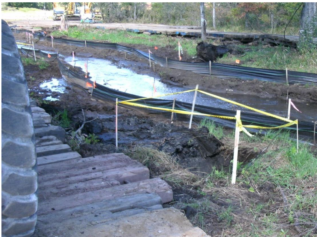
41+50L – 42+00L: Looking downstream (September 13, 2010)
