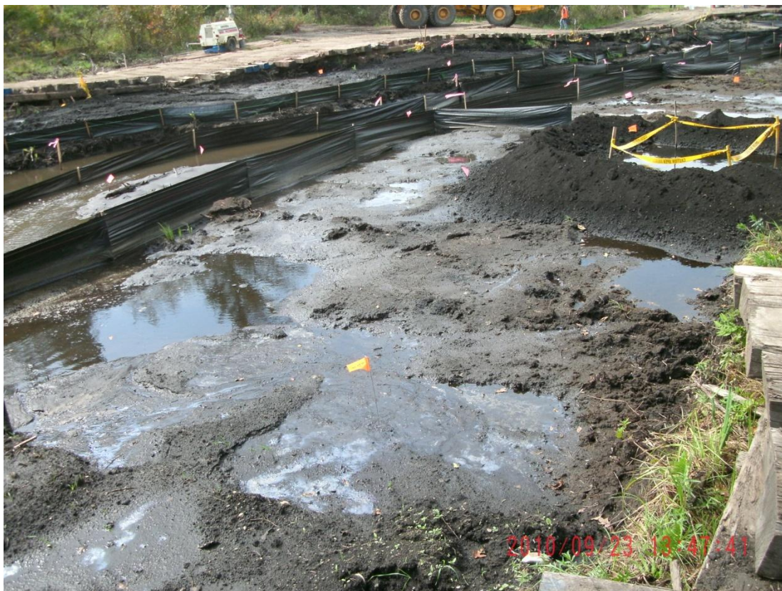
49+00L – 49+50L: Looking upstream (September 23, 2010)
