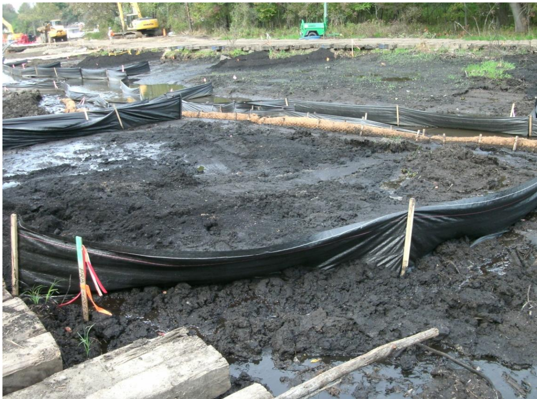
43+00L – 43+50L: Looking downstream (September 23, 2010)
