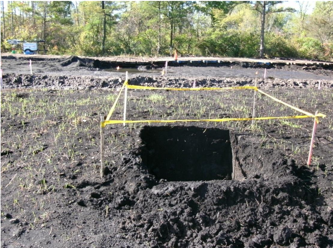
46+00R - 46+50R: Looking away from Talmadge Creek (September 12, 2010)
