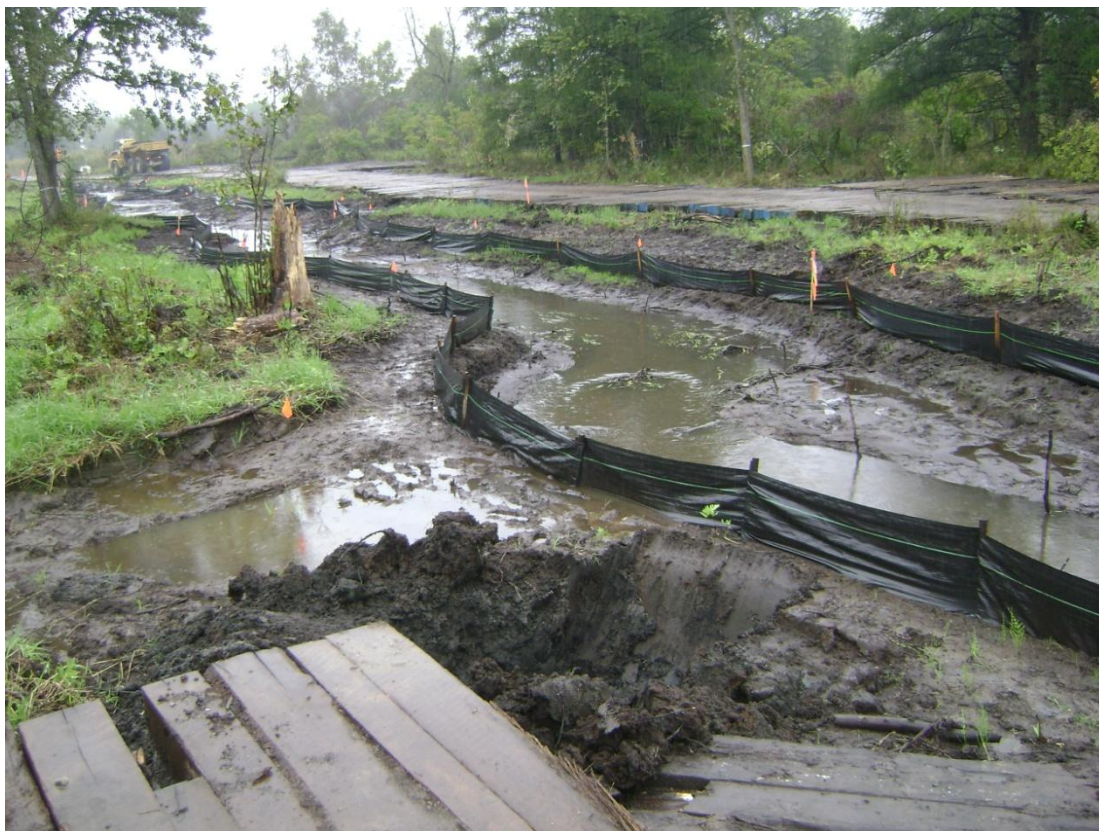
42+00R – 42+50R: Looking upstream (September 11, 2010)
