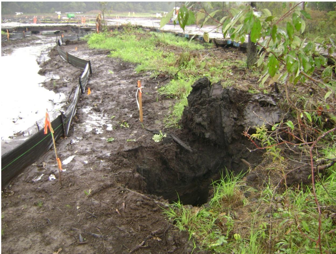
41+00R – 41+50R: Looking downstream (September 11, 2010)
