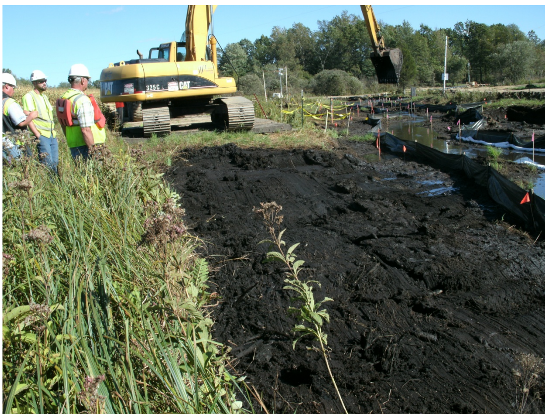
32+50R – 33+00R: Looking upstream (September 13, 2010)
