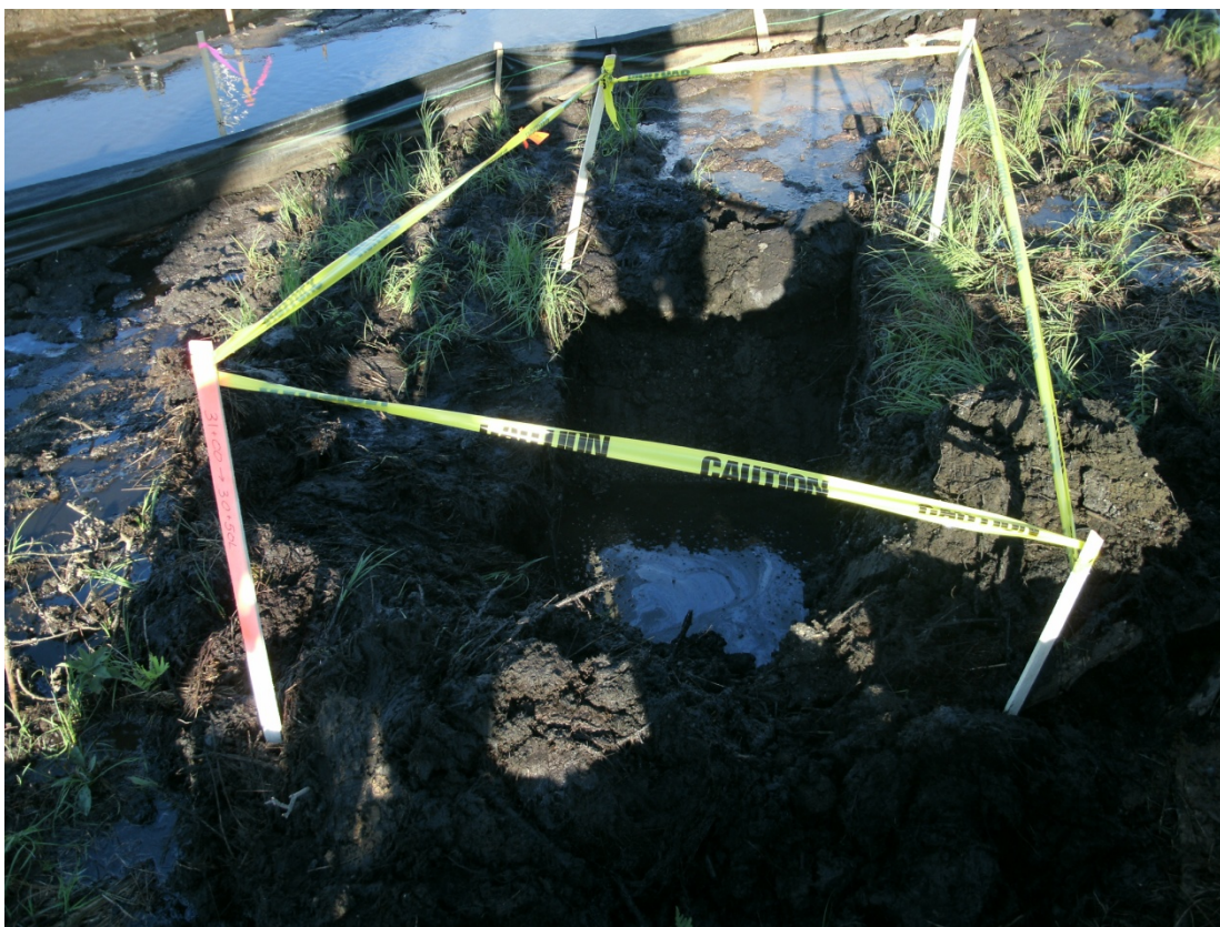
30+50L – 31+00L: Looking upstream at 6-hour test pit (September 14, 2010)
