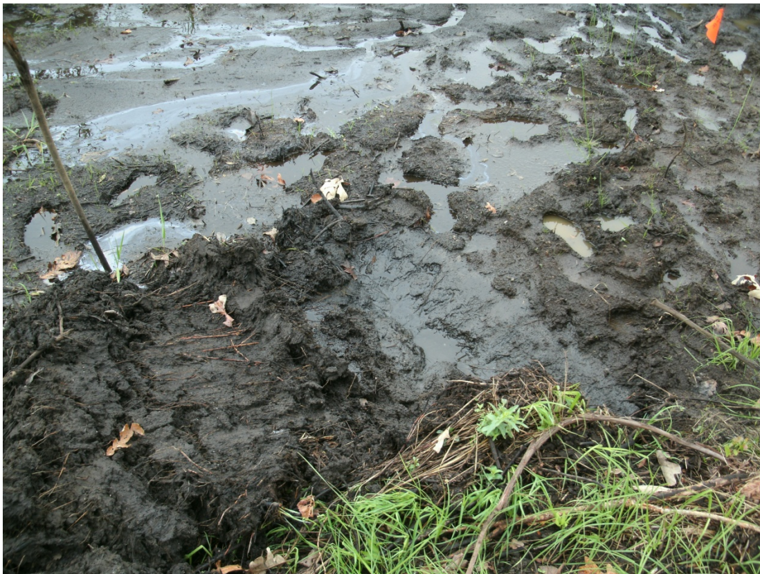
37+00R – 37+50R: Looking at 6-hour test pit (September 16, 2010)
