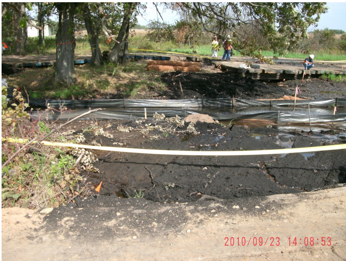
35+00L – 35+50L: Looking toward Talmadge Creek (September 23, 2010)
