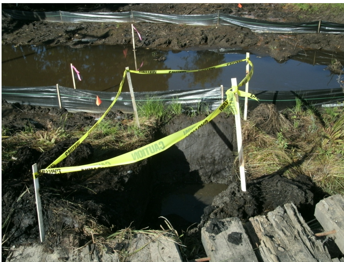
34+50L – 35+00L: Looking toward Talmadge Creek (September 14, 2010)
