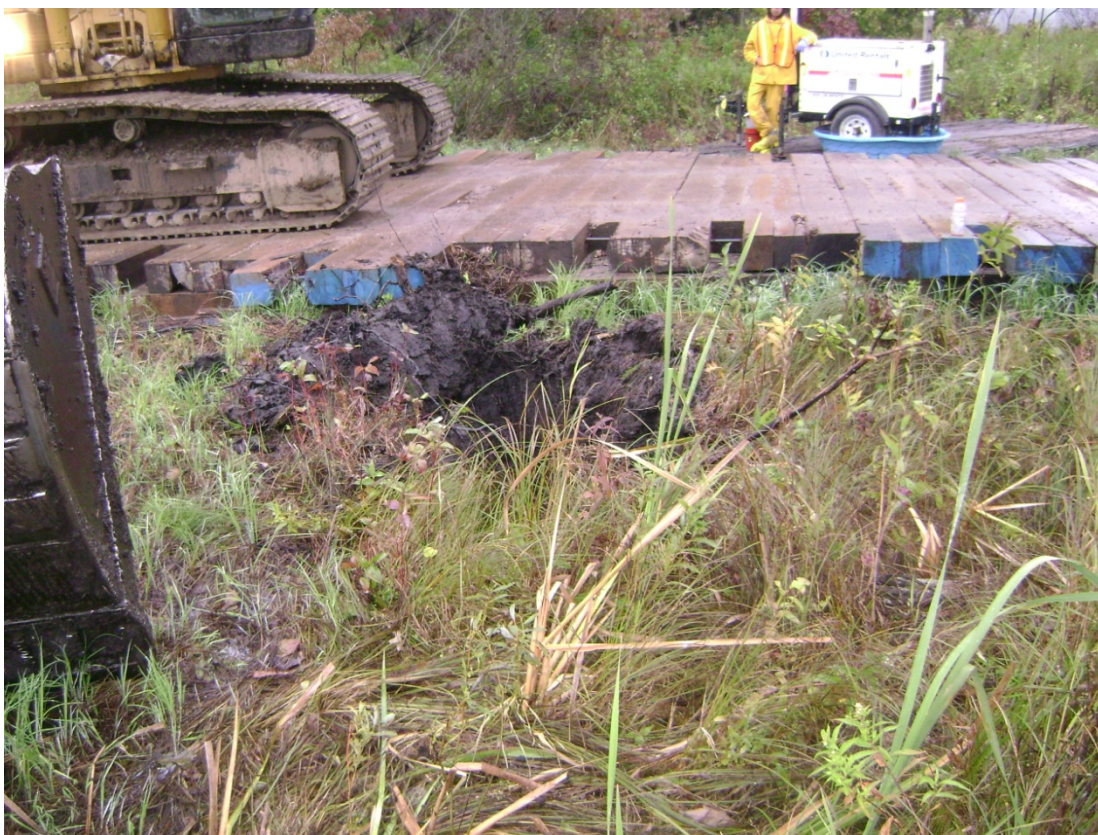
37+50R – 38+00R: Looking from Talmadge Creek toward mat road (September 11, 2010)
