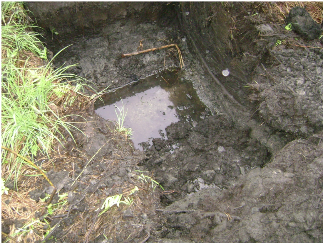
38+00R – 38+50R: Looking at 6-hour test pit (September 11, 2010)
