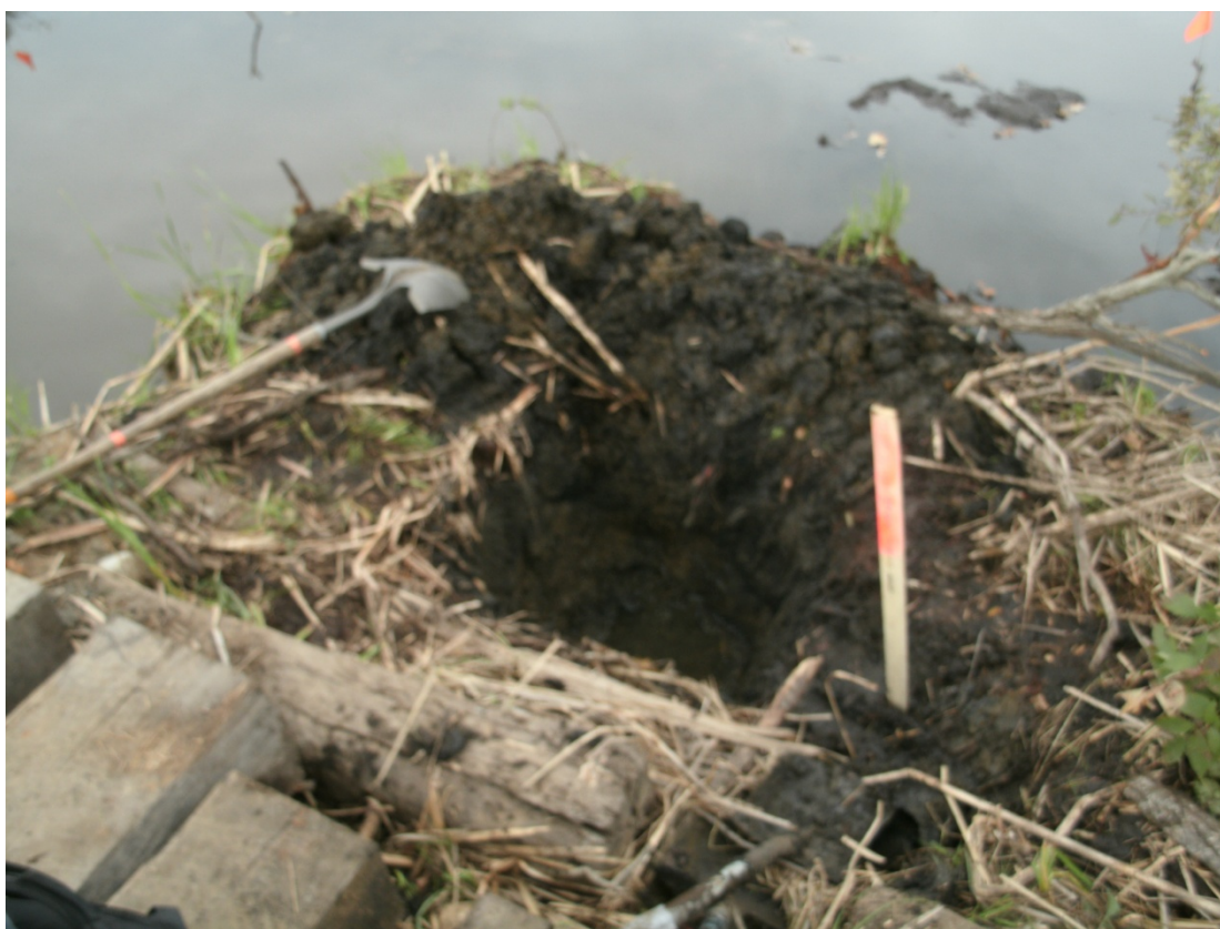
36+50L – 37+00L: Looking toward Talmadge Creek at 6-hour test pit (September 20, 2010)
