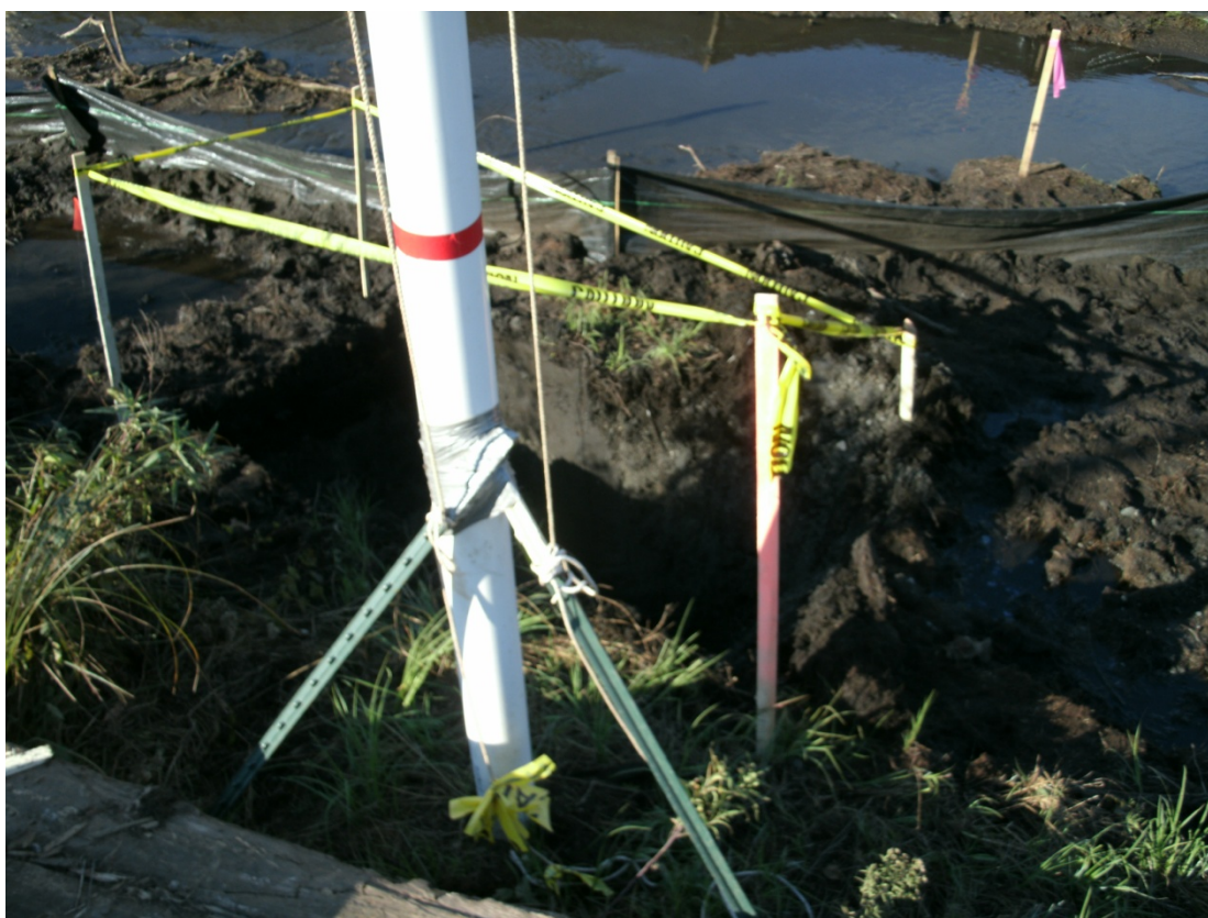
31+50L – 32+00L: Looking toward Talmadge Creek (September 14, 2010)
