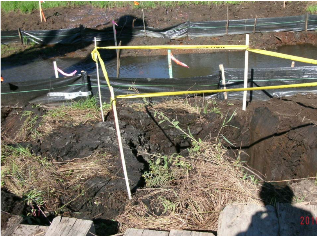
38+50L – 39+00L: Looking toward Talmadge Creek (September 13, 2010)
