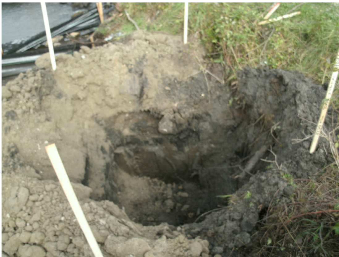
37+50L – 38+00L: Looking toward Talmadge Creek at 6-hour test pit (September 20, 2010)
