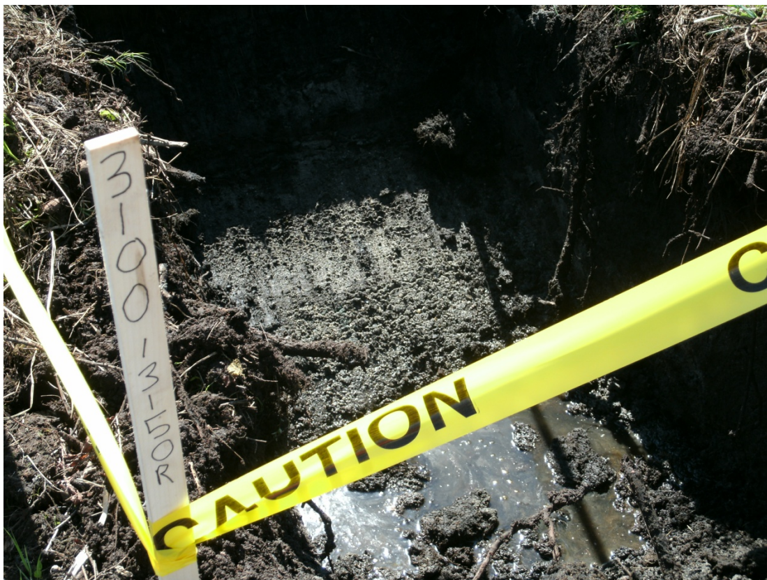
31+00R – 31+50R: Looking at 6-hour test pit (September 13, 2010)
