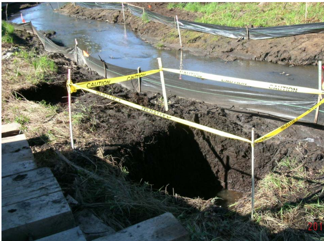
39+00L – 39+50L: Looking downstream (September 15, 2010)
