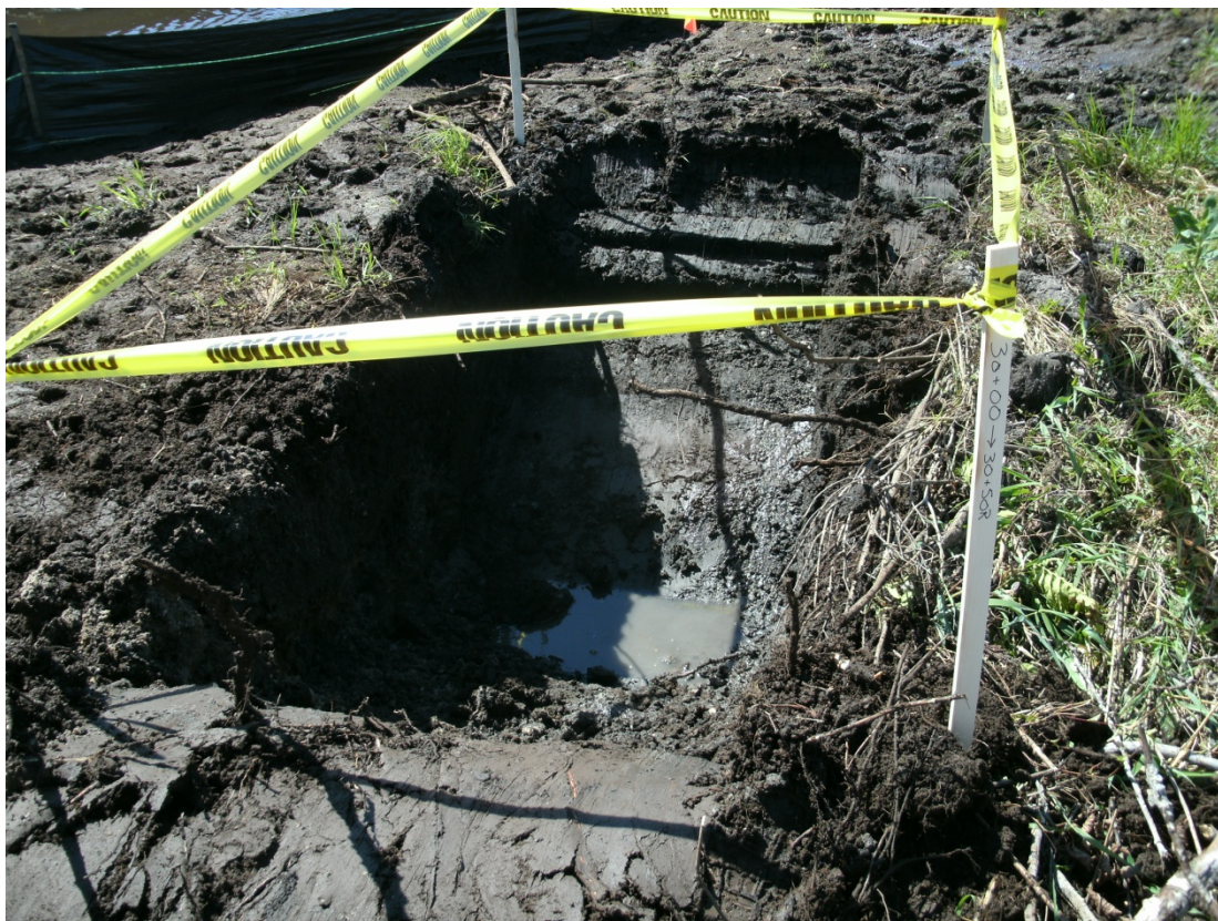
30+00R – 30+50R: Looking at 6-hour test pit (September 14, 2010)
