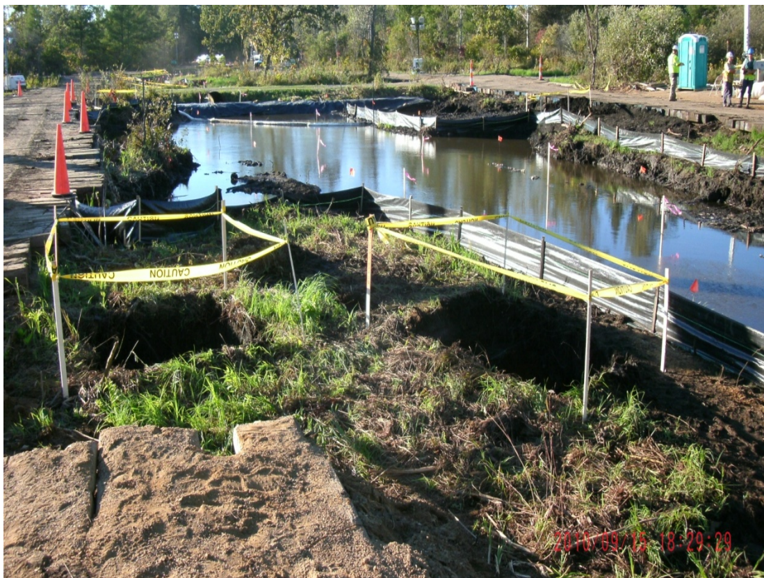
36+00L – 36+50L: Looking downstream (September 15, 2010)
