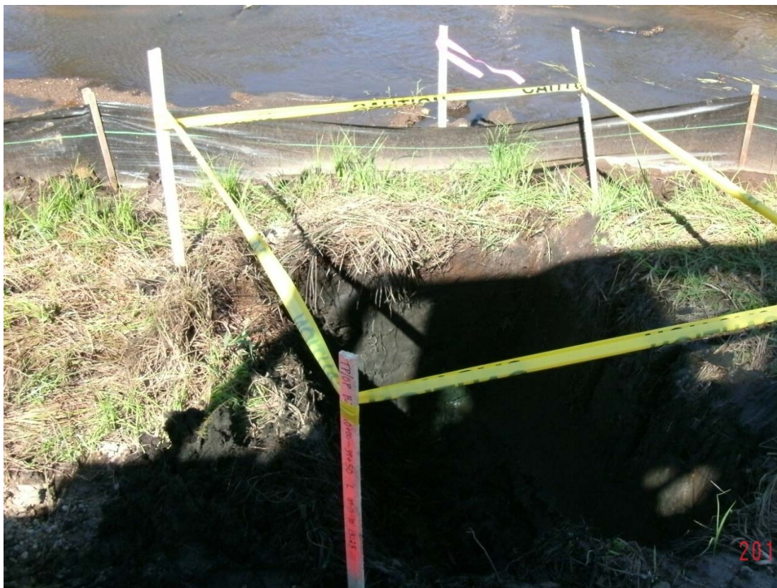
39+50L – 40+00L: Looking toward Talmadge Creek (September 13, 2010)
