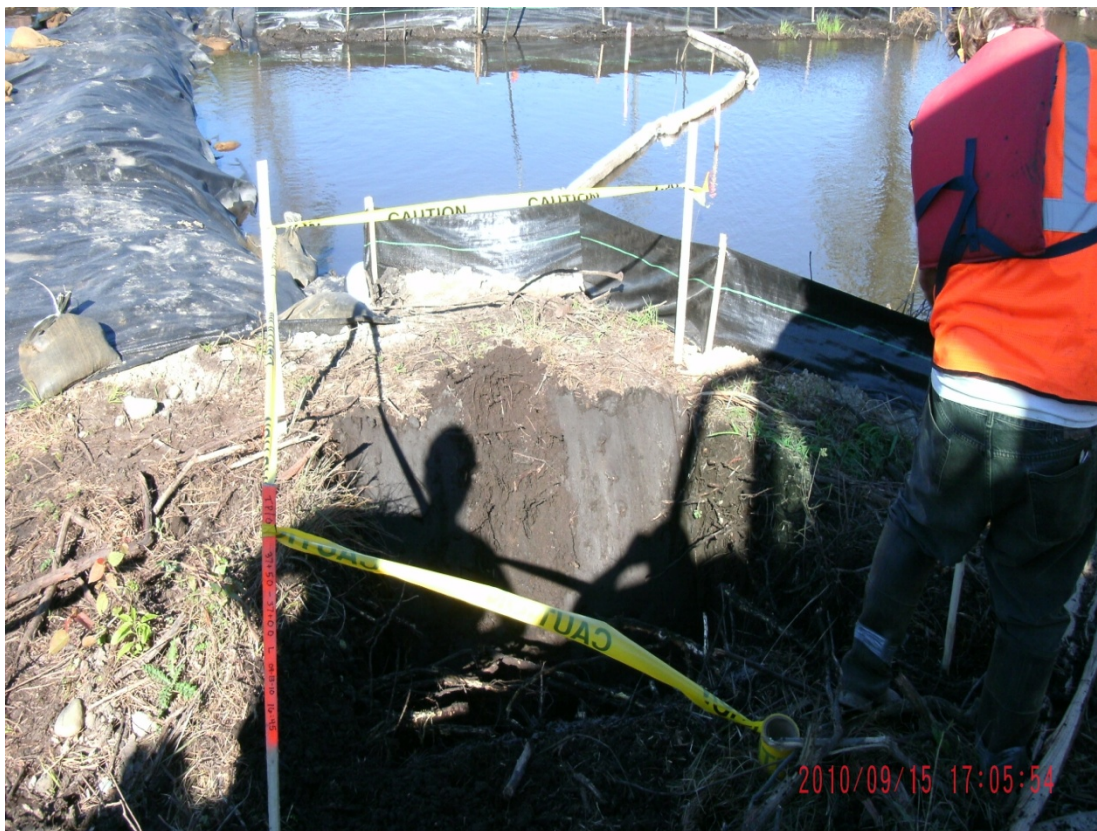
37+00L – 37+50L: Looking toward Talmadge Creek (September 15, 2010)
