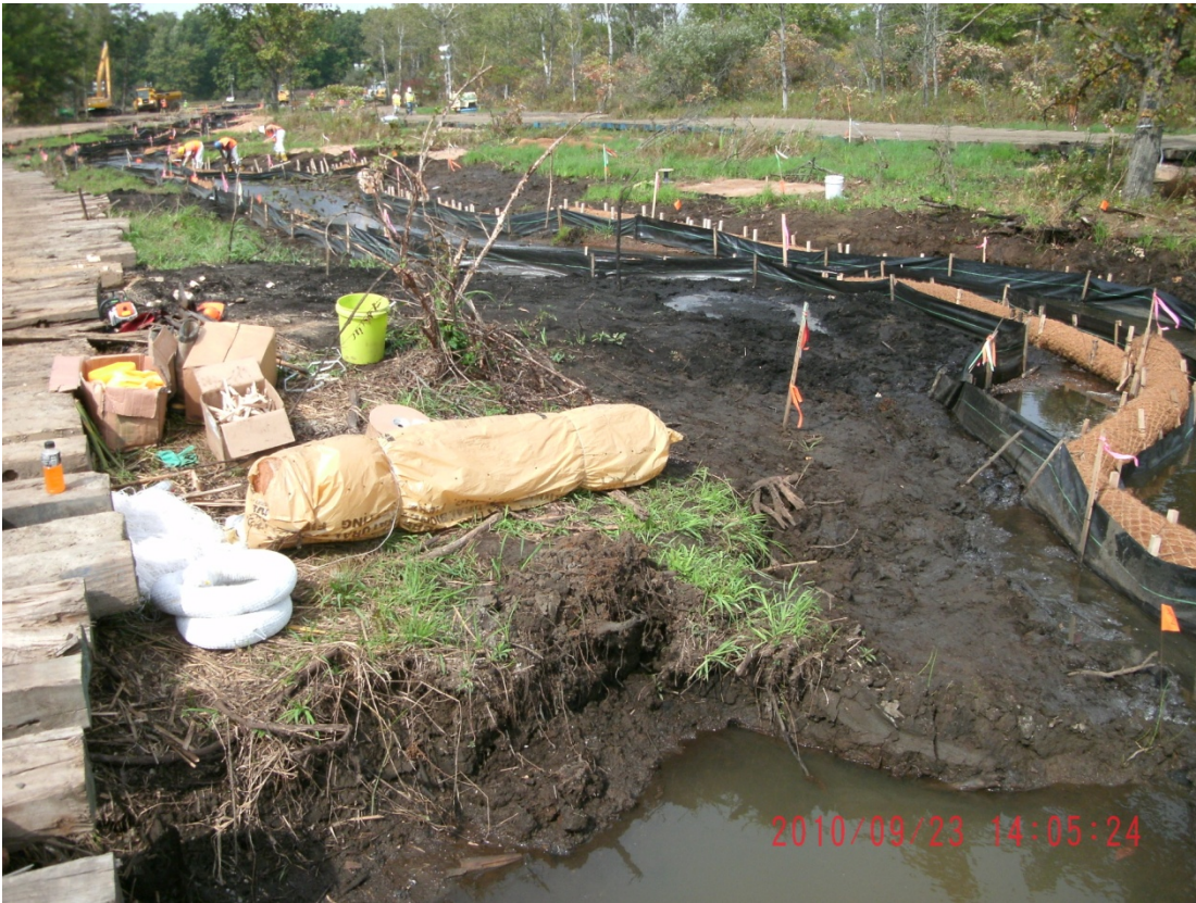
38+00L – 38+50L: Looking downstream (September 23, 2010)
