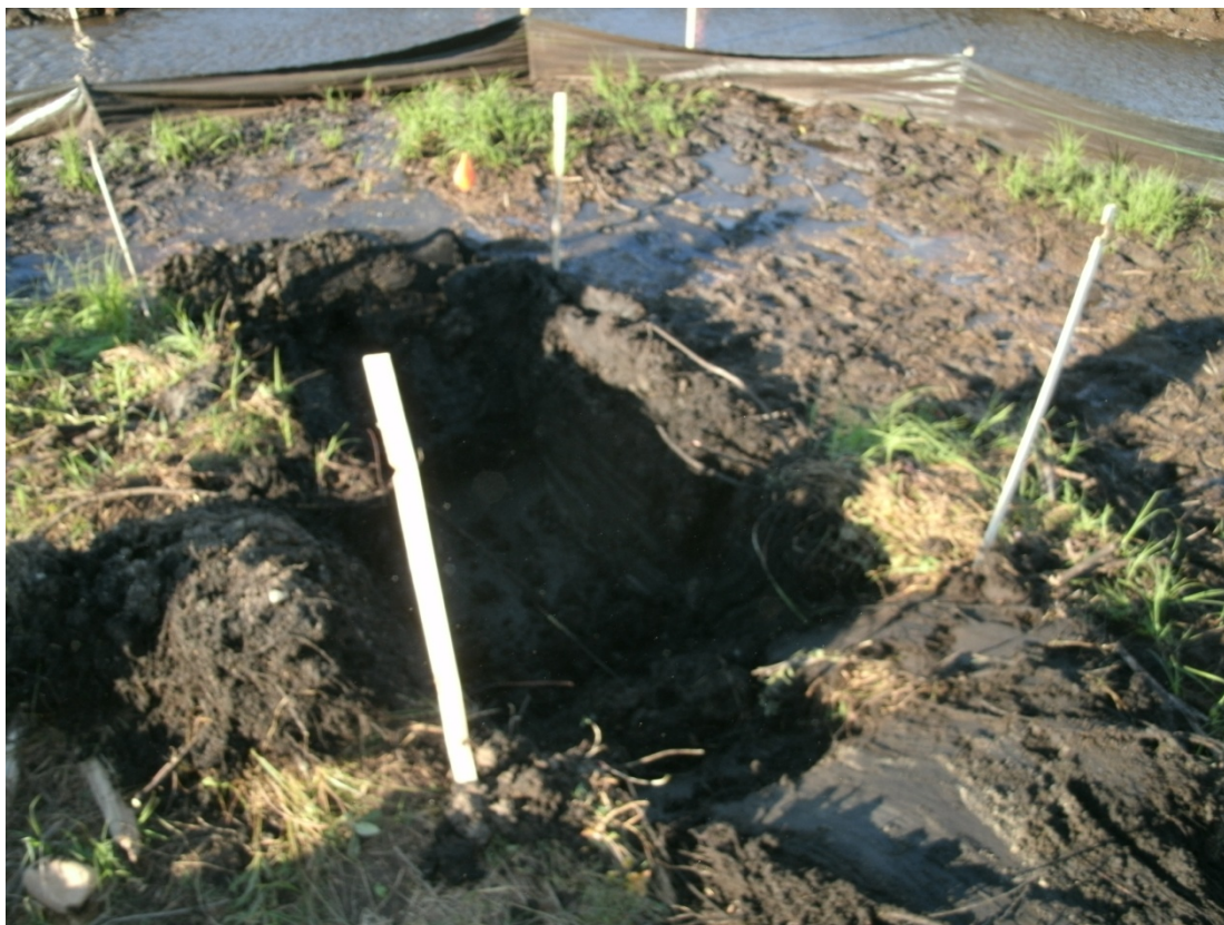
31+00L – 31+50L: Looking toward Talmadge Creek (September 14, 2010)
