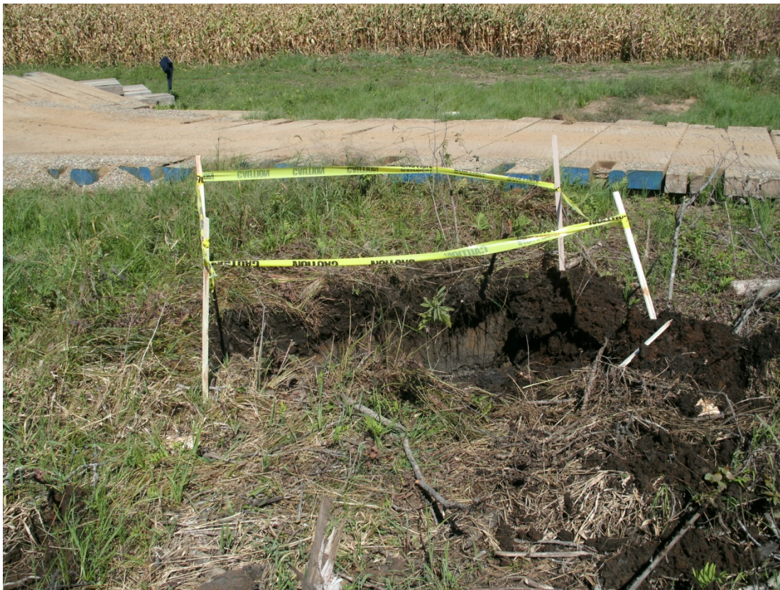
30+00L – 30+50L: Looking away from Talmadge Creek (September 14, 2010)
