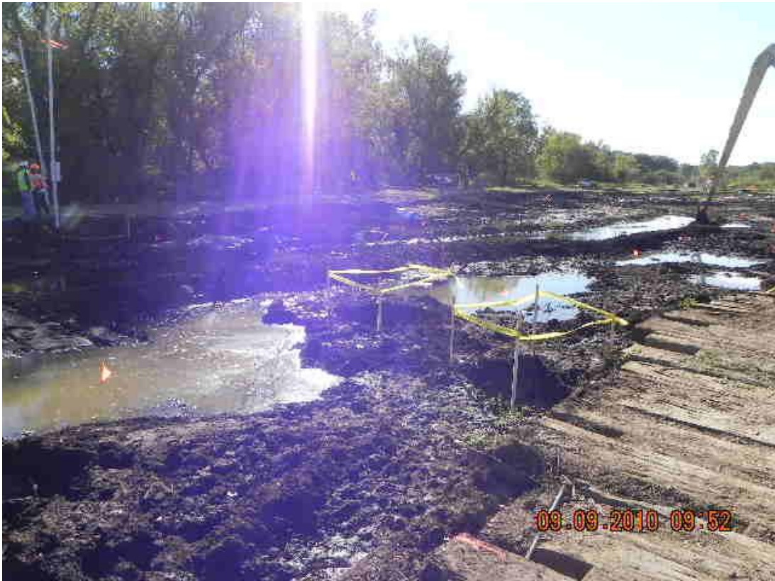
22+00L – 22+50L: Looking upstream (September 9, 2010)
