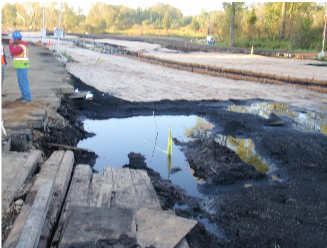
23+25R – 23+75R: Looking upstream at 48-hour observation pit (September 15, 2010)
