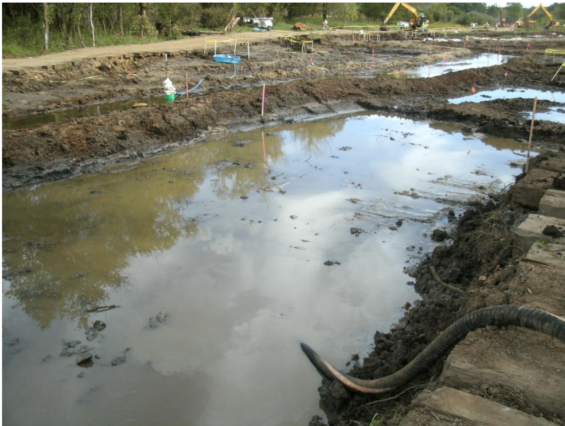
22+50L – 23+00L: Looking upstream at area cleared for backfill (September 9, 2010)
