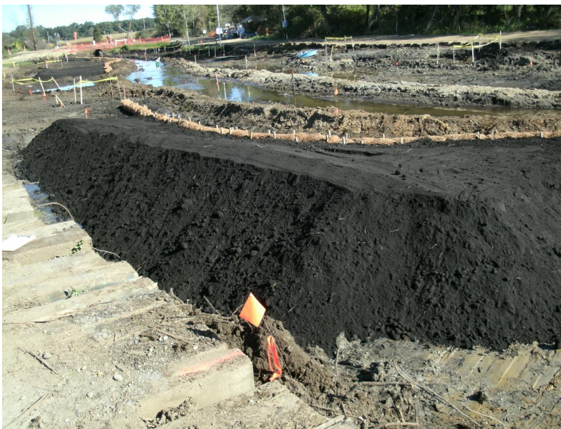
20+50L – 21+00L: Looking downstream (September 10, 2010)
