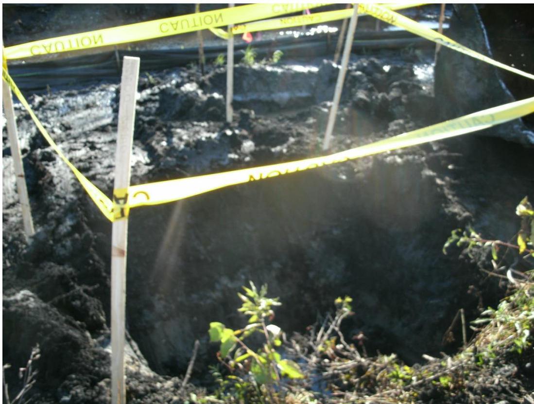
26+00L – 26+50L: Looking toward Talmadge Creek at 6-hour test pit (September 13, 2010)
