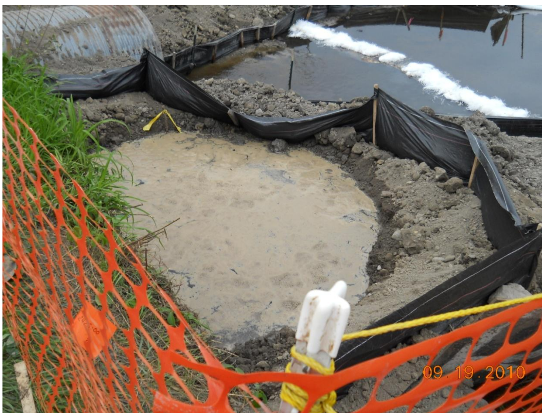
23+75R – 24+50R: Looking toward Talmadge Creek at 6-hour test pit (September 19, 2010)
