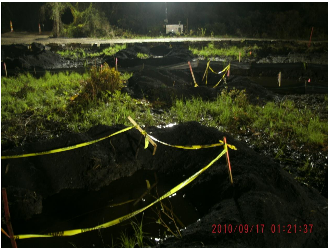
25+00R – 25+50R: Looking toward Talmadge Creek at 48-hour observation pit (September 17, 2010)
