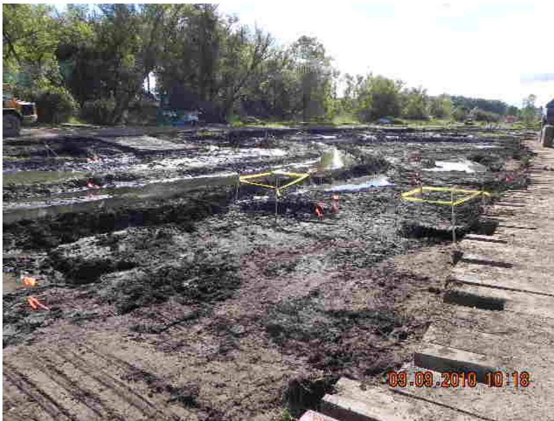
21+00L – 21+50L: Looking upstream (September 9, 2010)
