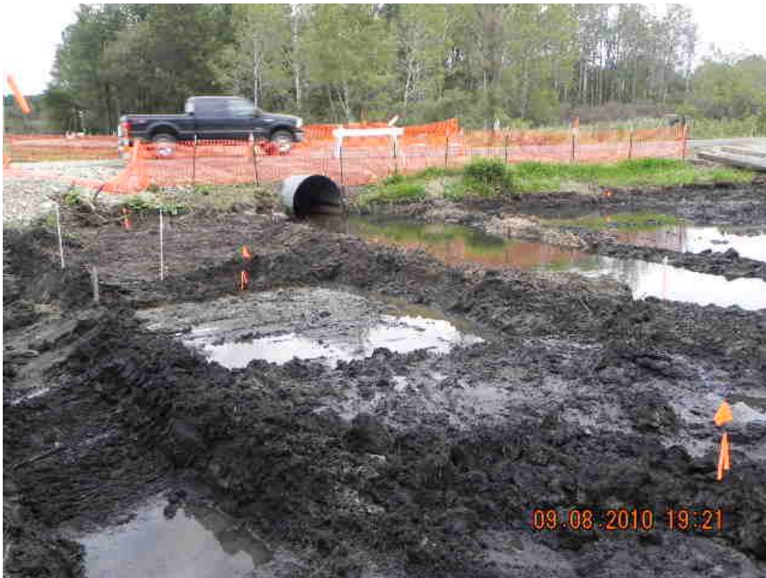
24+00L – 24+50L: Looking downstream at Division Drive over Talmadge Creek (September 8, 2010)
