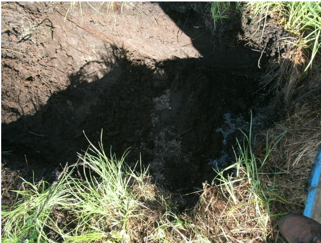
28+50R- 29+00R: Looking at 48-hour observation pit (September 12, 2010)
