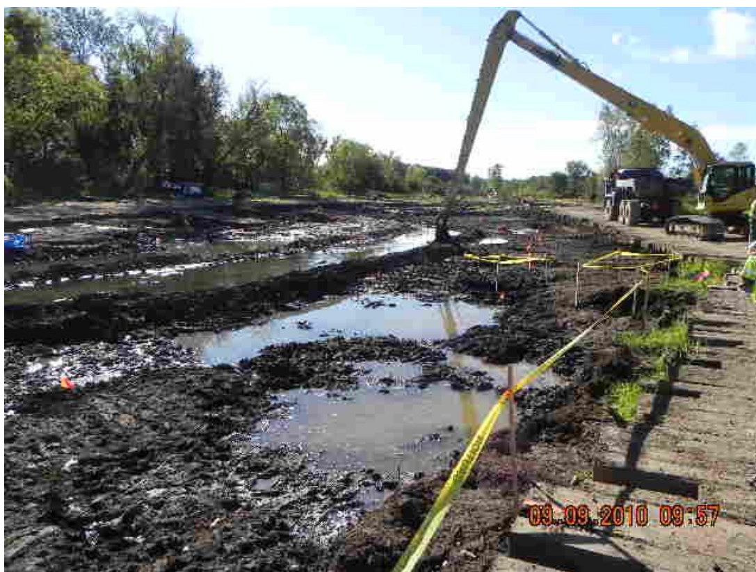
21+50L – 22+00L: Looking upstream (September 9, 2010)
