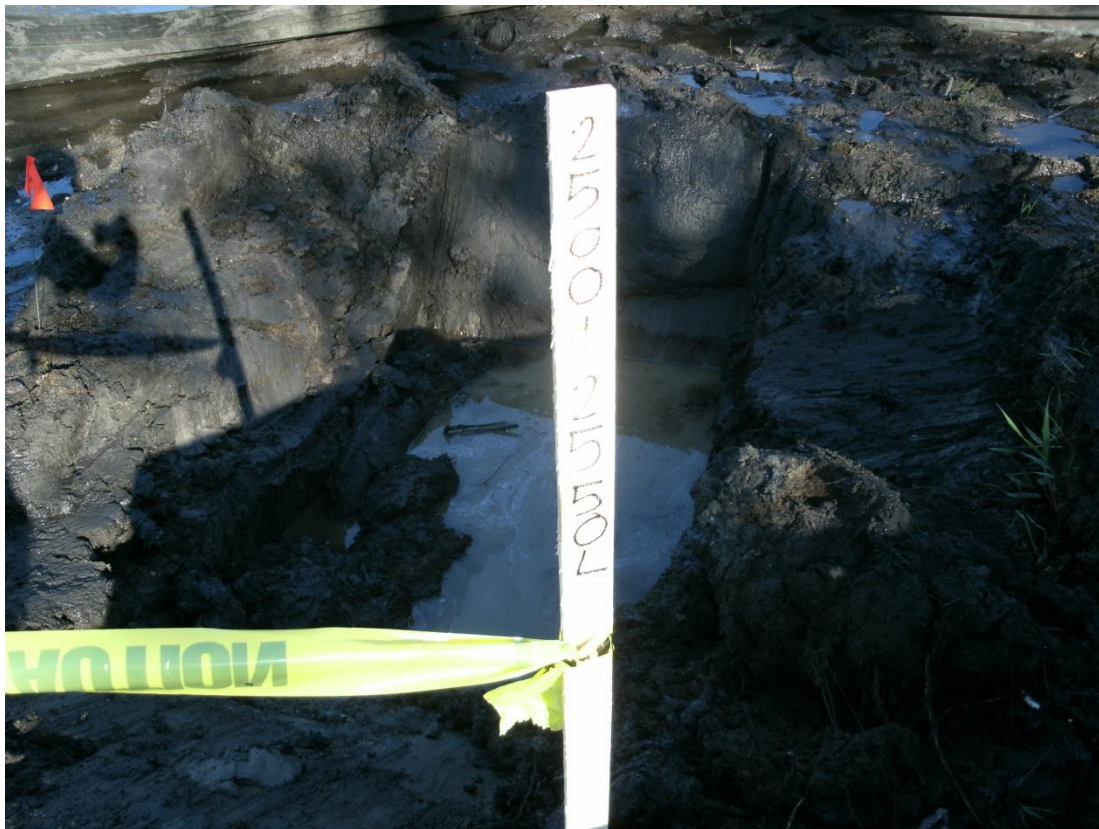
25+00L – 25+50L: Looking at 6-hour test pit (September 12, 2010)
