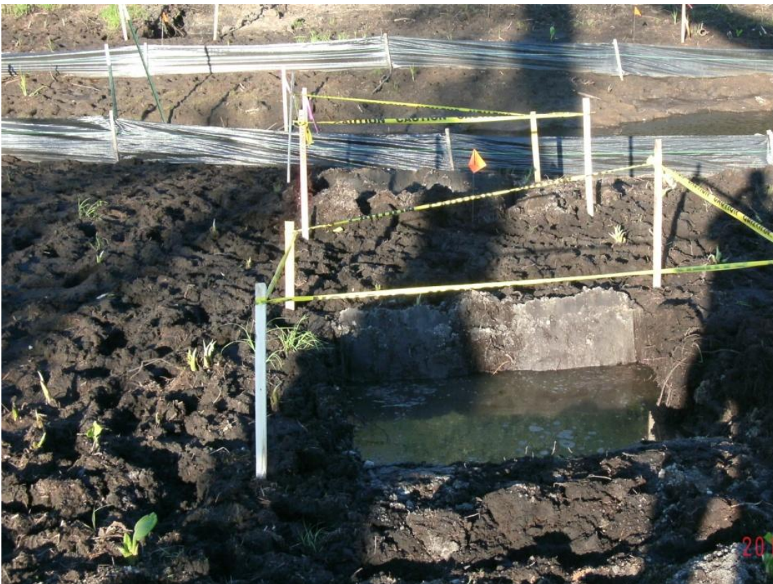
28+50L – 29+00L: Looking toward Talmadge Creek at 6-hour test pit (September 14, 2010)
