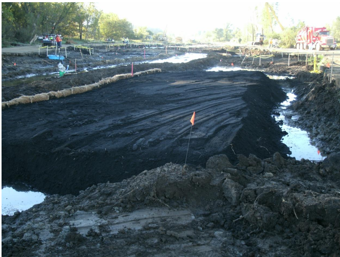
23+00L – 23+50L: Looking upstream at backfill (September 10, 2010)
