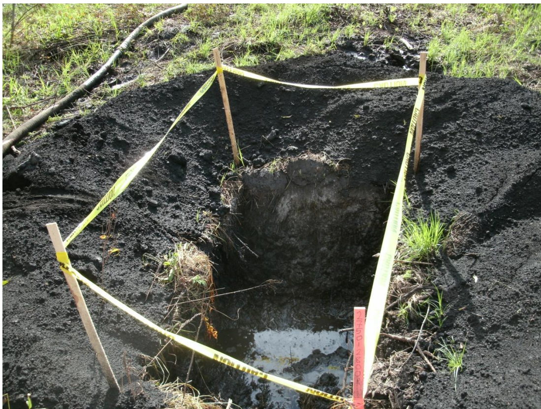
27+50R – 28+00R: Looking at 48-hour observation pit (September 17, 2010)
