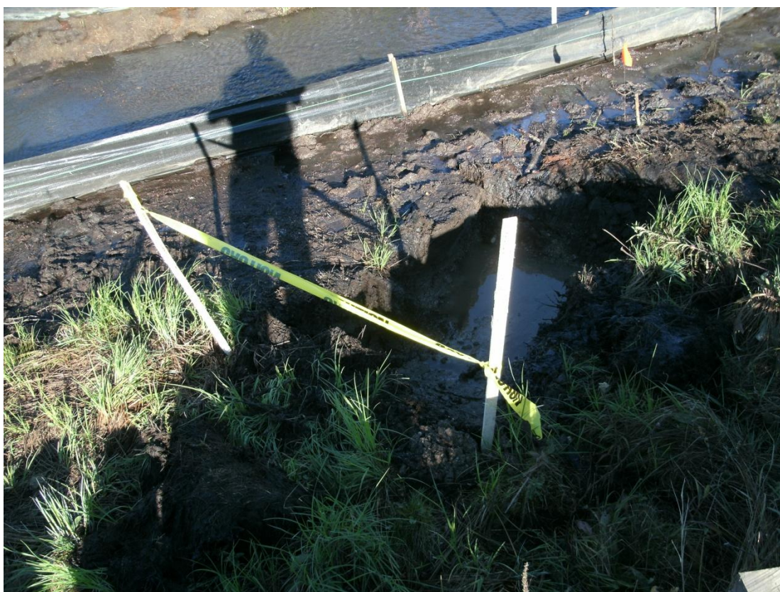
25+50L – 26+00L: Looking toward Talmadge Creek at 6-hour test pit (September 12, 2010)
