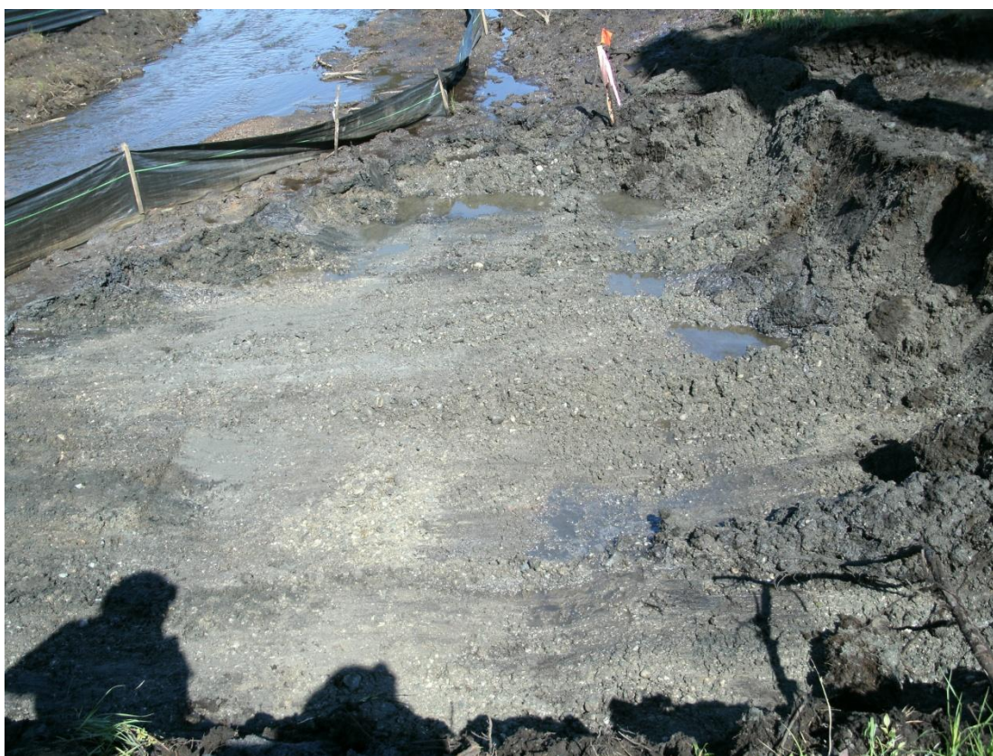
28+00R – 28+50R: Looking toward Talmadge Creek at scraped area (September 12, 2010)
