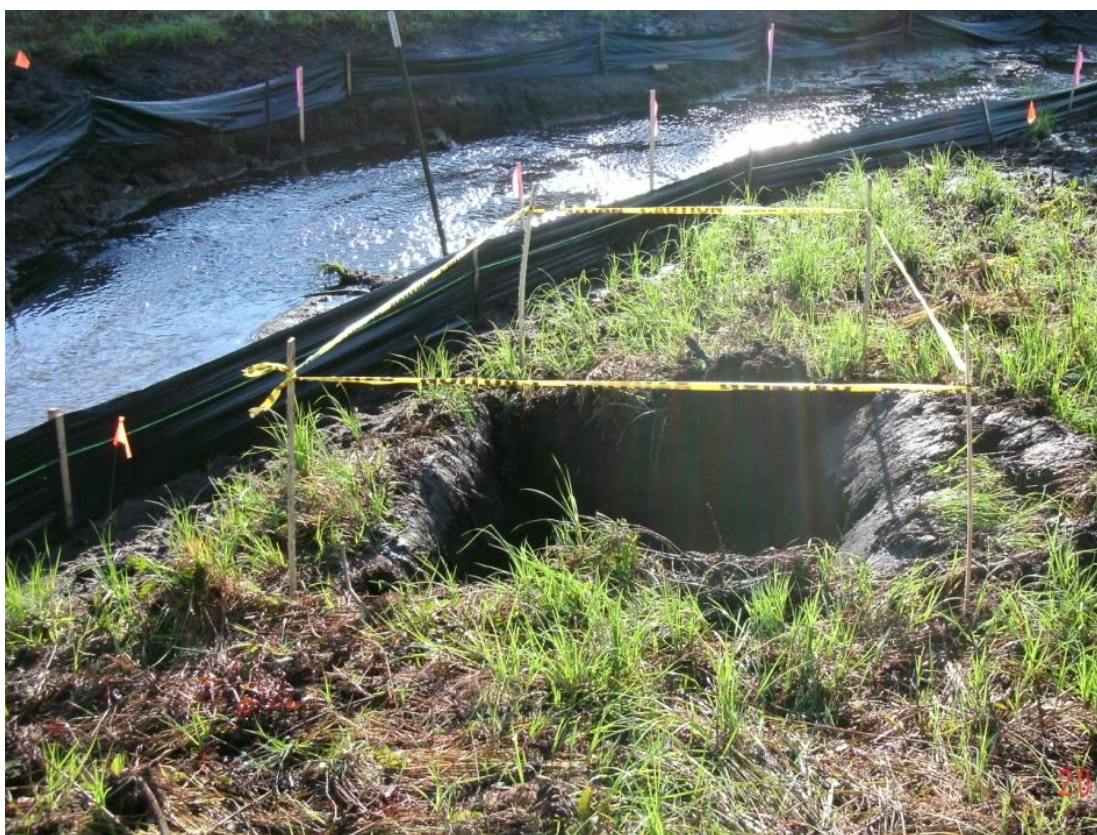
29+50L – 30+00L: Looking toward Talmadge Creek at 6-hour test pit (September 15, 2010)
