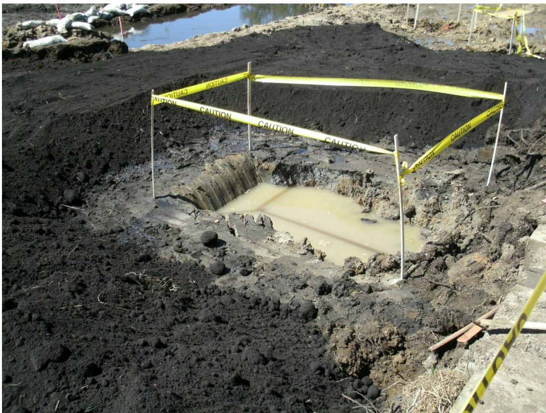
19+25R – 19+75R: Looking downstream at 48-hour observation pit (September 10, 2010)
