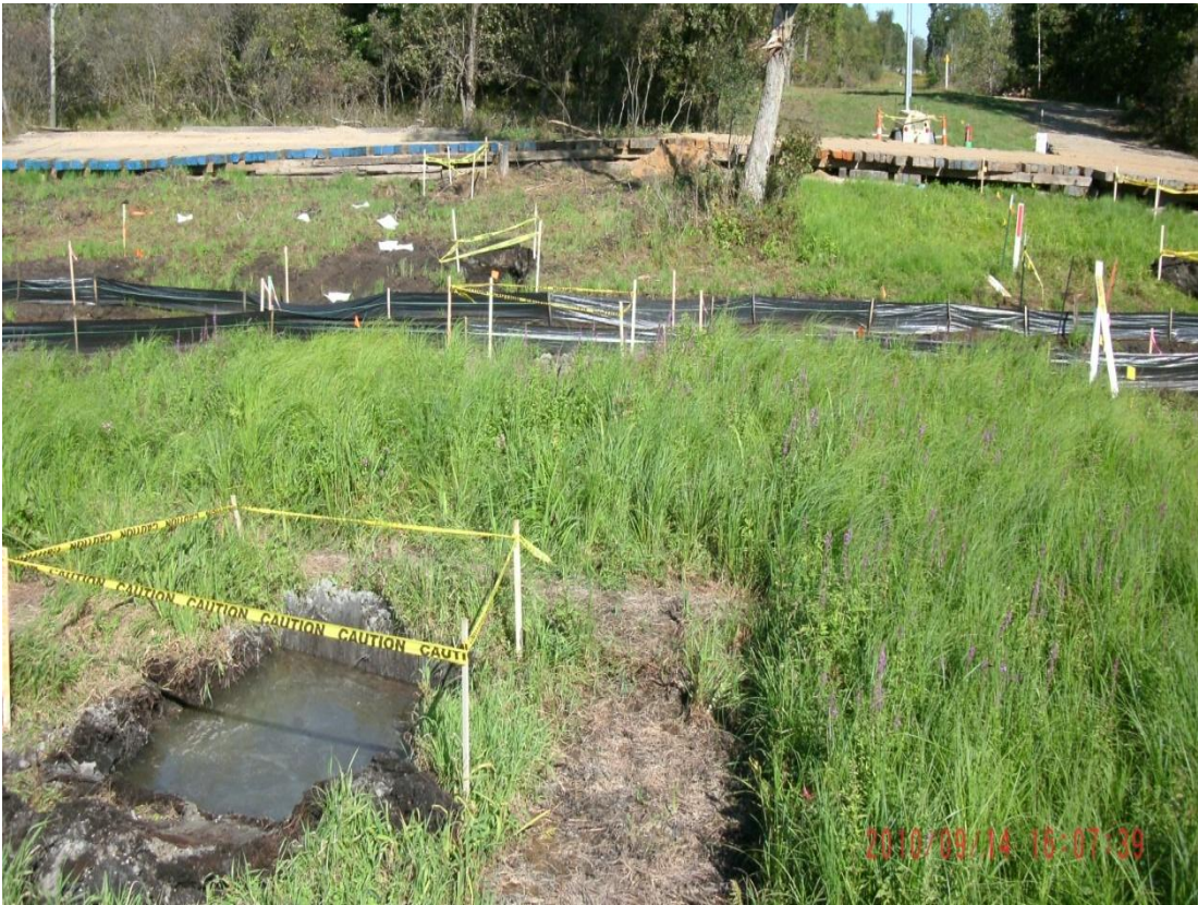
28+00L – 28+50L: Looking toward Talmadge Creek at 6-hour test pit (September 14, 2010)
