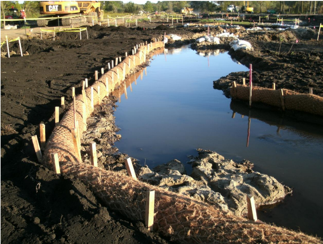
20+25R – 20+75R: Looking upstream (September 10, 2010)
