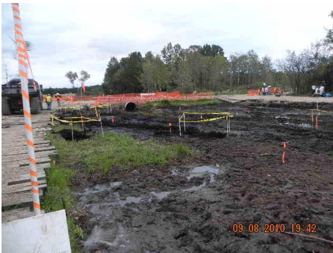
23+50L – 24+00L: Looking downstream (September 8, 2010)
