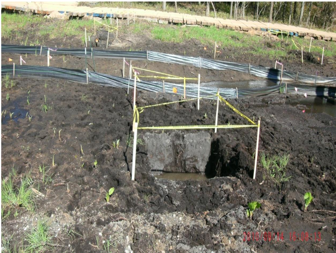
27+00L – 27+50L: Looking toward Talmadge Creek at 6-hour test pit (September 14, 2010)
