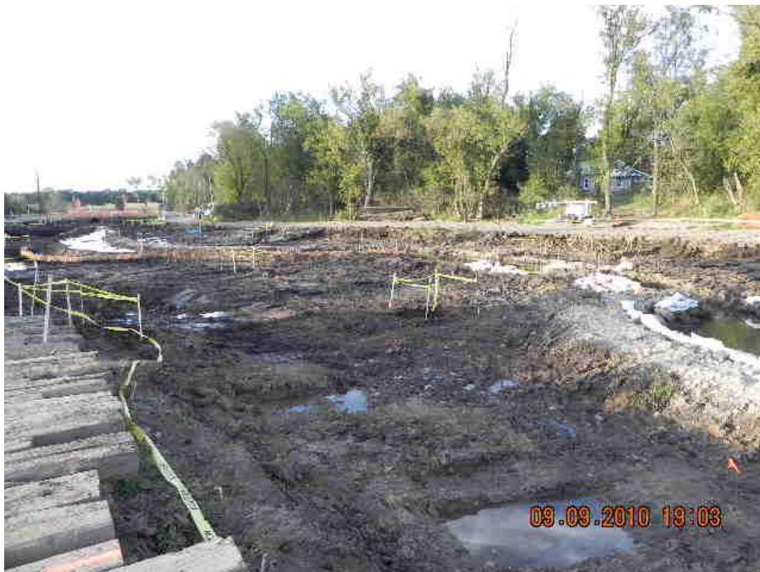
20+00L – 20+50L: Looking downstream (September 9, 2010)
