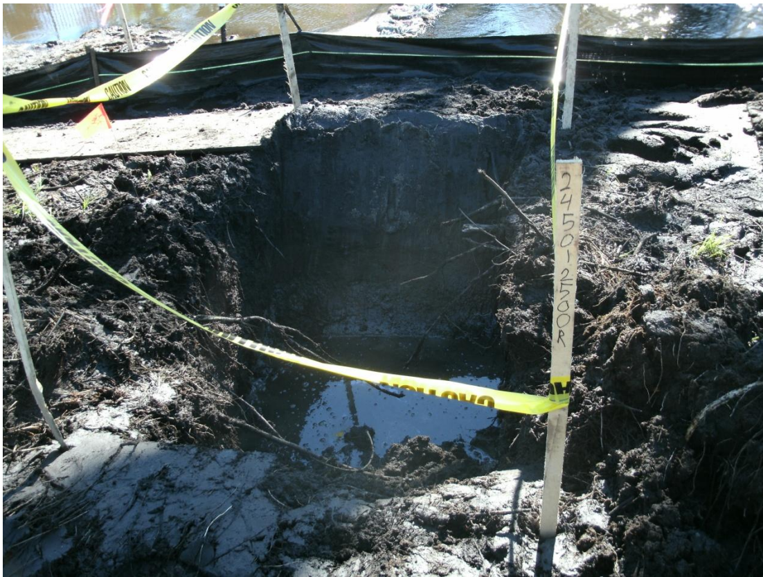
24+50R – 25+00R: Looking toward Talmadge Creek at 6-hour test pit (September 12, 2010)
