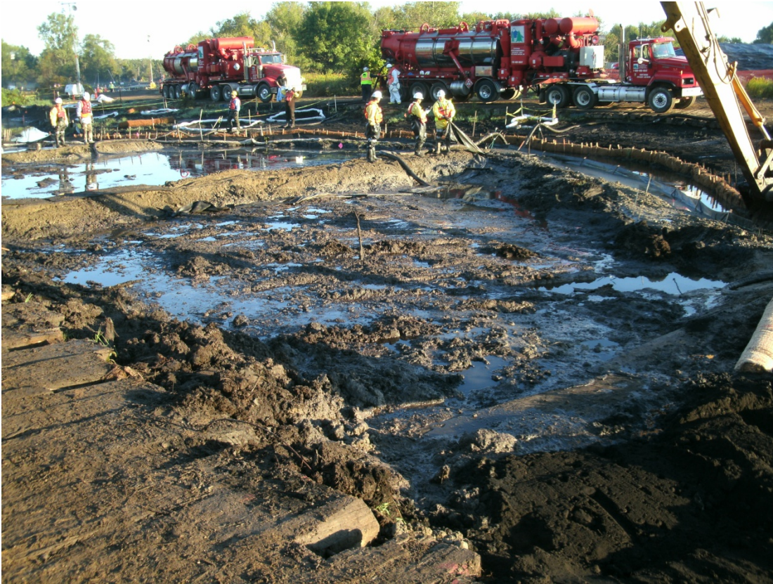
12+00L – 12+50L: Looking toward Talmadge Creek prior to backfill (September 13, 2010)
