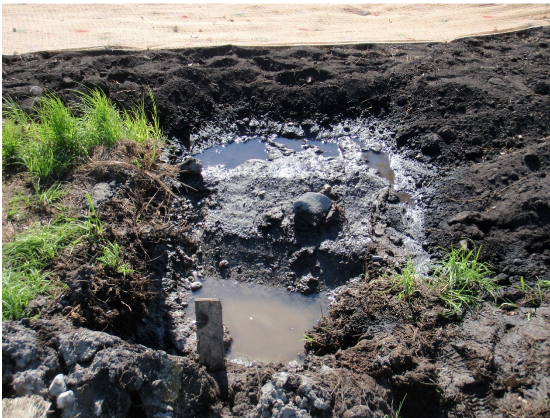
15+75R – 16+25R: Looking at 48-hour observation pit prior to backfill (September 14, 2010)
