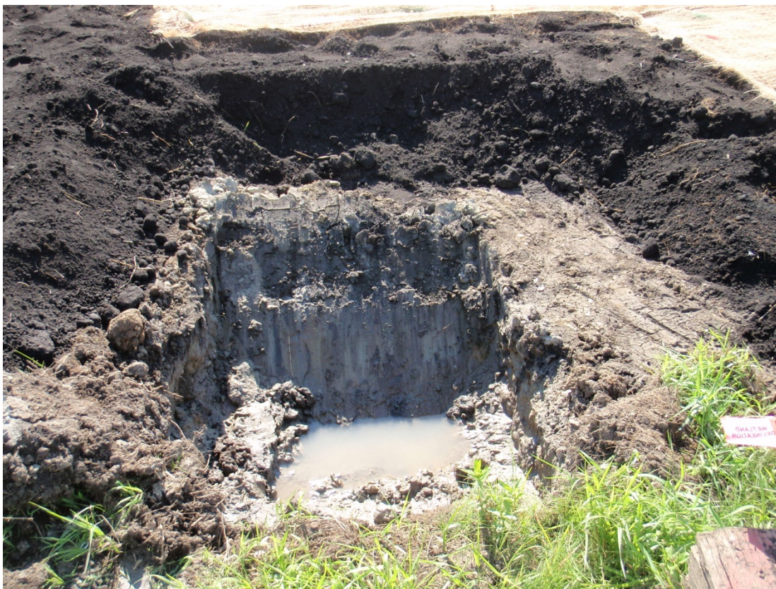
17+75R – 18+25R: Looking at 48-hour observation pit prior to backfill (September 14, 2010)
