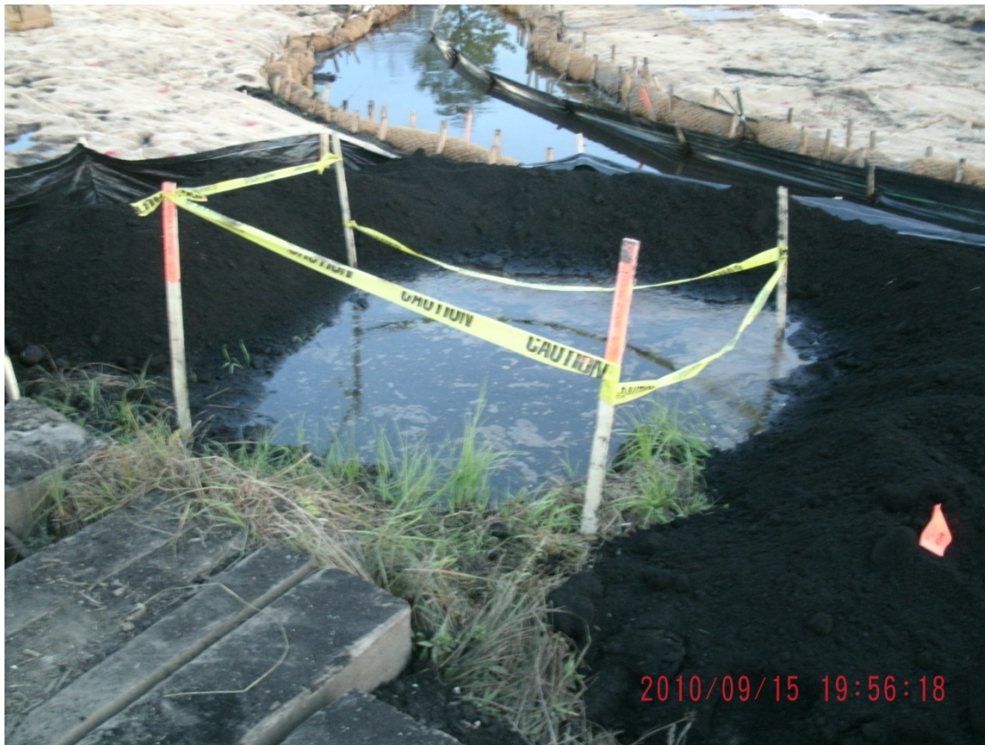
11+50R – 12+00R: Looking at 48-hour observation pit prior to backfill (September 15, 2010)
