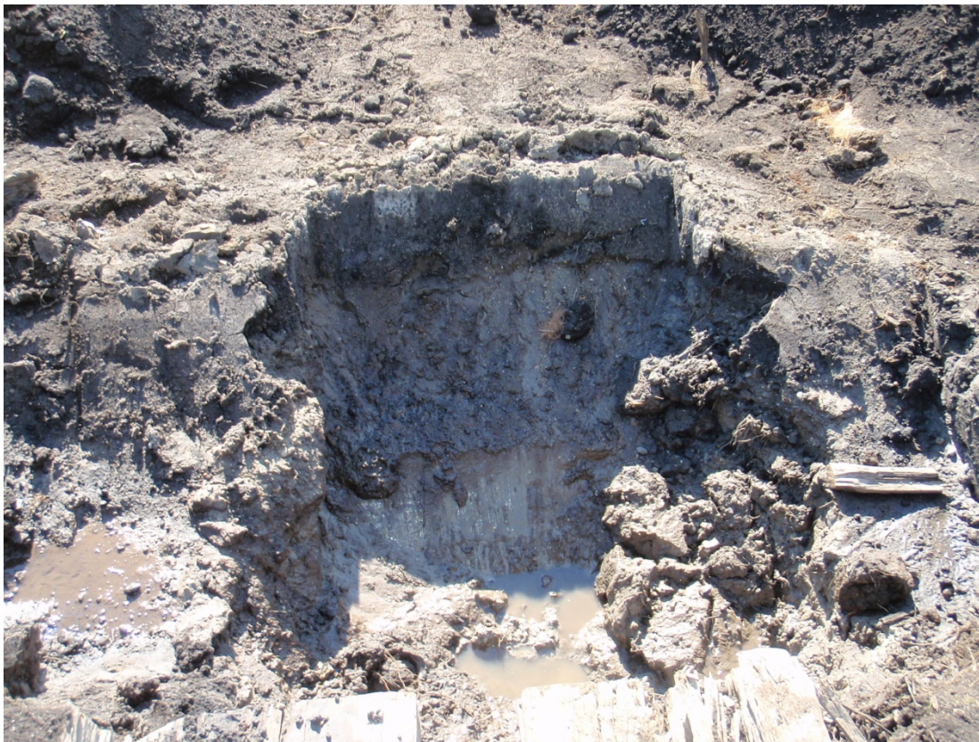
18+25R – 18+75R: Looking at 48-hour observation pit prior to backfill (September 14, 2010)
