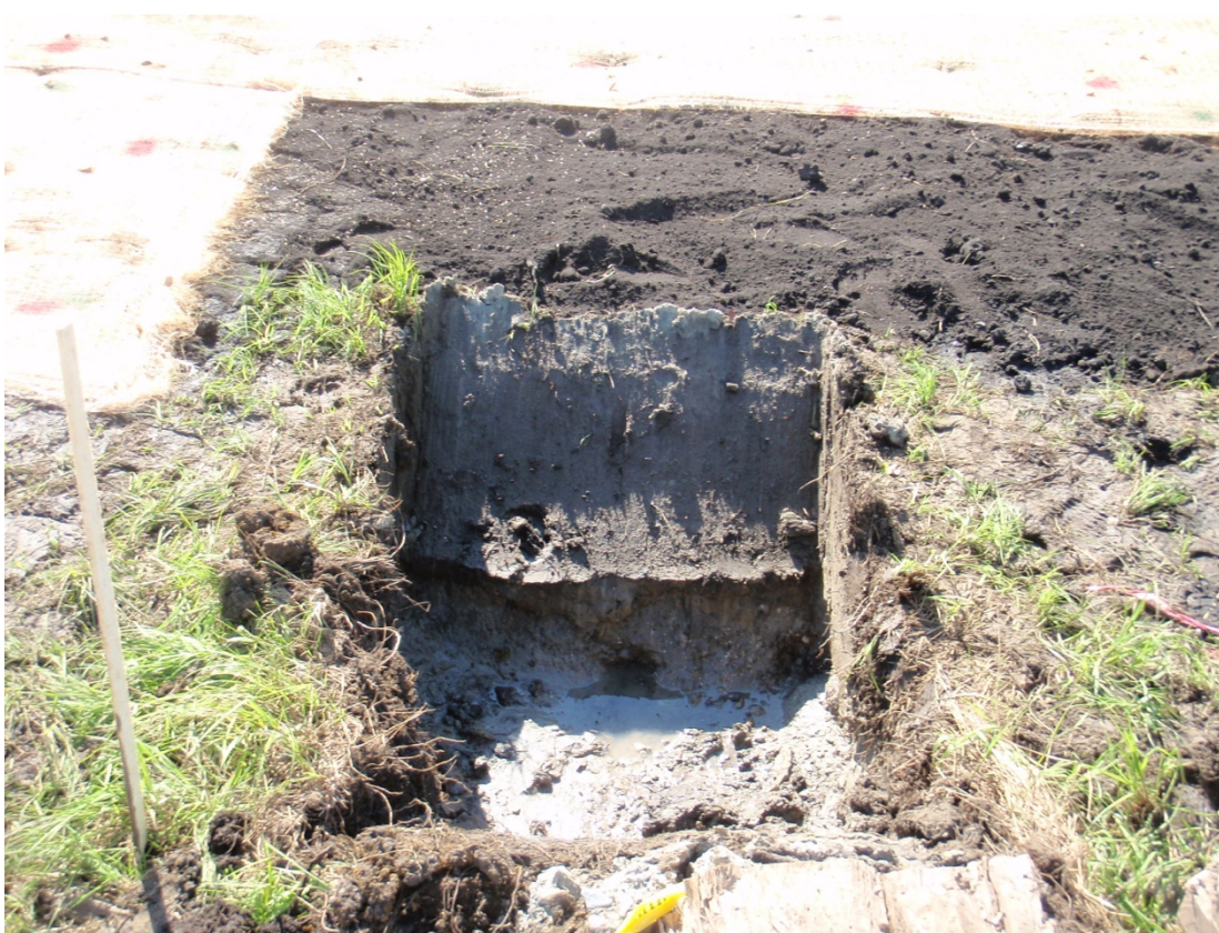
17+25R – 17+75R: Looking at 48-hour observation pit prior to backfill (September 14, 2010)
