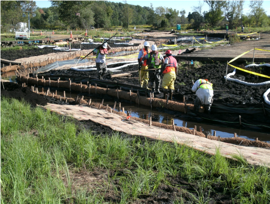
10+00L – 10+50L: Looking toward Talmadge Creek at coir log installation (September 14, 2010)
