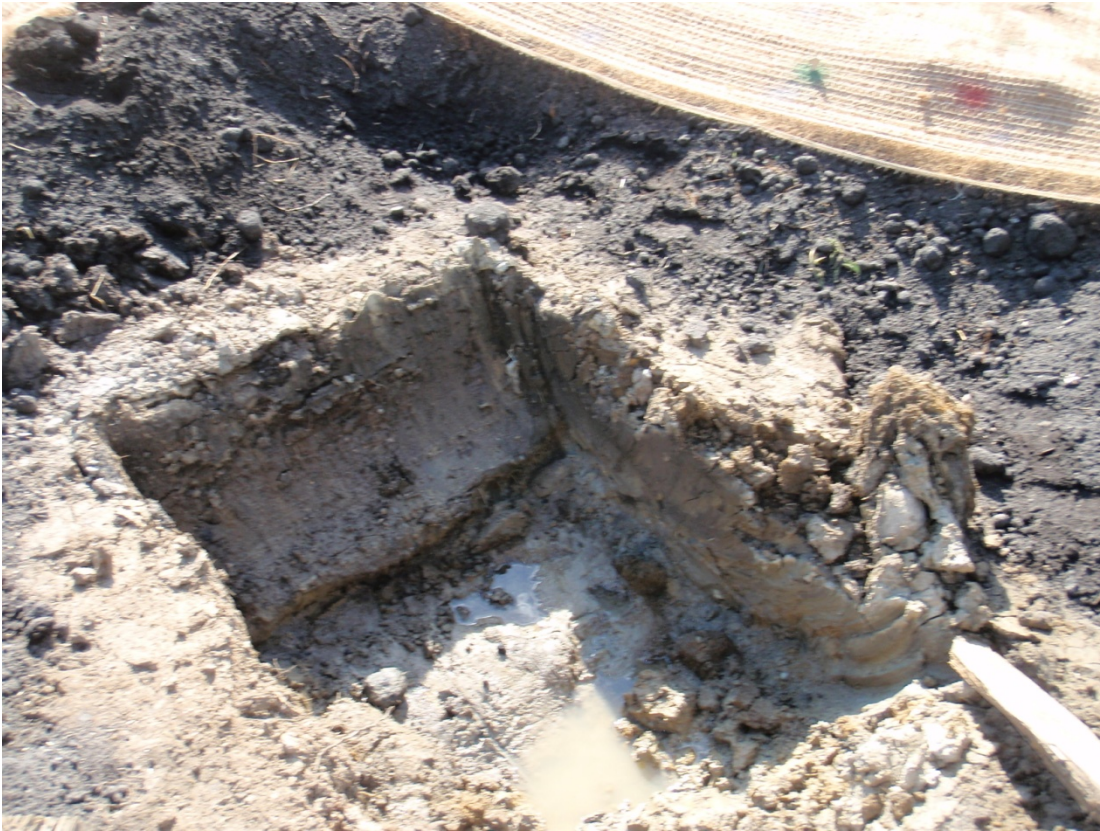
18+75R – 19+25R: Looking at 48-hour observation pit prior to backfill (September 14, 2010)
