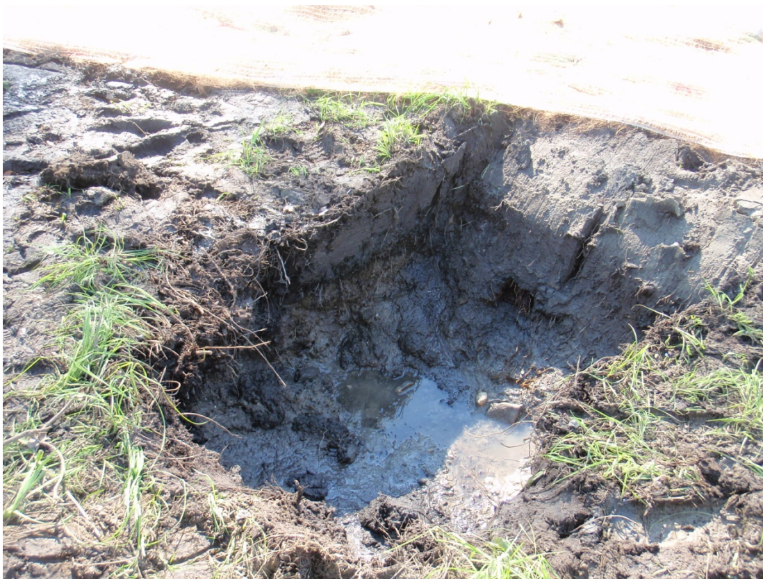
16+75R – 17+25R: Looking at 48-hour observation pit prior to backfill (September 14, 2010)
