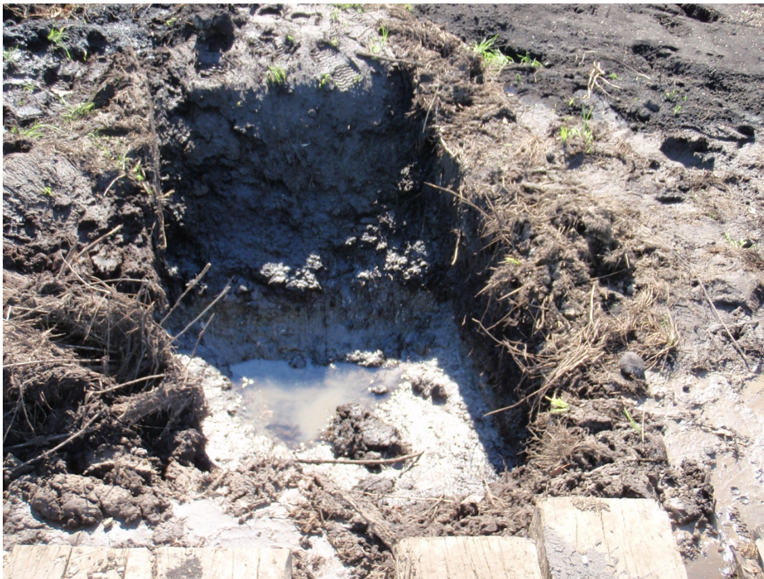
16+25R – 16+75R: Looking at 48-hour observation pit prior to backfill (September 14, 2010)
