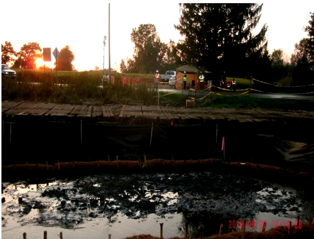
101+50L – 102+00L: Looking toward Talmadge Creek (September 22, 2010)
