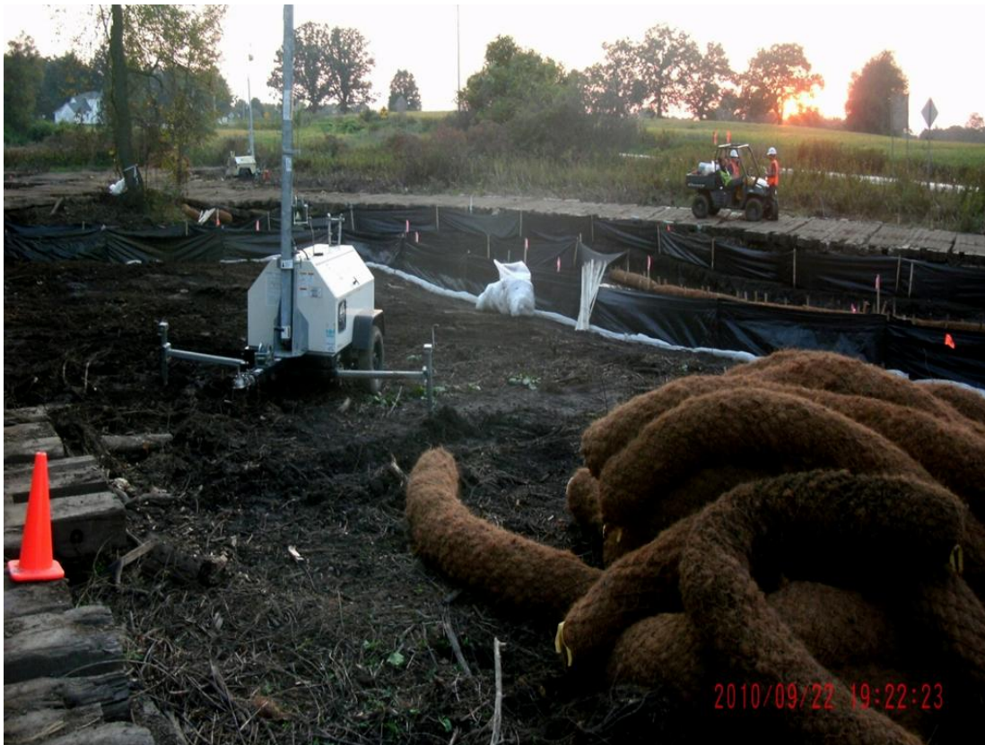
99+00R – 99+50R: Looking upstream (September 22, 2010)
