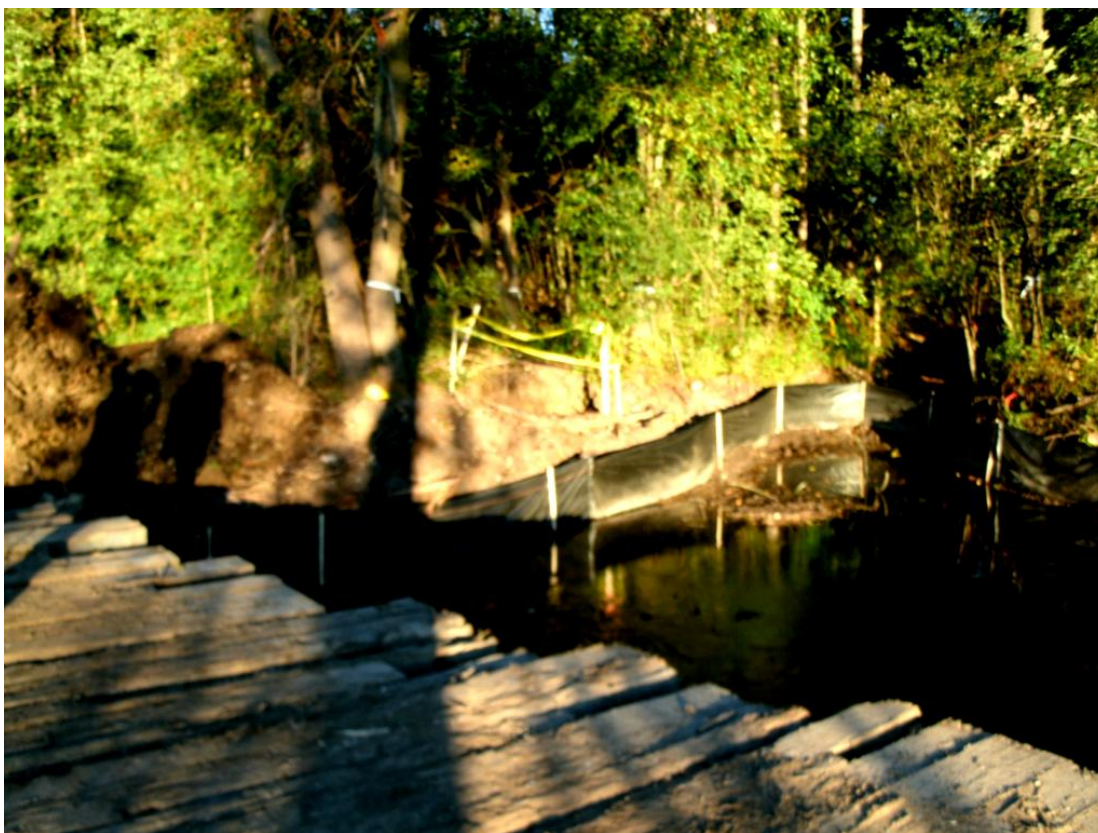
98+50R - 99+00R: Looking upstream from across Talmadge Creek (September 14, 2010)
