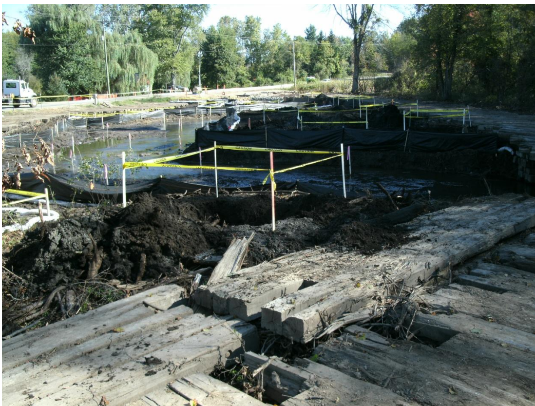
99+50L – 100+00L: Looking downstream (September 14, 2010)
