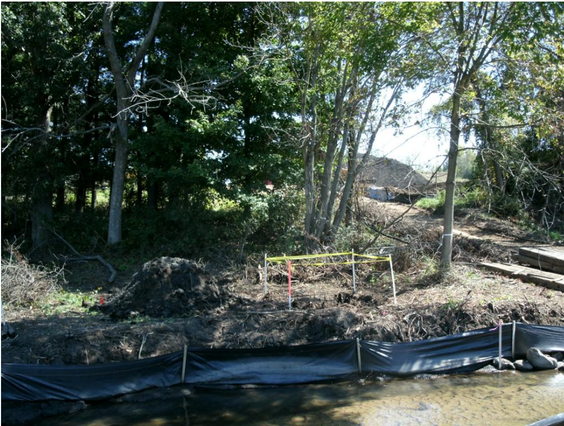
92+00R – 92+50R: Looking across Talmadge Creek (September 14, 2010)
