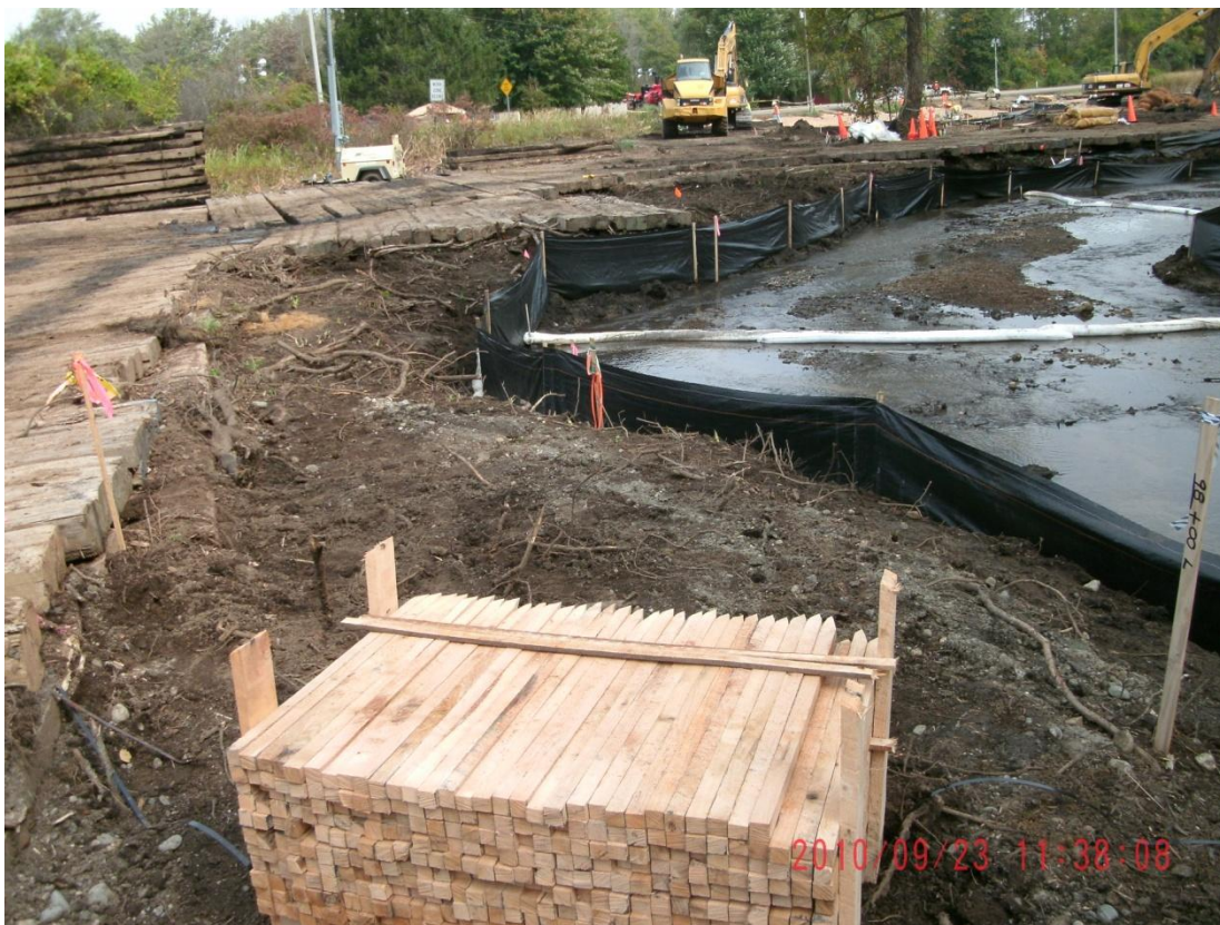
98+00L – 98+50L: Looking downstream (September 23, 2010)
