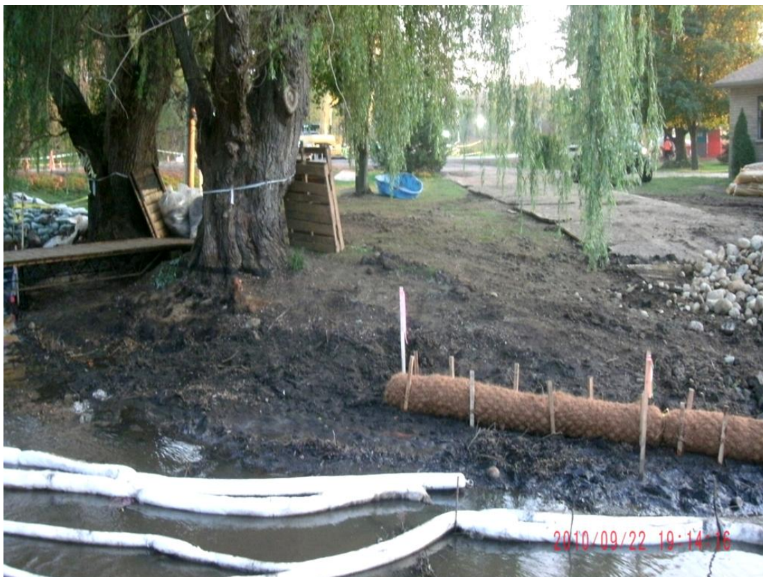
104+00L – 104+50L: Looking across Talmadge Creek (September 22, 2010)
