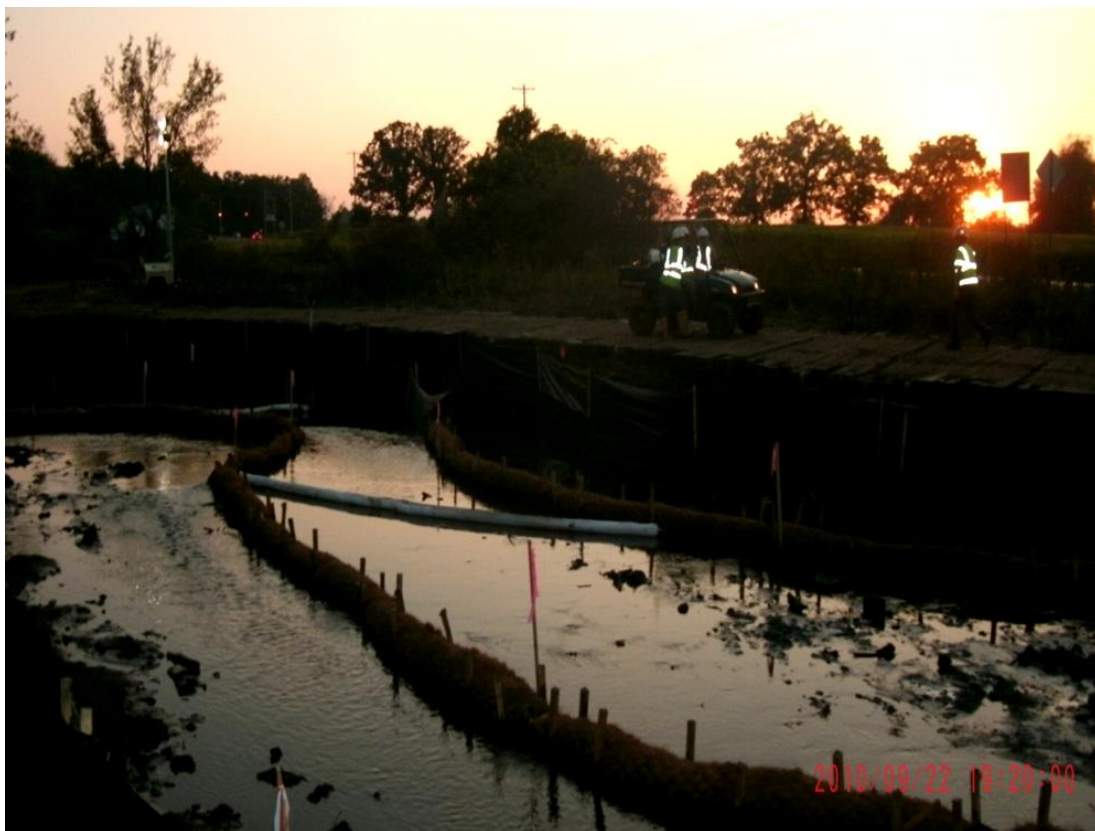
101+00L – 101+50L: Looking downstream (September 22, 2010)
