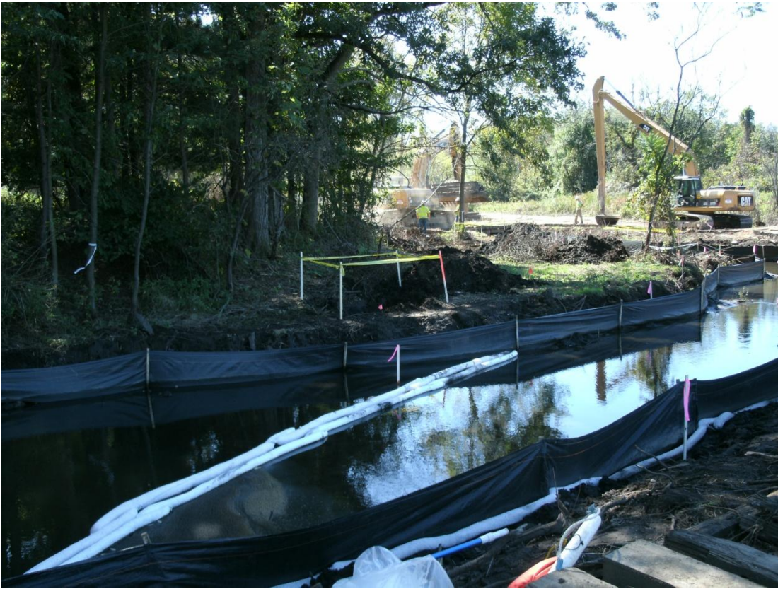
93+00R – 93+50R: Looking upstream across Talmadge Creek (September 14, 2010)
