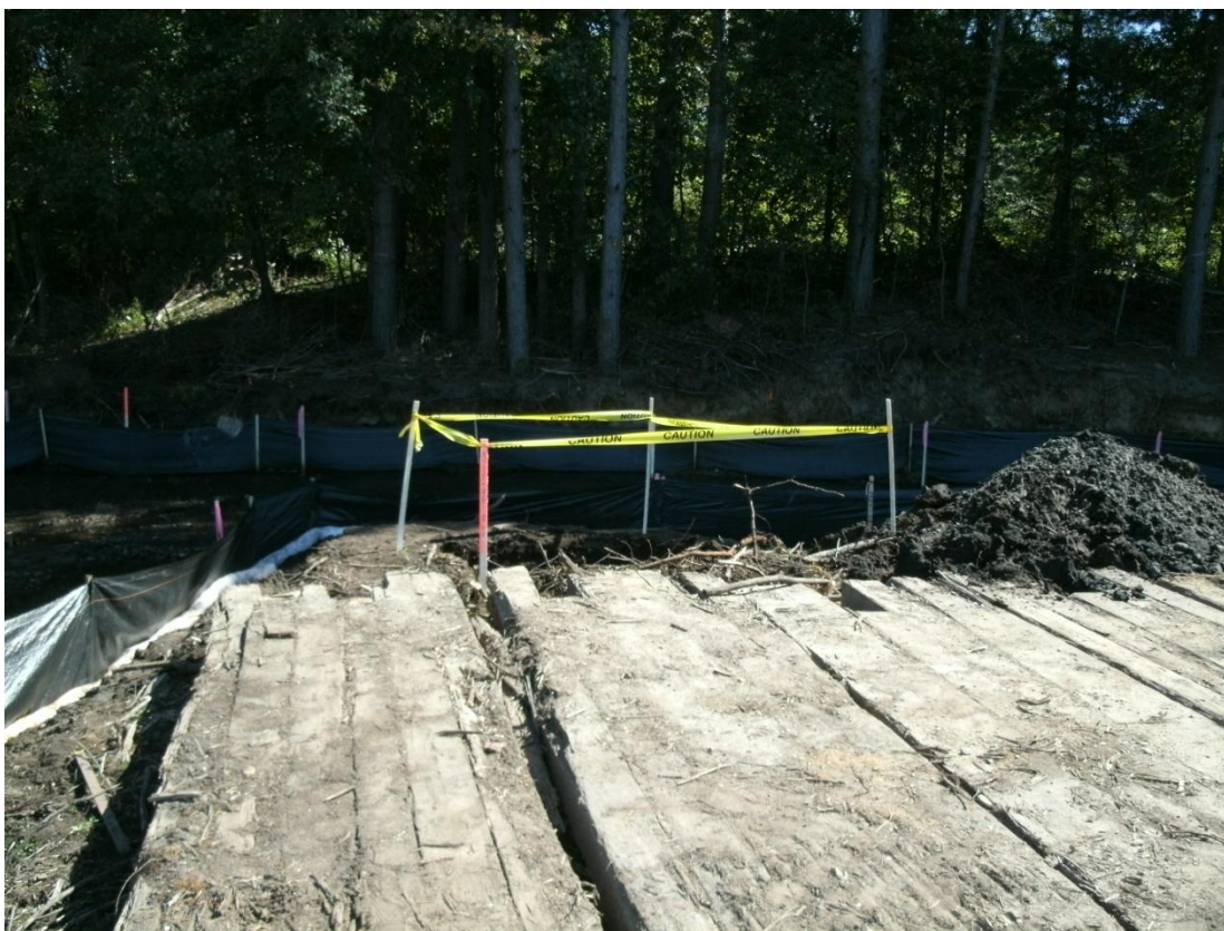
97+50L – 98+00L: Looking toward Talmadge Creek (September 14, 2010)
