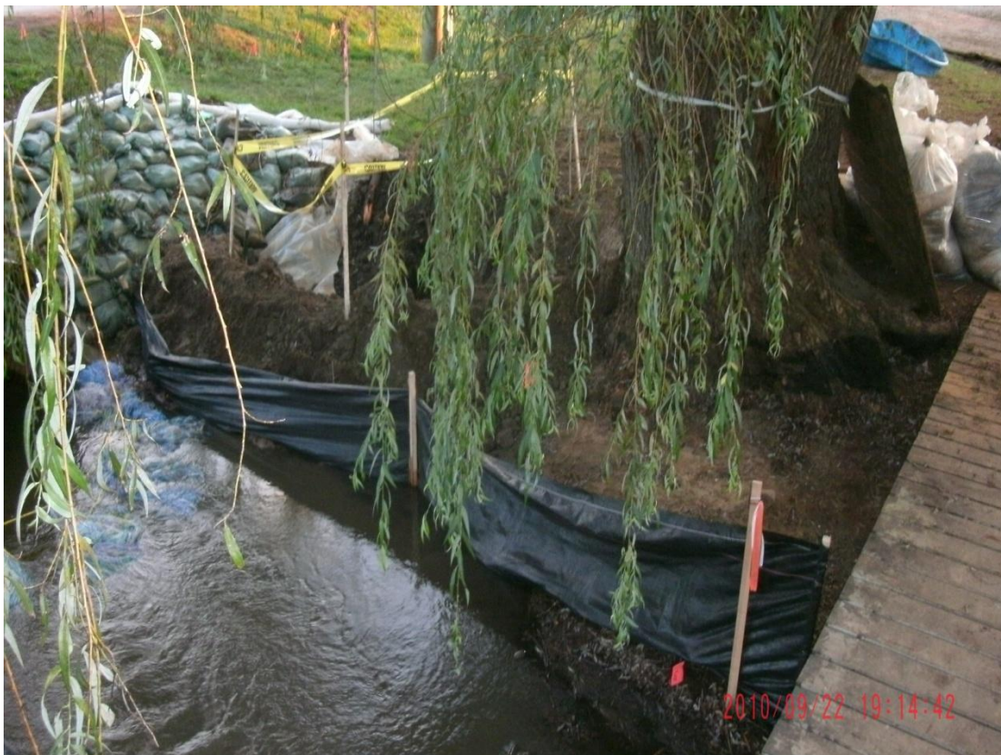
103+50L – 104+00L: Looking across Talmadge Creek (September 22, 2010)
