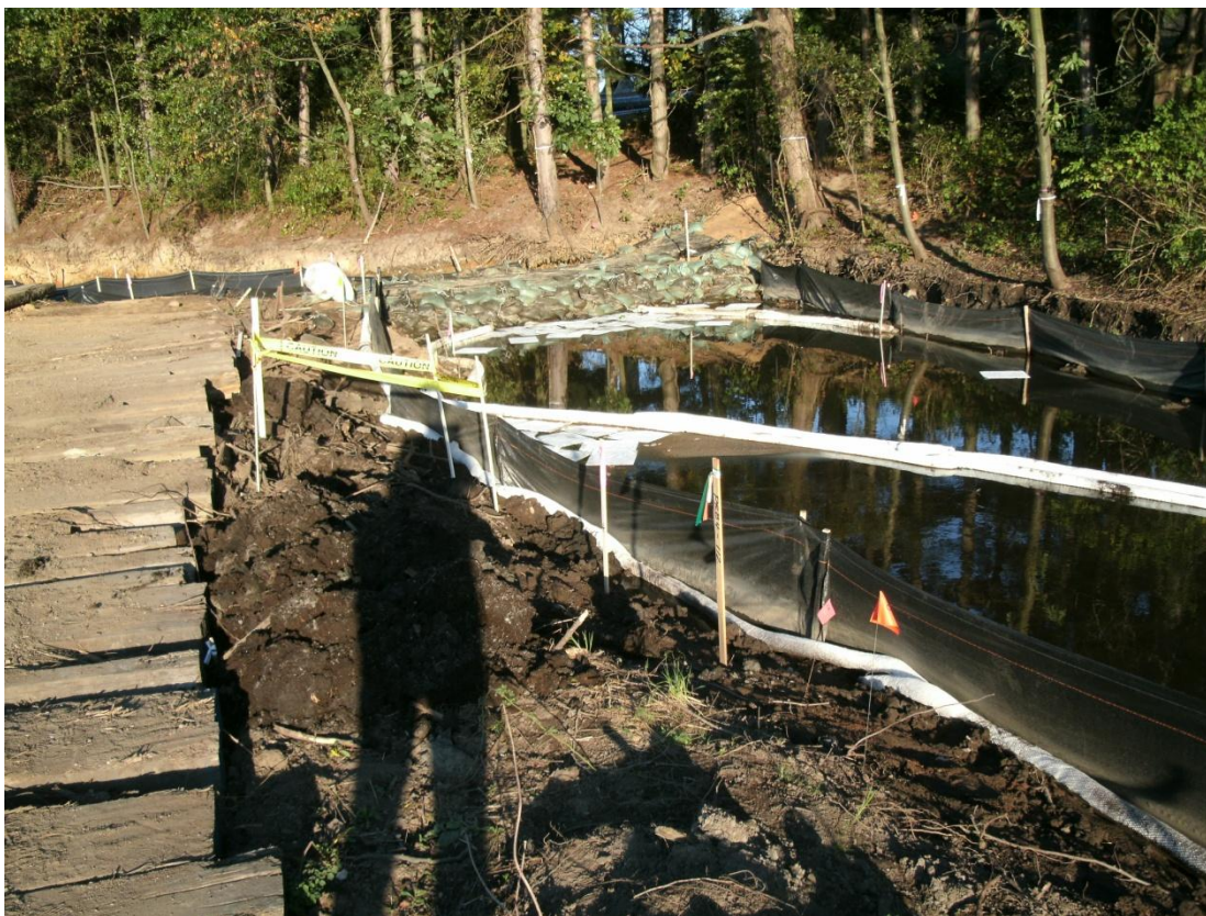
96+50L – 97+00L: Looking downstream (September 14, 2010)
