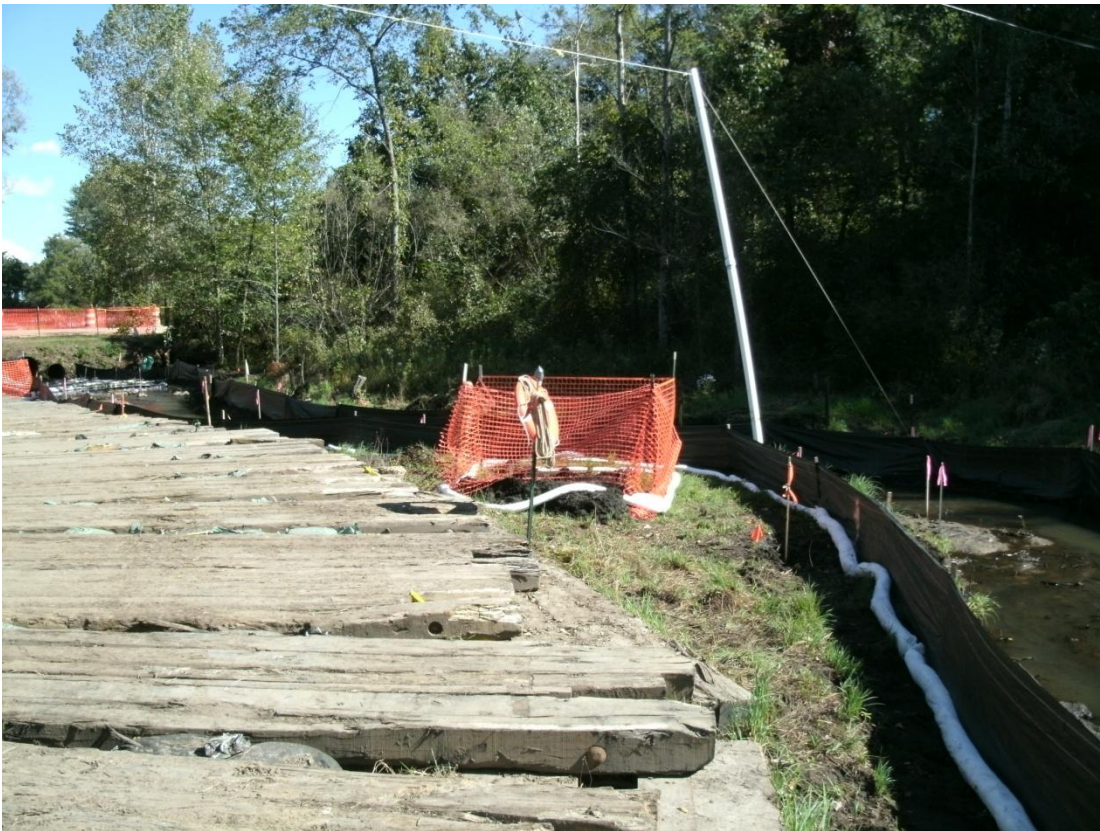
93+50R – 94+00R: Looking upstream (September 13, 2010)
