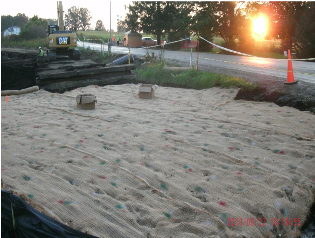
103+00L – 103+50L: Looking from Talmadge Creek (September 22, 2010)
