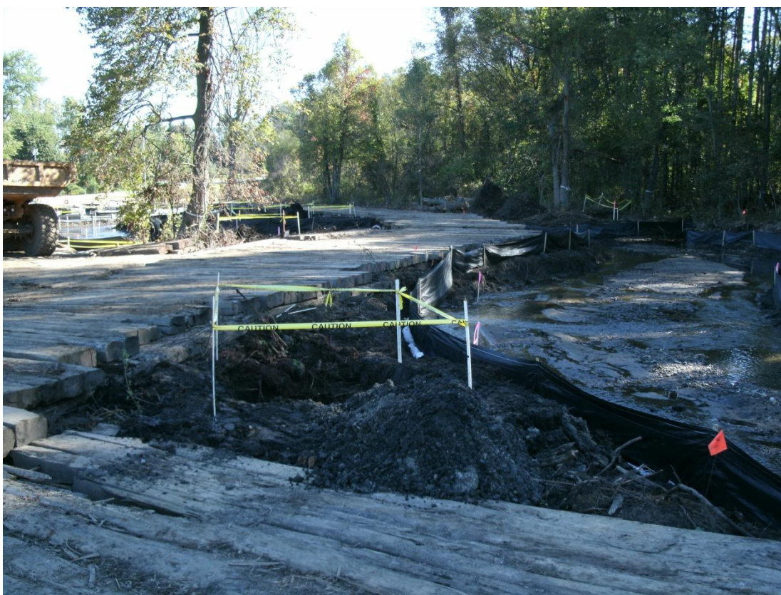
98+50L – 99+00L: Looking downstream (September 14, 2010)
