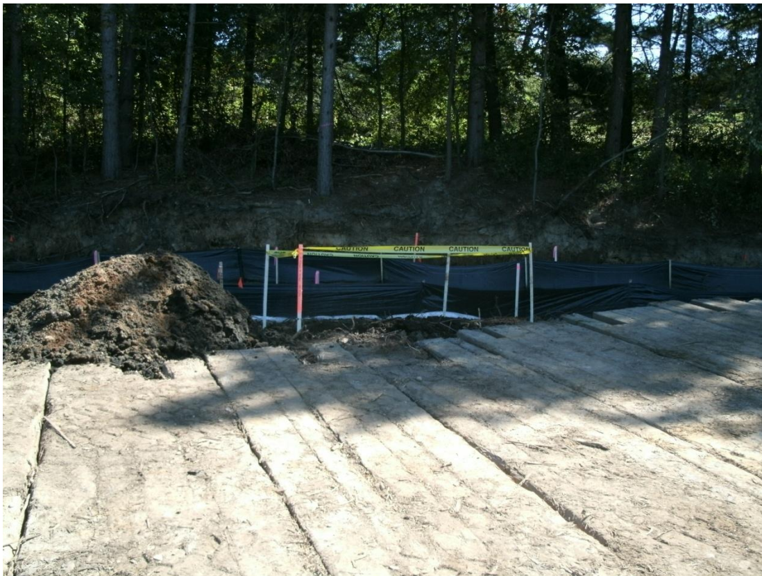
97+00L – 97+50L: Looking toward Talmadge Creek (September 14, 2010)
