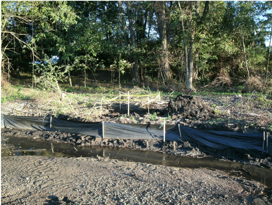
96+00R – 96+50R: Looking from across Talmadge Creek (September 13, 2010)
