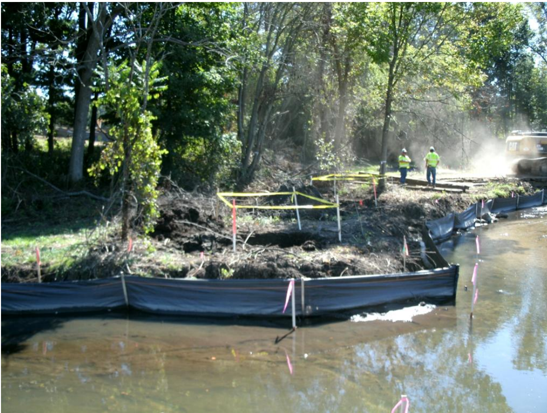
92+50R – 93+00R: Looking across Talmadge Creek (September 14, 2010)
