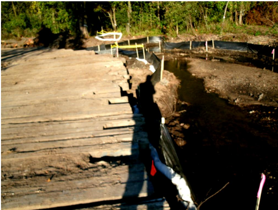
99+00L – 99+50L: Looking downstream (September 14, 2010)
