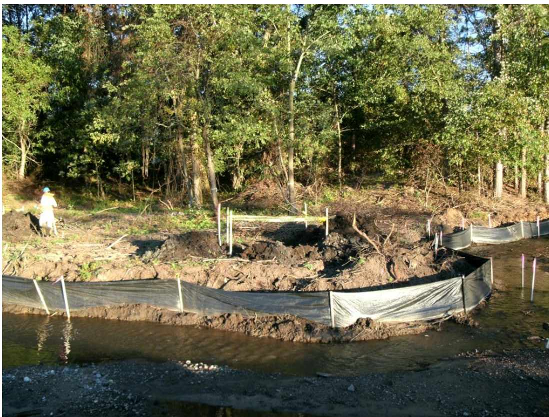
95+50R – 96+00R: Looking from across Talmadge Creek (September 13, 2010)
