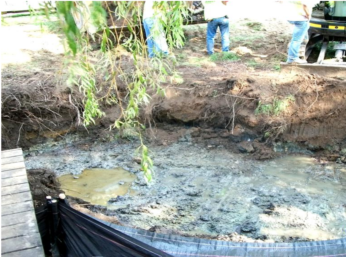
100+00R – 100+50R: Looking from Talmadge Creek (September 21, 2010)
