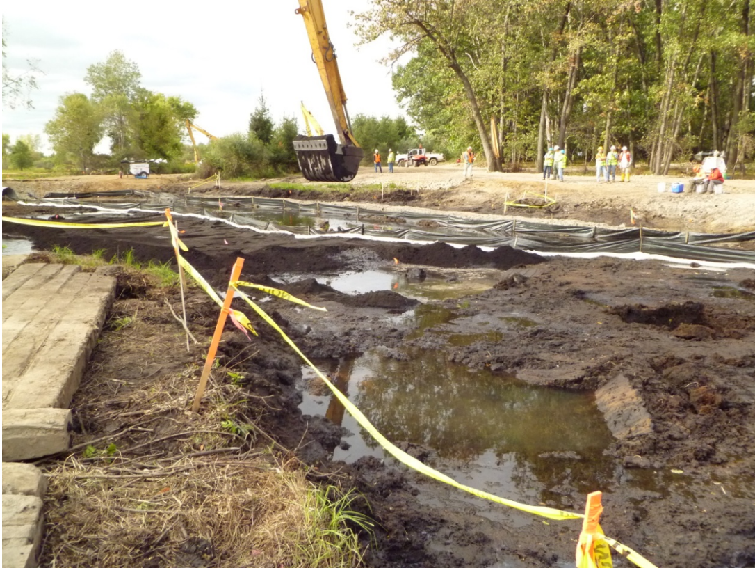
00+00L – 00+50L: Looking downstream prior to backfilling (September 8, 2010)
