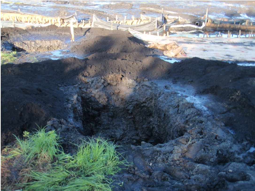
07+00R - 07+50R: Looking toward Talmadge Creek prior to backfill (September 15, 2010)
