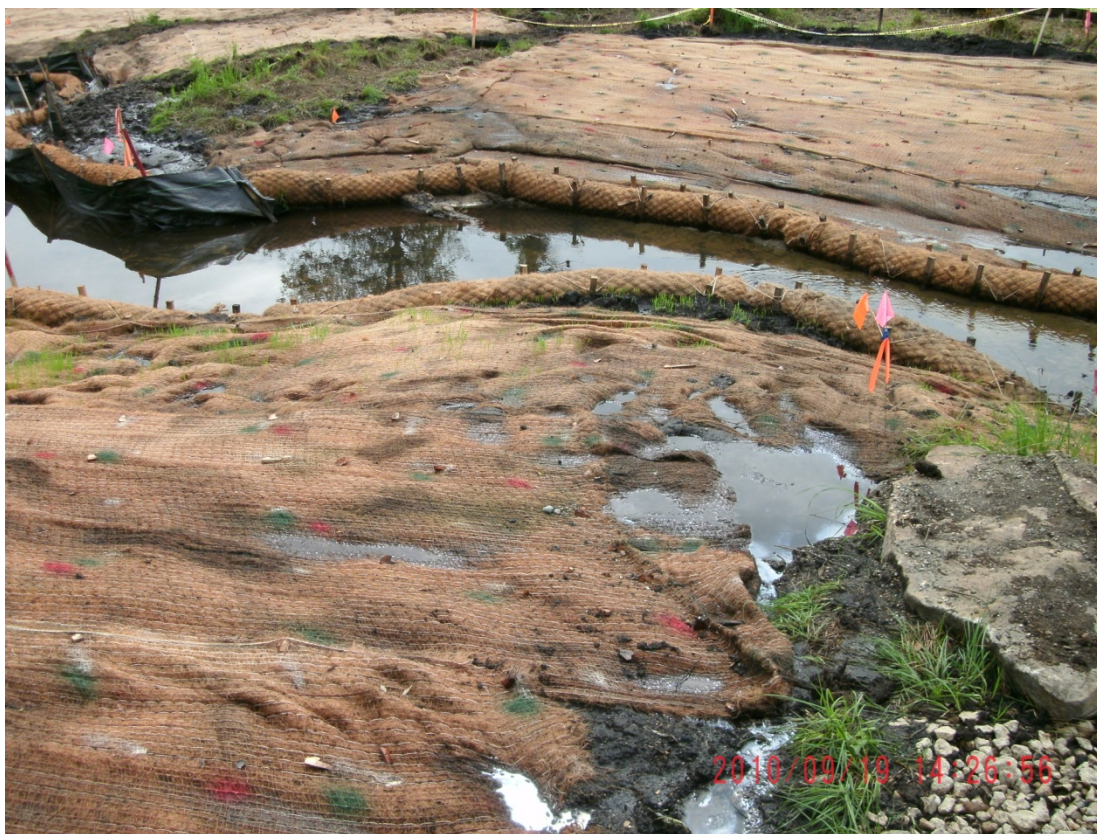
03+00R – 03+50R: Looking toward Talmadge Creek (September 19, 2010)
