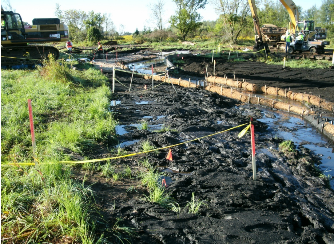
06+50R - 07+00R: Looking downstream prior to backfill (September 12, 2010)
