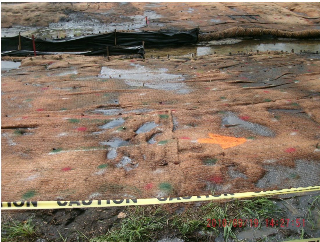
04+00R – 04+50R: Looking toward Talmadge Creek (September 19, 2010)
