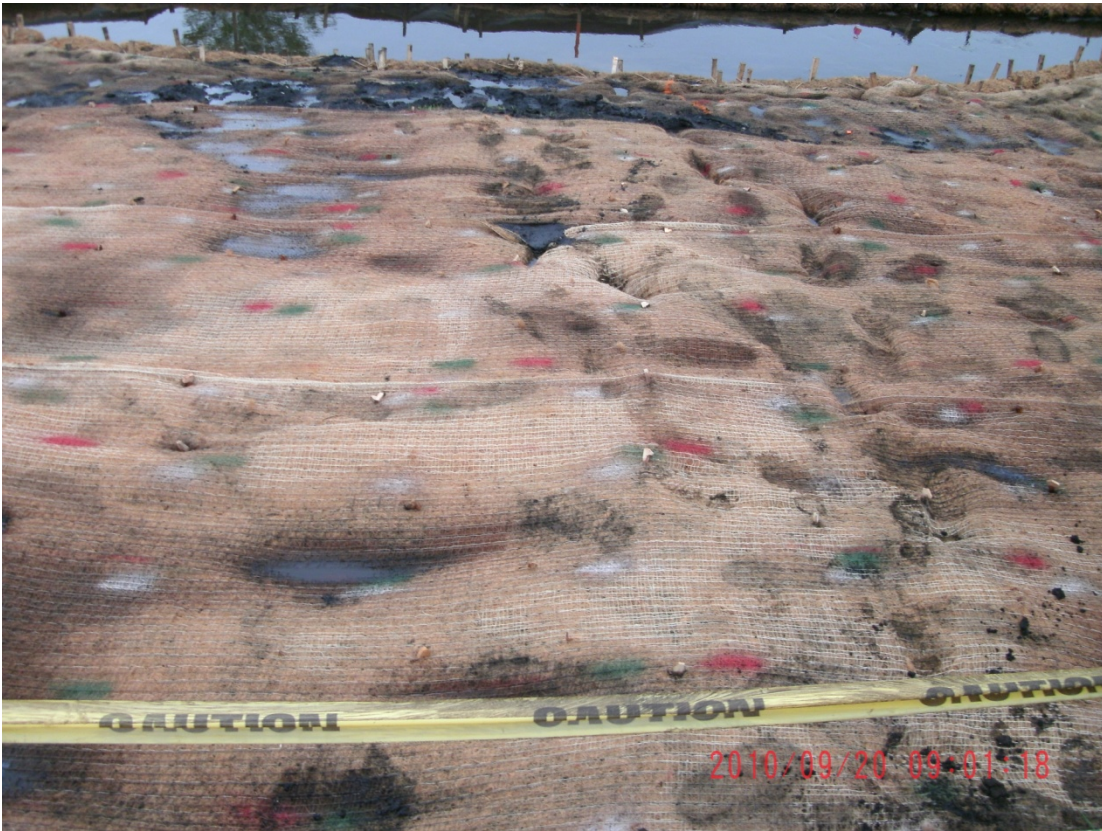
08+50R – 09+00R: Looking toward Talmadge Creek (September 20, 2010)
