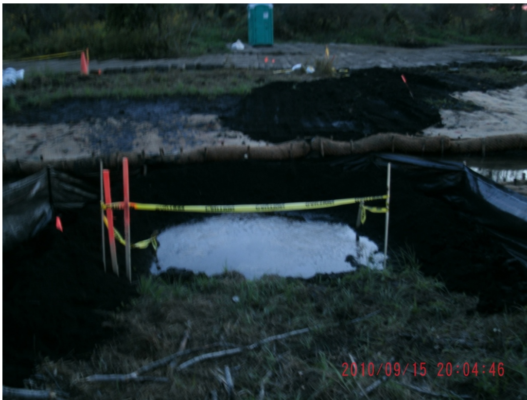
04+50R - 05+00R: Looking toward Talmadge creek at 6-hour test pit (September 15, 2010)
