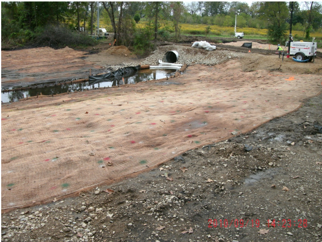
01+50R – 02+00R: Looking toward Talmadge Creek (September 19, 2010)
