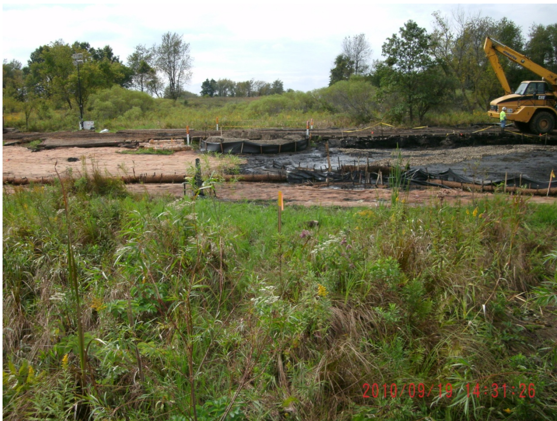
06+00R – 06+50R: Looking toward Talmadge Creek (September 19, 2010)
