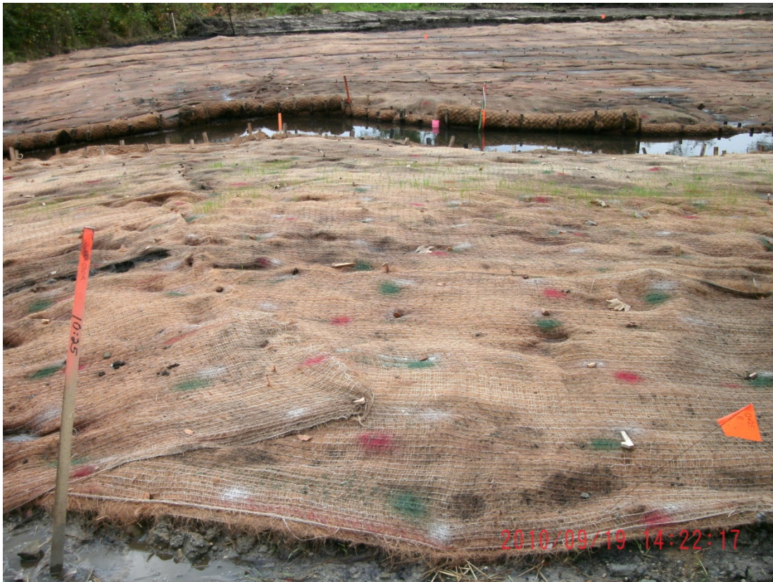
00+00R – 00+50R: Looking toward Talmadge Creek (September 19, 2010)
