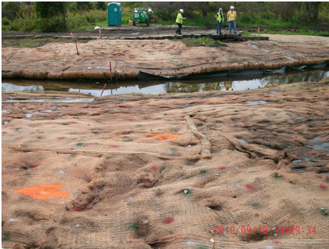
05+00R – 05+50R: Looking toward Talmadge Creek (September 19, 2010)
