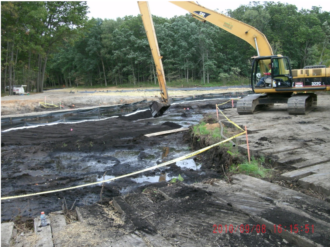
00+50L – 01+00L: Looking upstream at backfilling (September 8, 2010)
