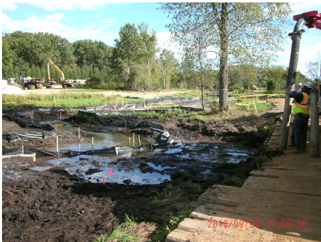
08+00L – 08+50L: Looking upstream prior to final excavation (September 9, 2010)
