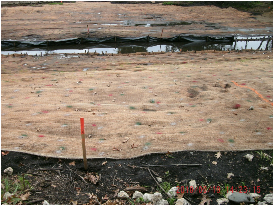
01+00R – 01+50R: Looking toward Talmadge Creek (September 19, 2010)
