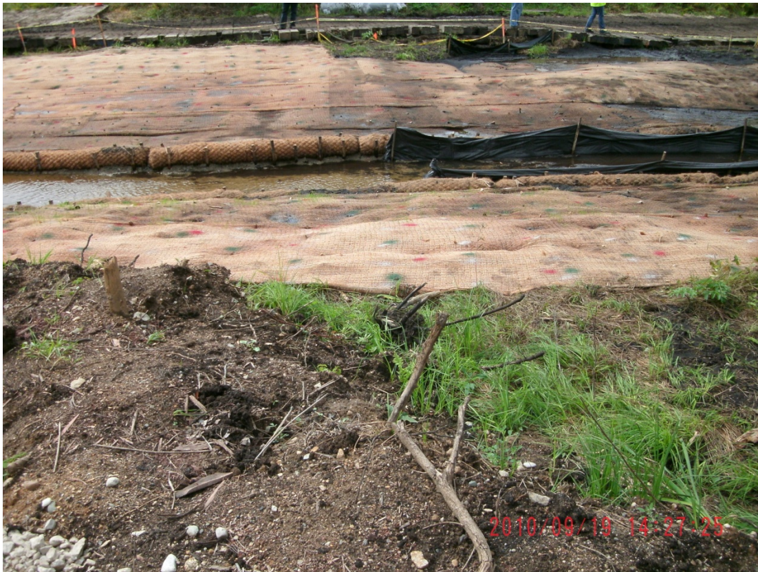
03+50R – 04+00R: Looking toward Talmadge Creek (September 19, 2010)
