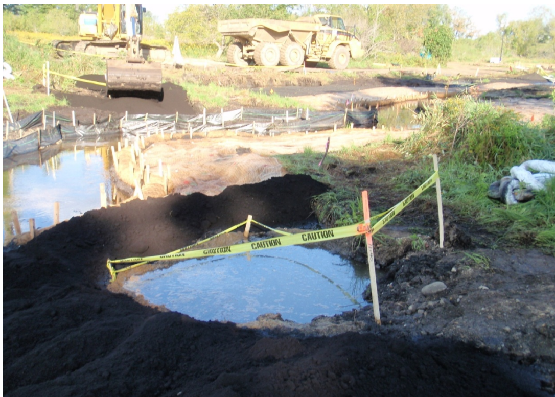
02+50R - 03+00R: Looking downstream (September 15, 2010)
