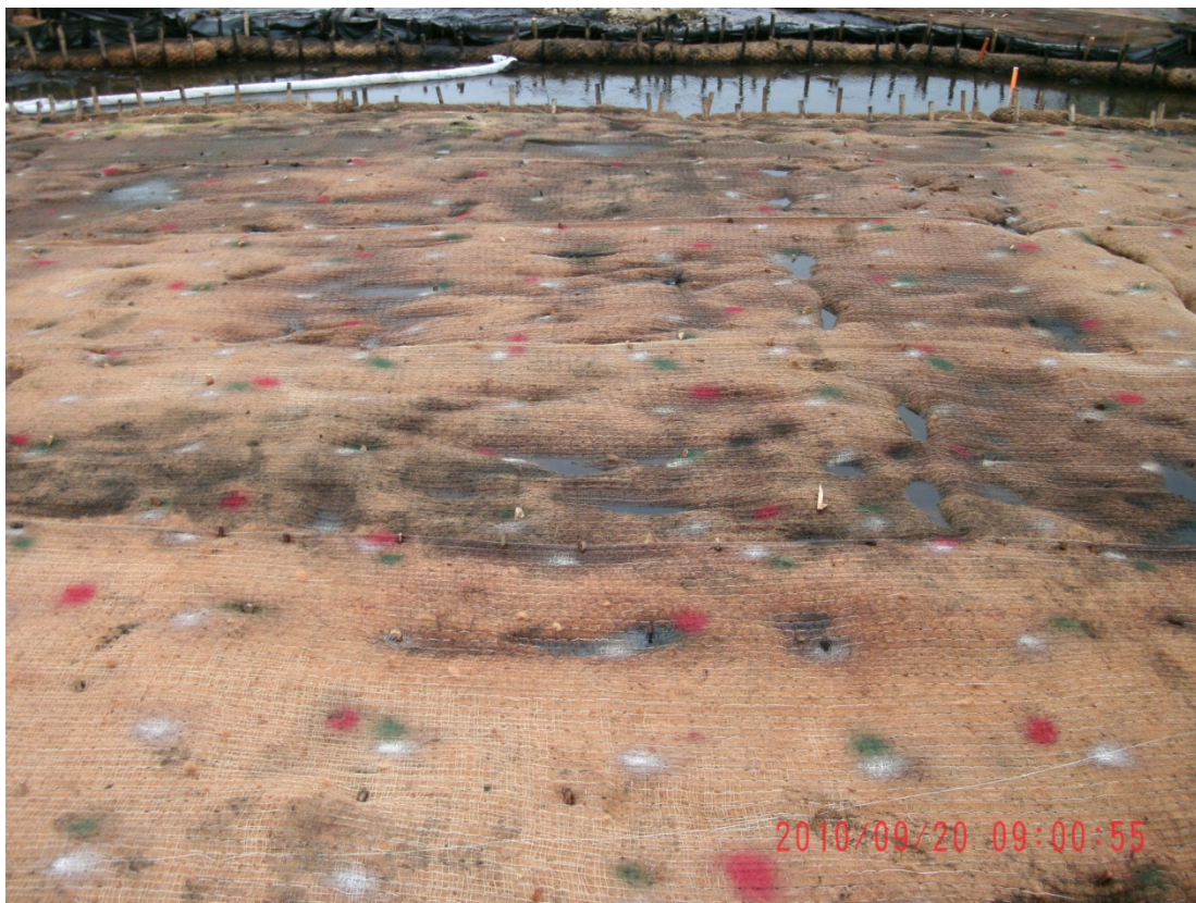
08+00R – 08+50R: Looking toward Talmadge Creek (September 20, 2010)
