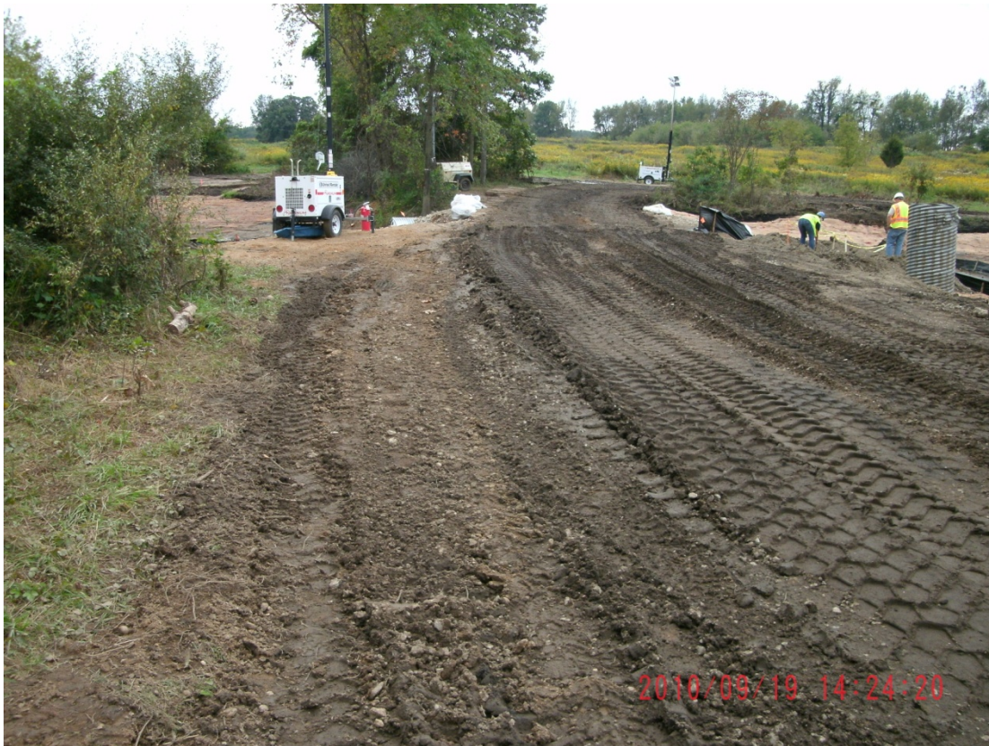
02+00R – 02+50R: Looking at road over Talmadge Creek (September 19, 2010)
