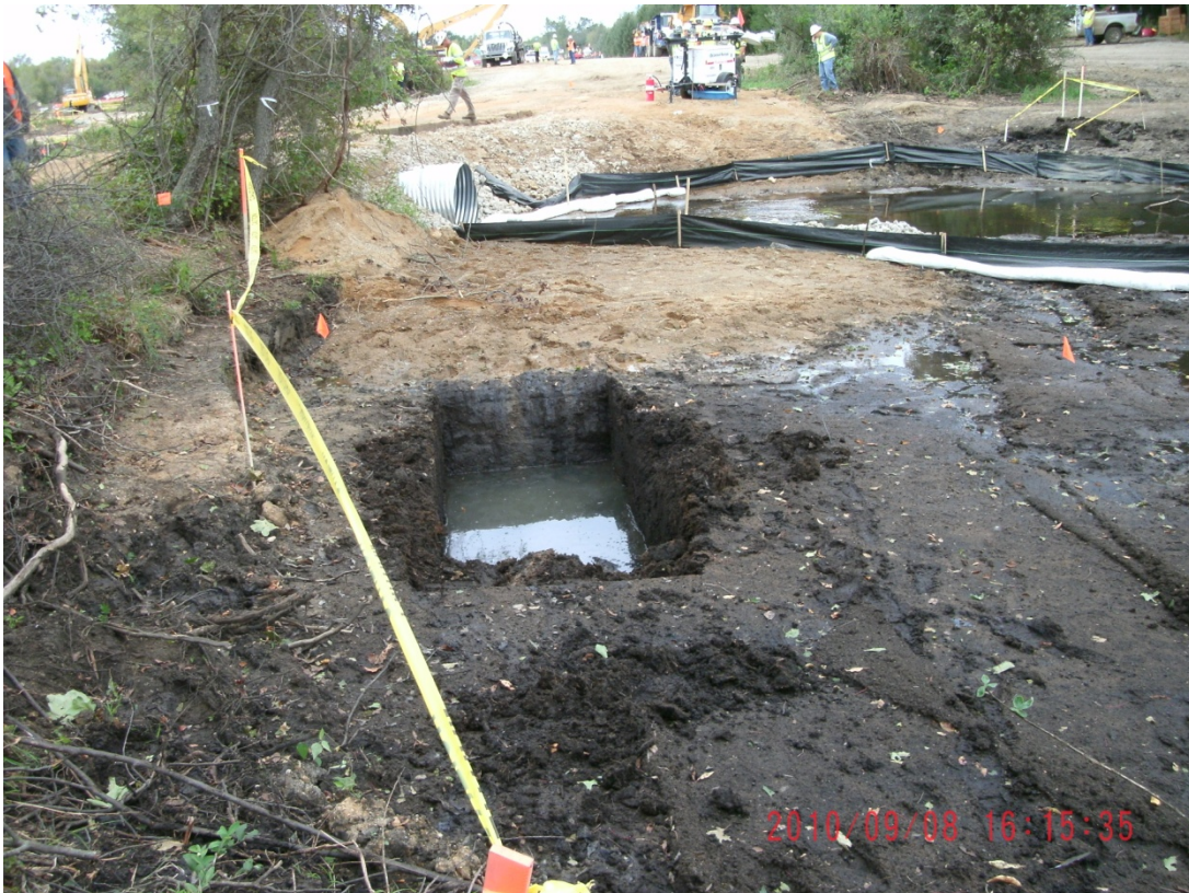
01+50L – 01+75L: Looking downstream at 6-hour test pit (September 8, 2010)
