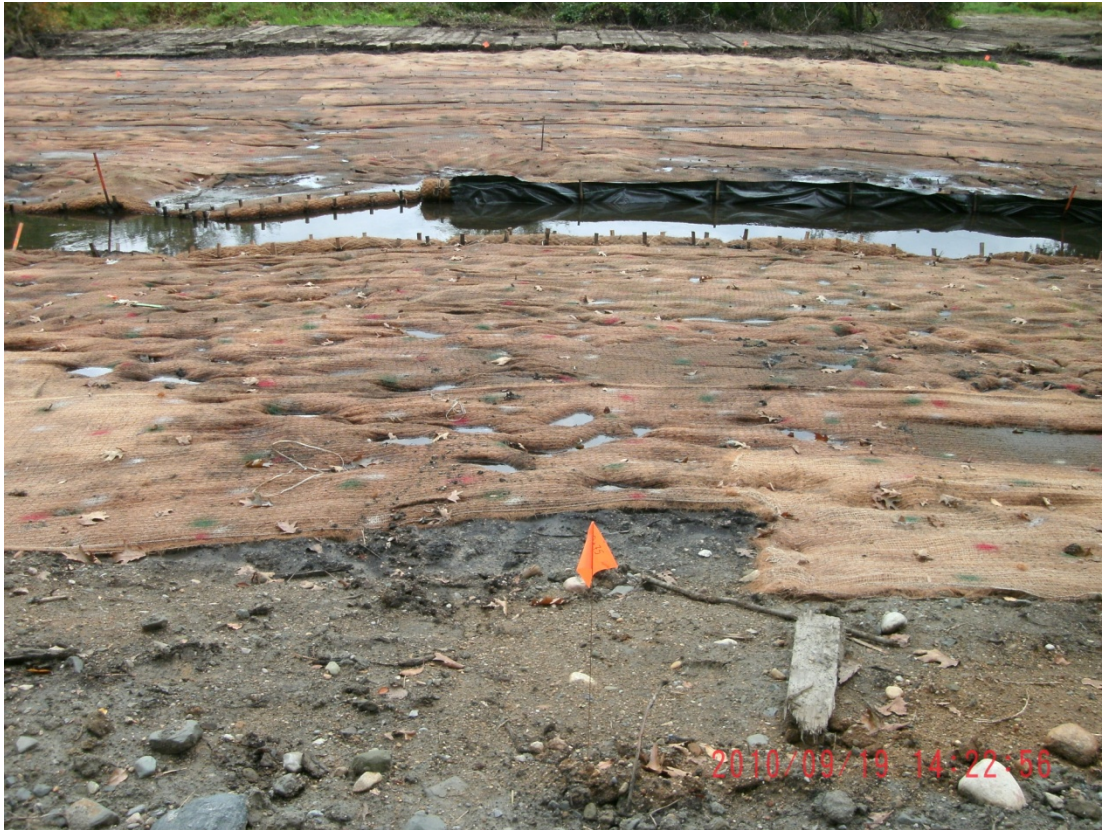
00+50R – 01+00R: Looking toward Talmadge Creek (September 19, 2010)
