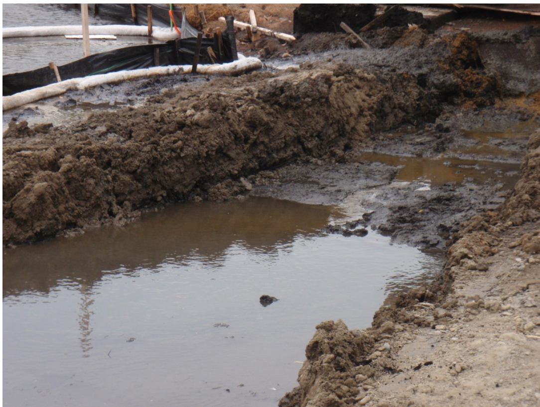
00-50R – 00+00R: Looking at test pit (September 25, 2010)
