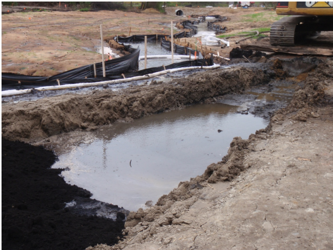
00-50R – 00+00R: Looking downstream (September 25, 2010)
