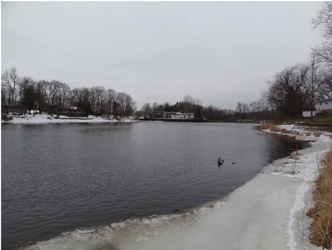
5. Ceresco Dam Impoundment River icing conditions.
