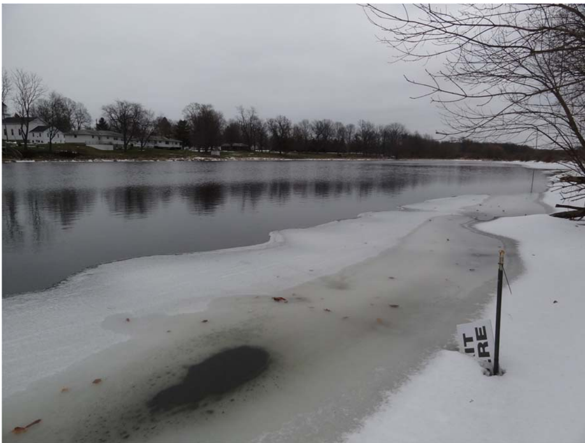
9. Ceresco Dam Impoundment River icing conditions.
