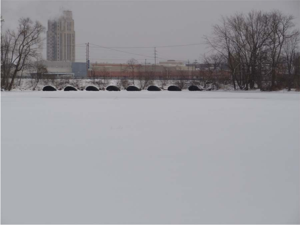
11. MP15.75 North Mill Pond culverts, observed the river completely frozen over.
