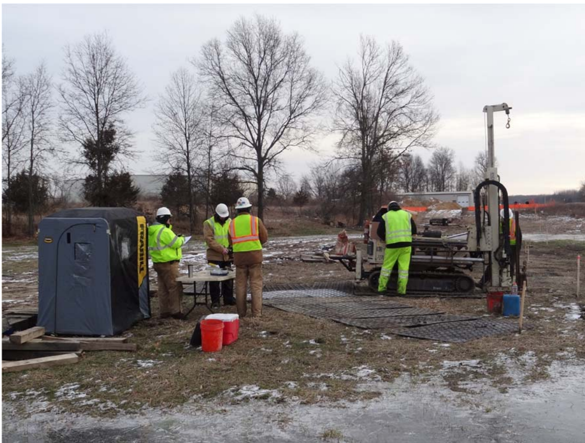
1. Source area observed a crew collecting soil cores.
