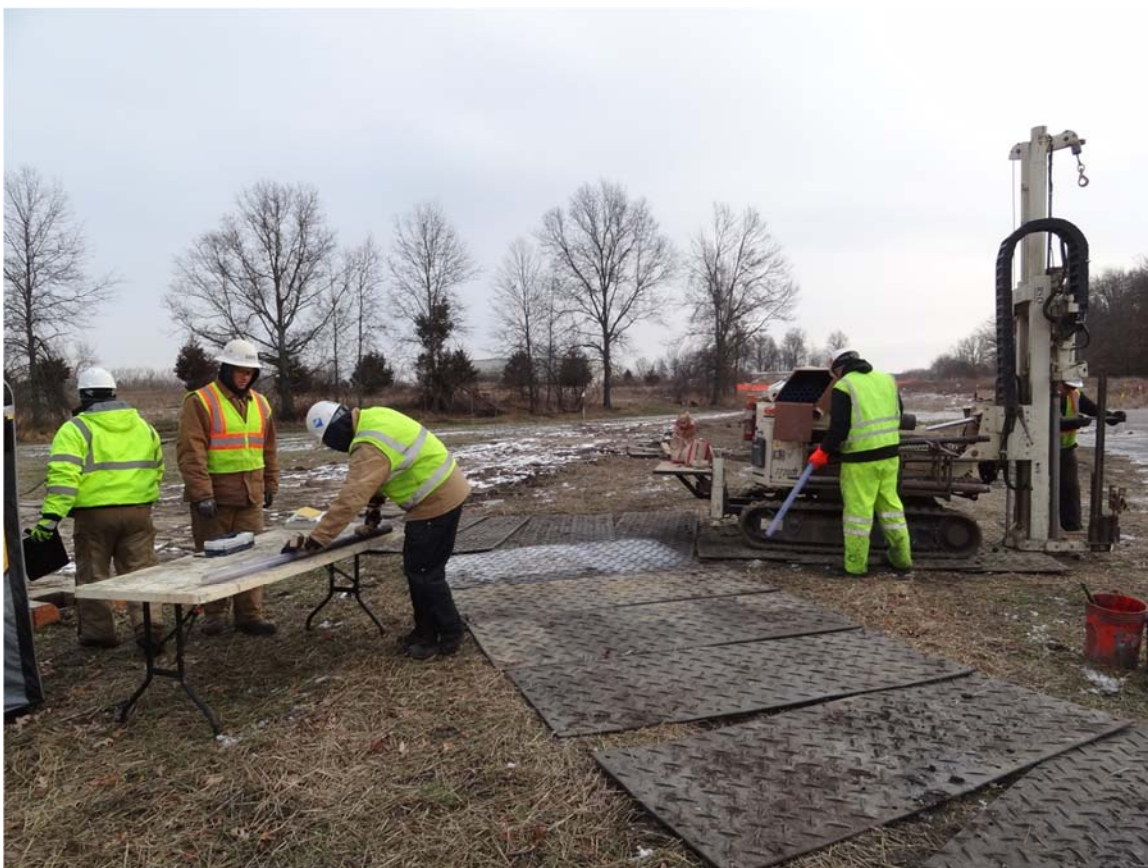
2. Source area observed a crew collecting soil cores.
