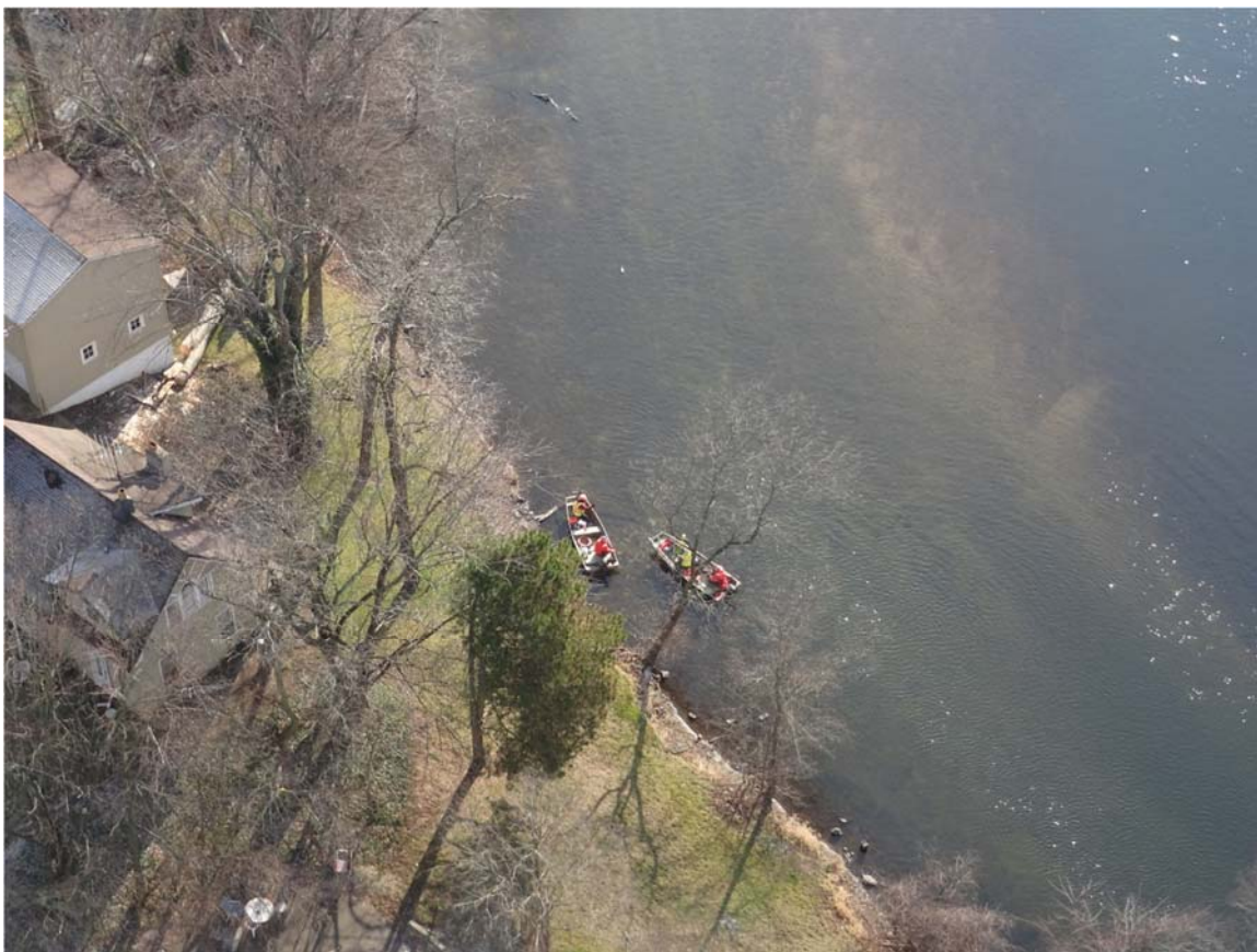
19. Poling crew observed below Morrow Lake Dam.
