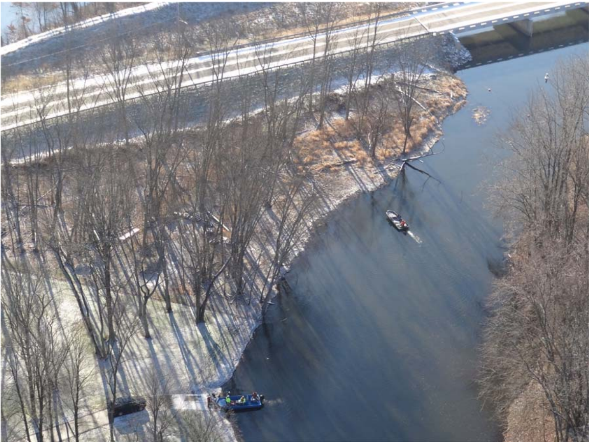
12. MP21.5 Sediment Trap observed a bathymetry crew.
