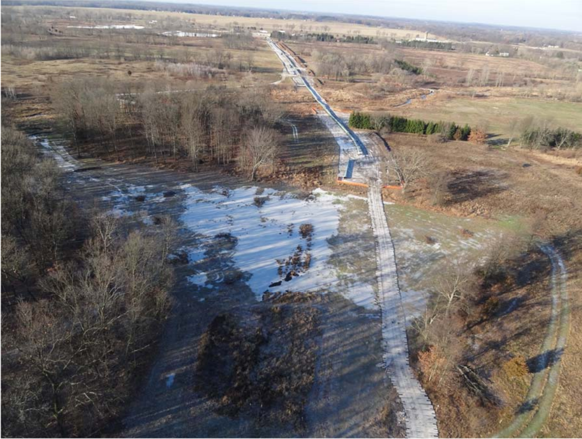
1. Source Area observed the pipeline installation preparation work continuing at the source area and across Talmadge Creek.
