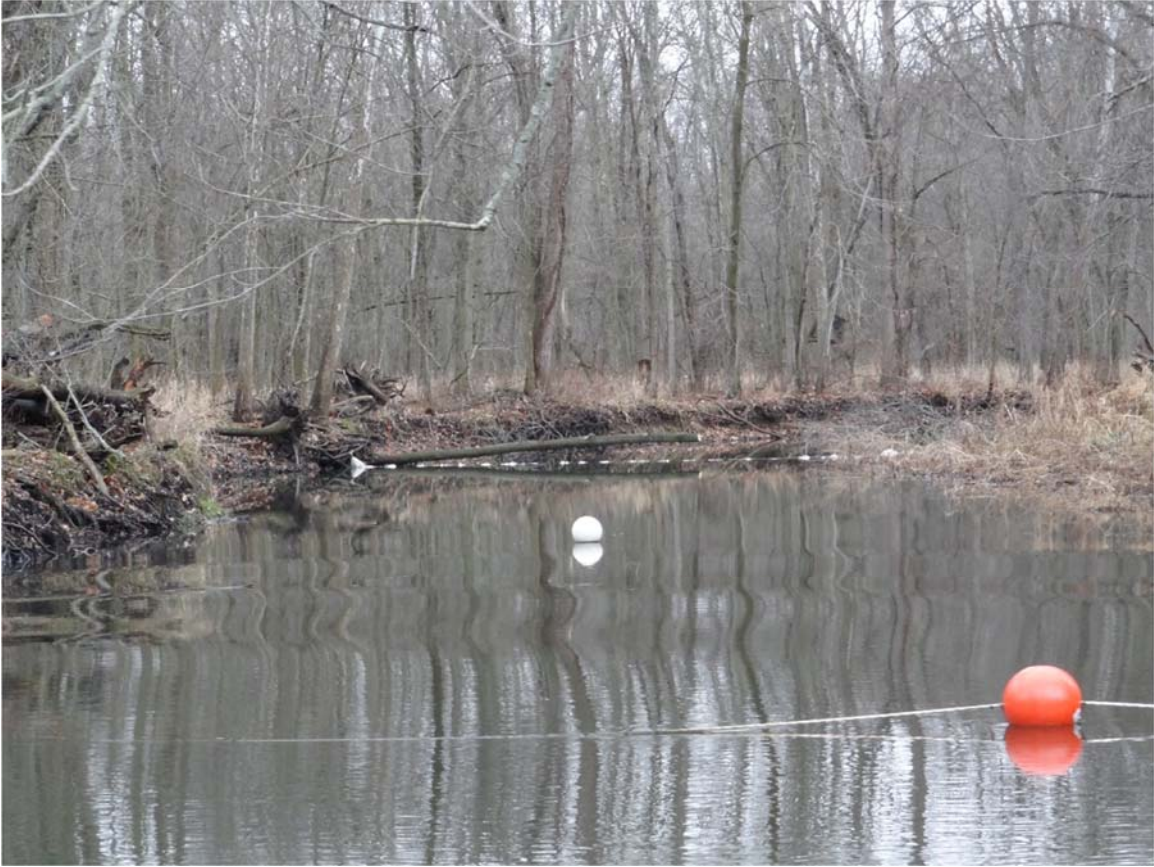
19. MP28.25 Snare boom remains across the channel to collect sheen and tar globs generated by the bathymetry team.
