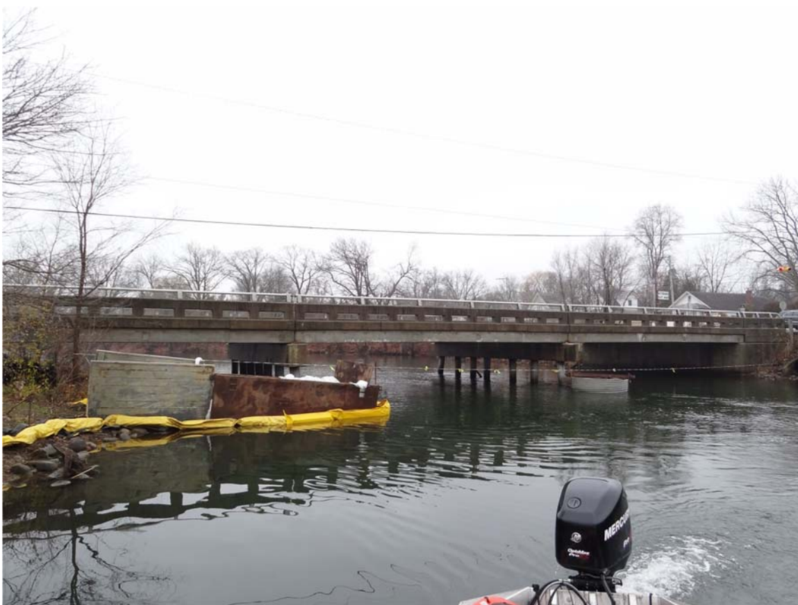
20. MP15.5 Burnham Street Bridge utility work continued, new obstructions observed in the river channel.
