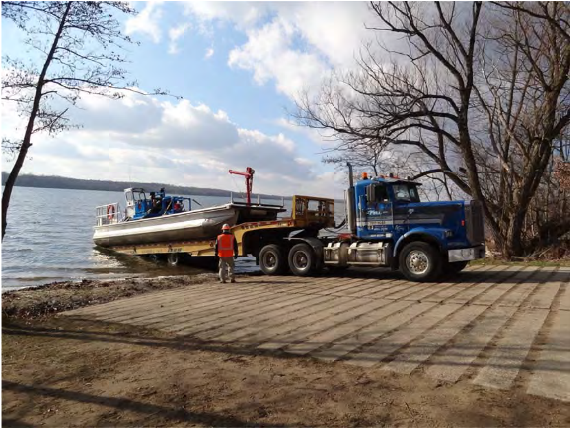
17. E4.0 boat launch, crews observed unloading pontoon boat to be used for boom anchor removal.
