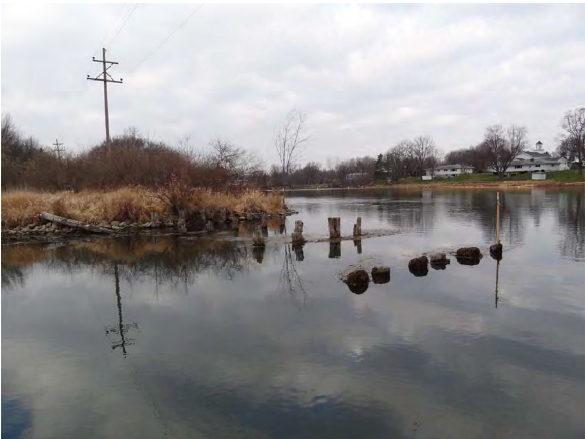
2. Ceresco Dam trestle, no sheen observed.
