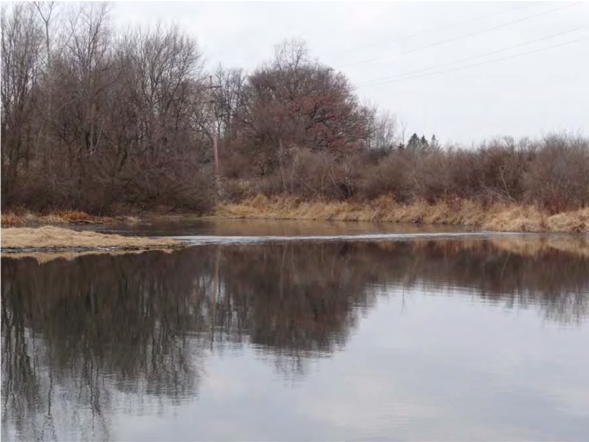
1. MP5.63 LDB, bank ice observed along river shoreline on upstream side of trestle.
