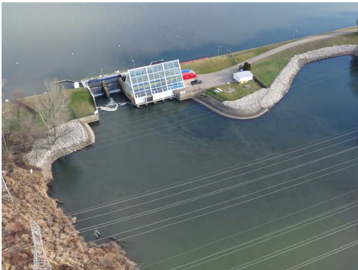
20. Morrow Lake Dam. No ice observed.
