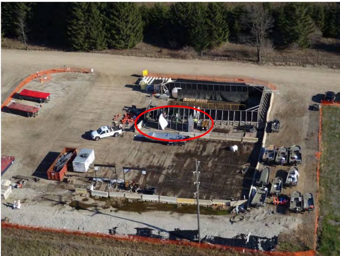
2. Frac Tank City, crews observed constructing shelter adjacent to decon area.
