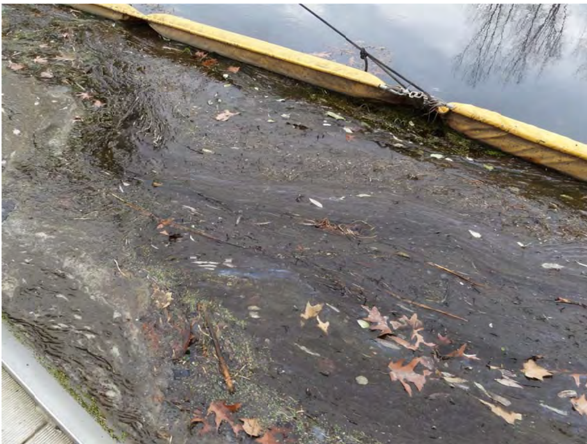
7. Ceresco Dam control point, sheen observed within containment.
