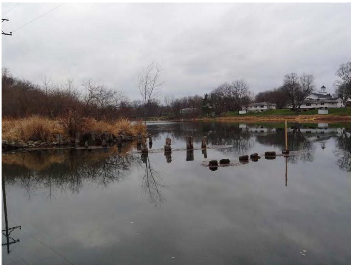
2. Ceresco Dam trestle, no sheen observed.
