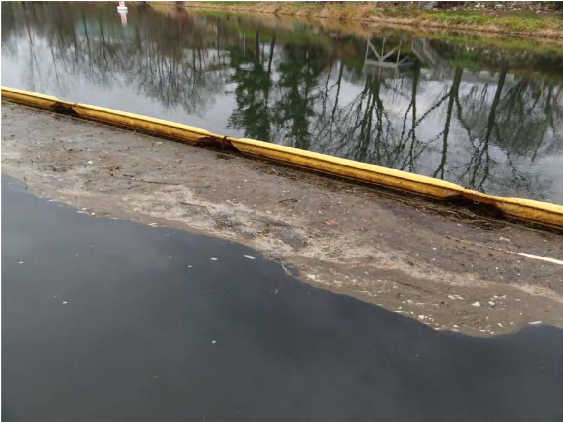
5. Ceresco Dam control point boom, some debris and sheen observed.
