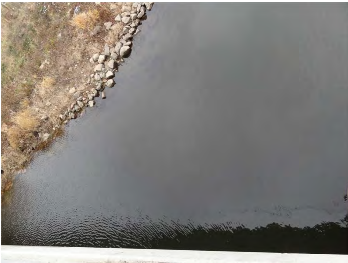
21. MP21.5 Custer Bridge no sheen or ice observed.
