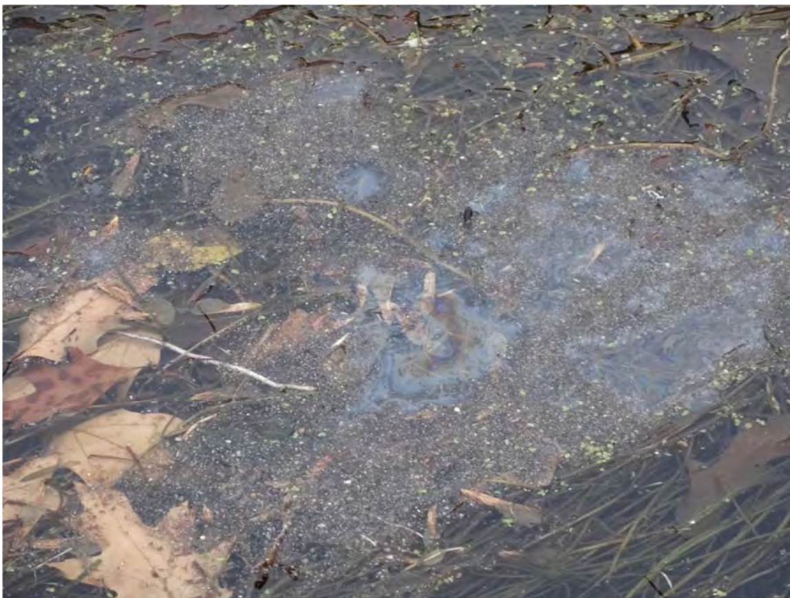
6. Ceresco Dam control point, observed sheen and tar globs collecting within the debris along the boom.
