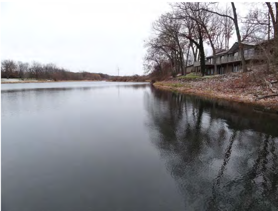
8. Ceresco Dam impoundment no ice observed forming along the LDB.
