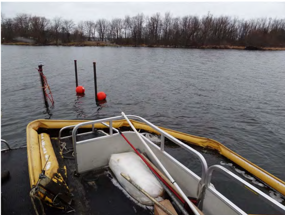
15. SWAT crew replaced the section of boom marking the anchor poles.
