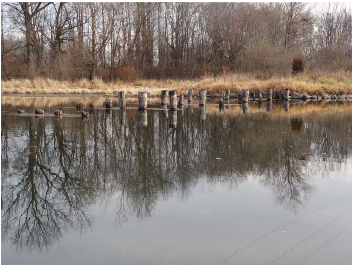
1. MP5.63 RDB, Ceresco Dam trestle, no sheen observed.
