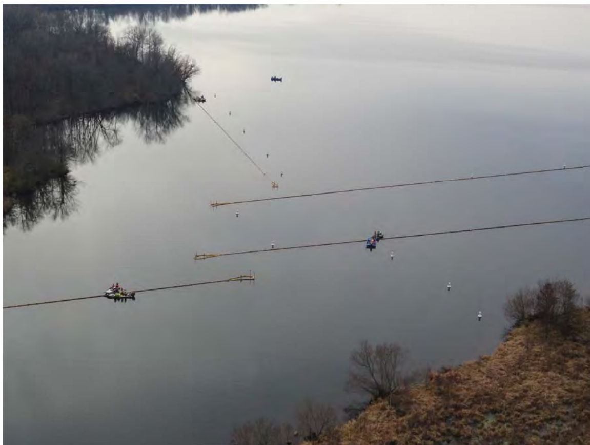
13. E4 containment system, observed post-curtain removal bathymetry survey crews along Boom E in western end of delta.
