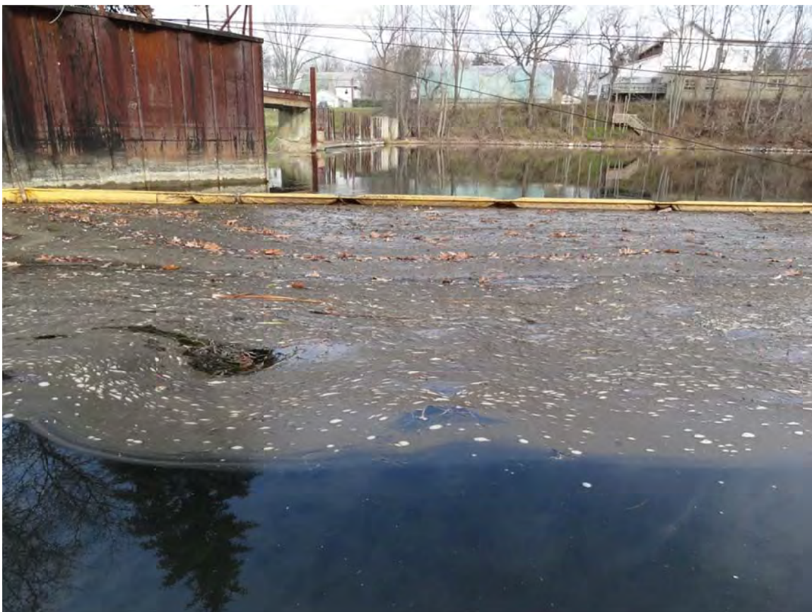
3. Debris observed along Ceresco Dam control point.
