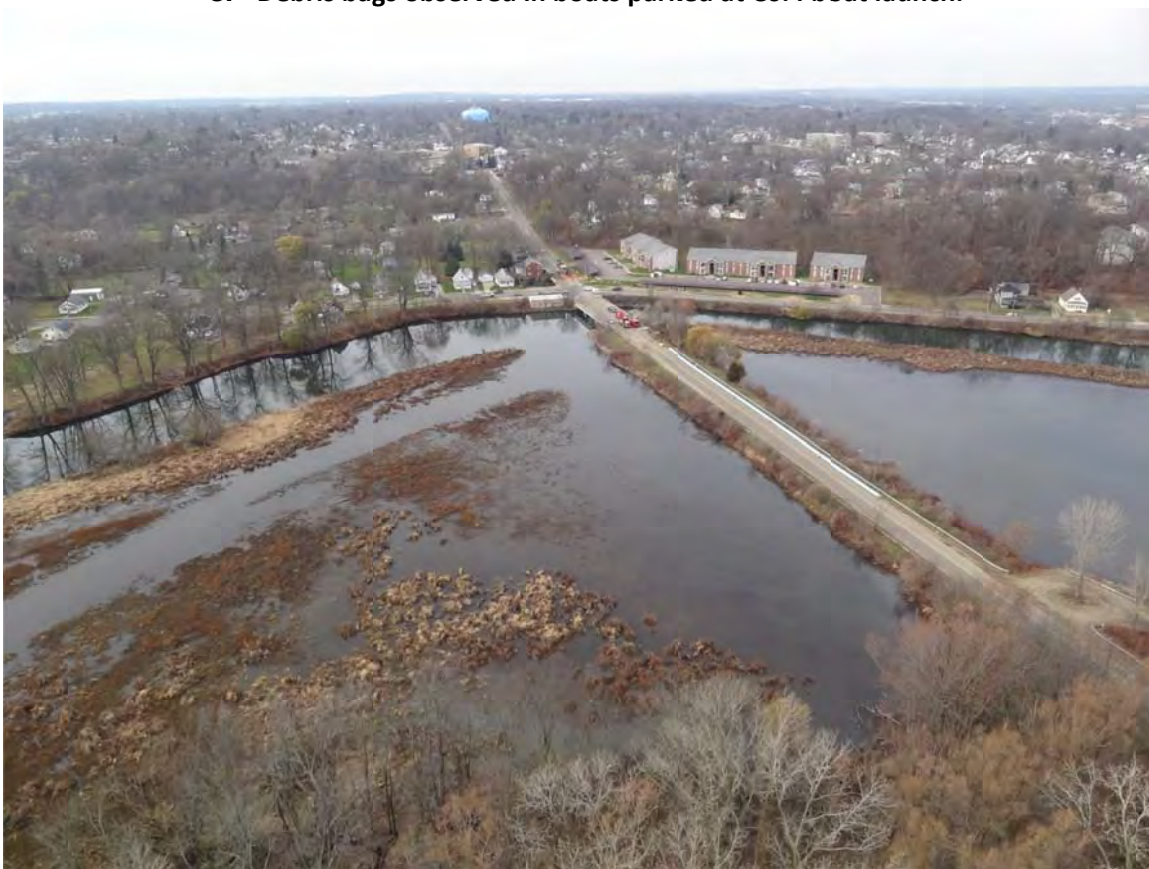
6. Mill Ponds, no sheen observed.
