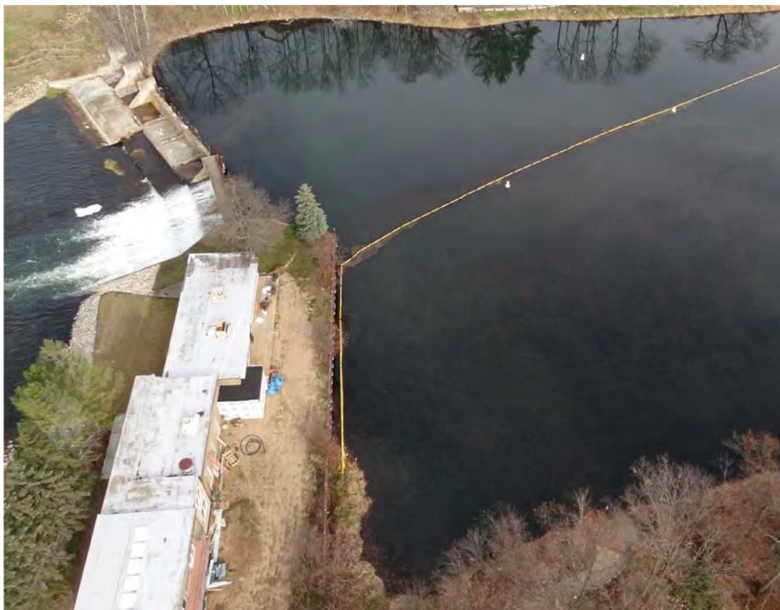
4. Ceresco Dam during afternoon overflight, debris had been removed from containment boom.
