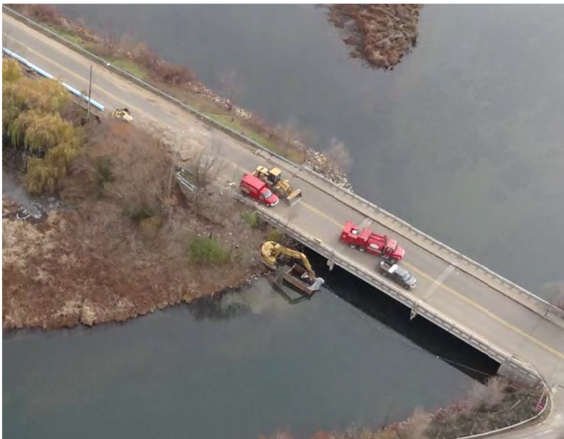
7. Observed crews installing utility piping in river at Burnham Street Bridge (Mill Ponds).
