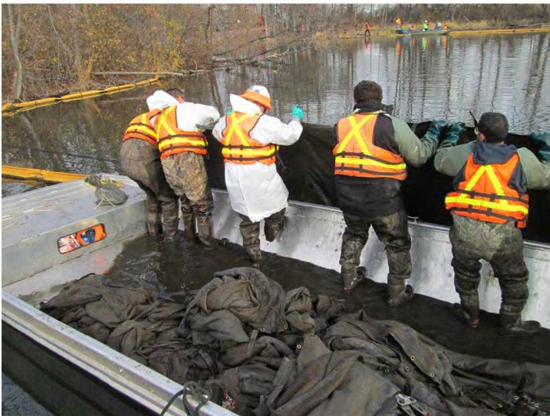
20. Observed crews removing sediment curtain from boom in Morrow Lake.
