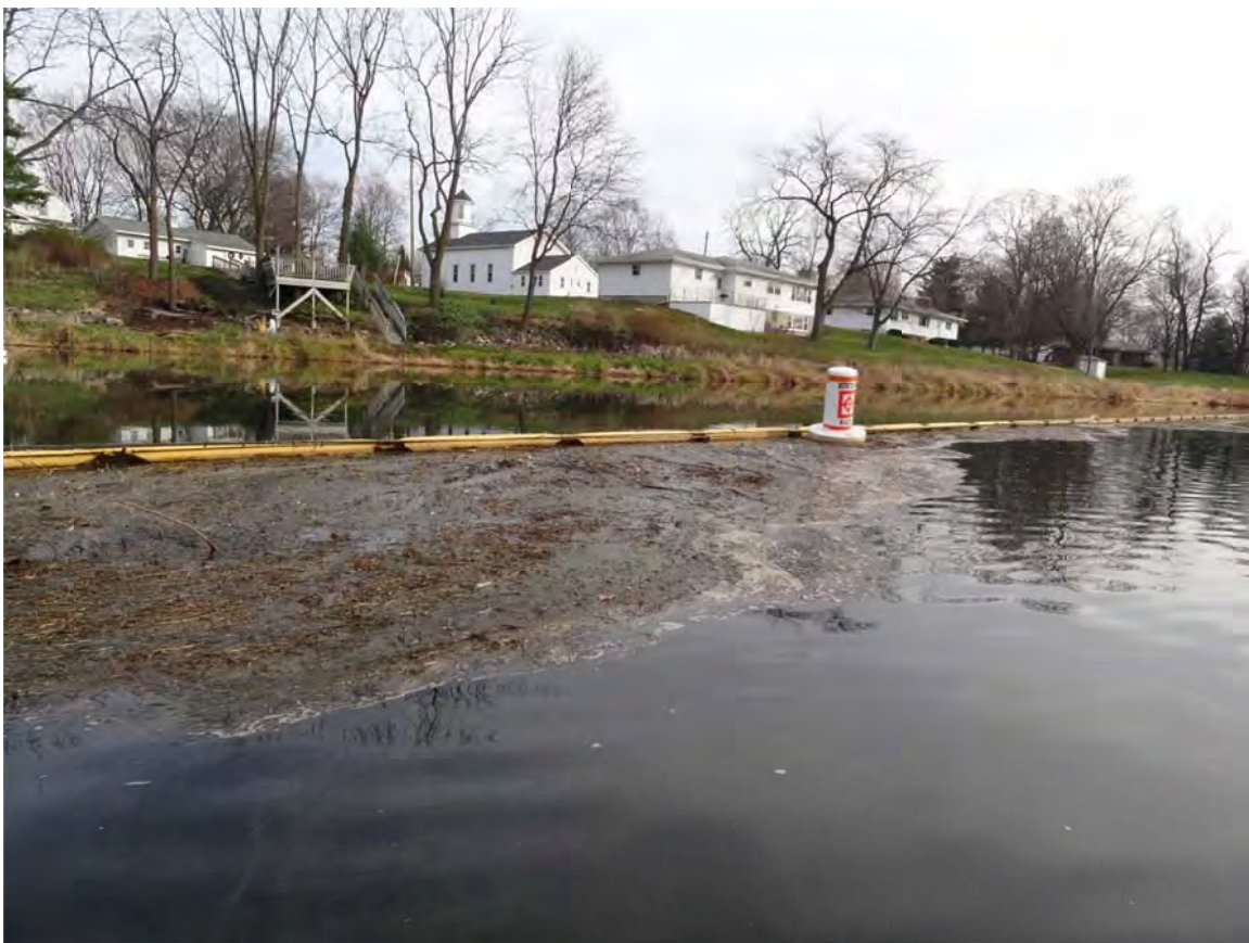
2. MP5.75 Ceresco Dam control point, debris observed along containment boom.
