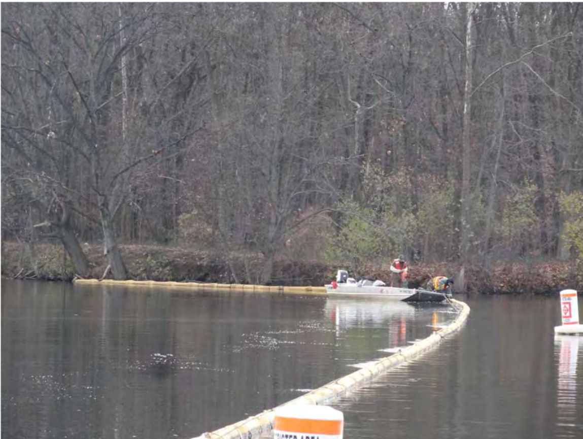
30. Morrow Lake Delta Gate C observed a crew inspecting the curtain.
