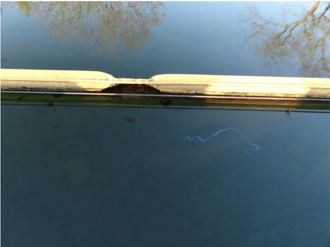
8. Ceresco Dam observed sheen collecting along the control point boom.
