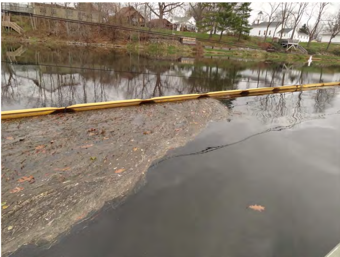
2. Ceresco Dam control point, sheen and debris observed.
