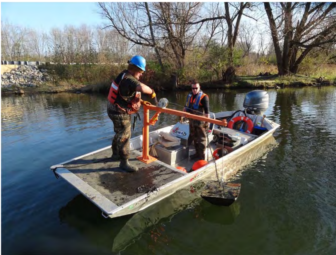
5. MP36.5 observed a crew removing a Walling Tube anchor.
