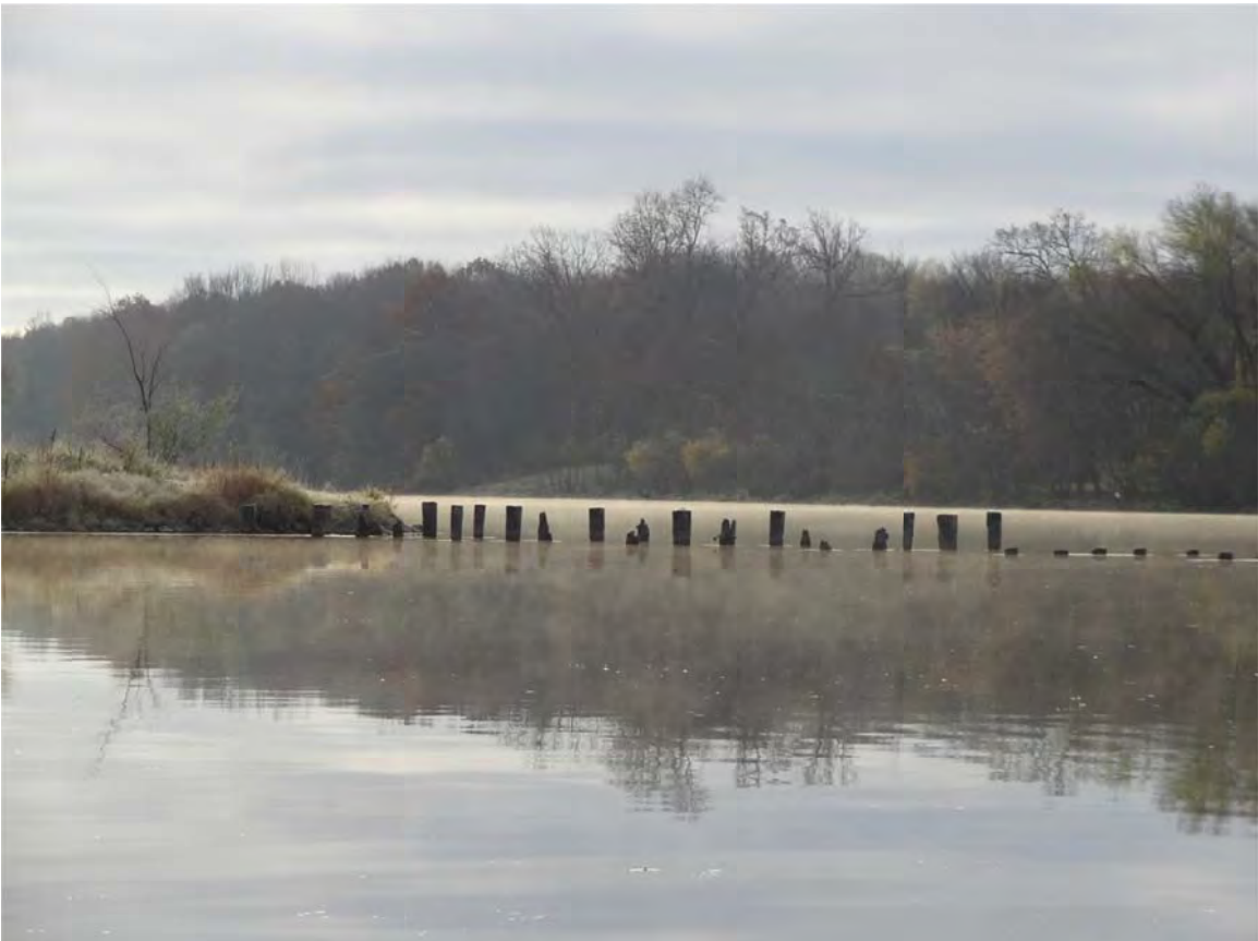
4. View from trestle at MP 5.75, no sheen observed.
