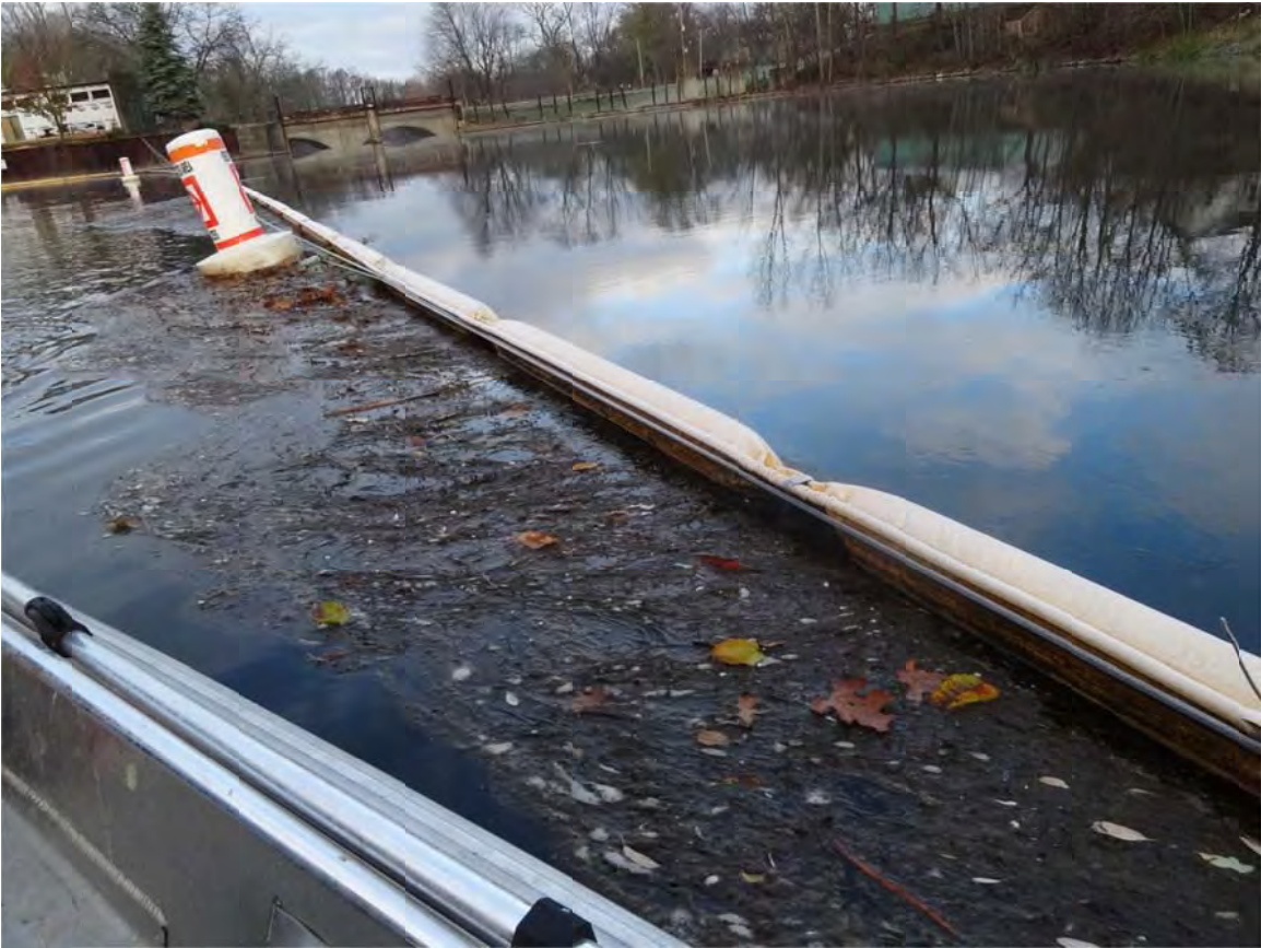
3. Debris along Ceresco Dam control point.
