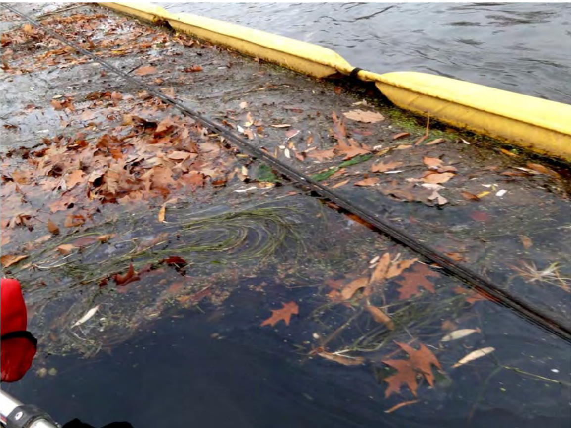
10. Ceresco Dam control point, sheen and tar globules observed within debris at containment point.
