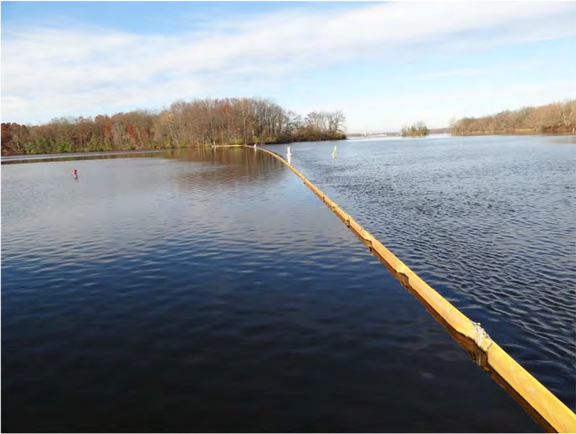
7. Morrow Lake Delta Gate C observed sheen and tar globs collecting along the boom.
