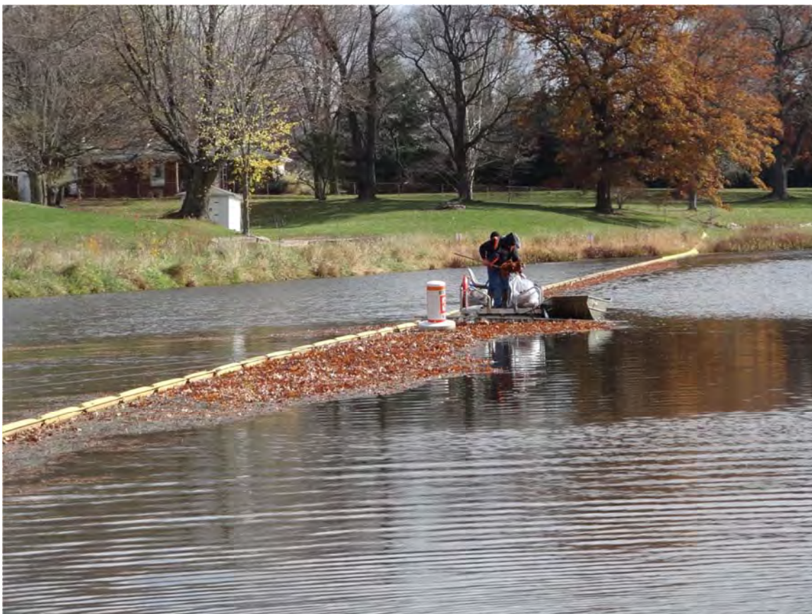
10. Ceresco Dam observed removing debris collecting along the boom.
