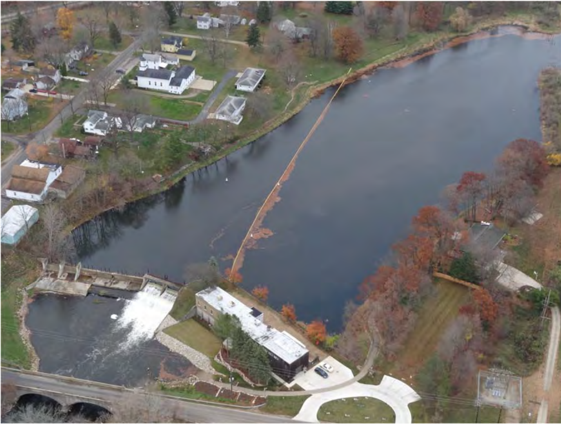
3. Ceresco Dam overview.
