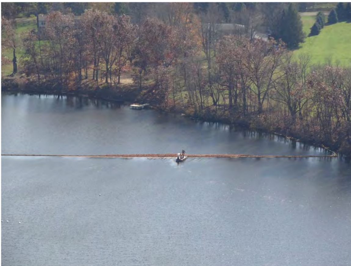
33. Morrow Lake Delta observed a crew removing debris from Gate B.
