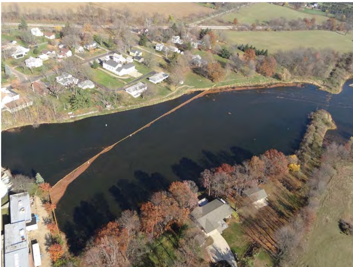
5. Ceresco Dam control point boom.
