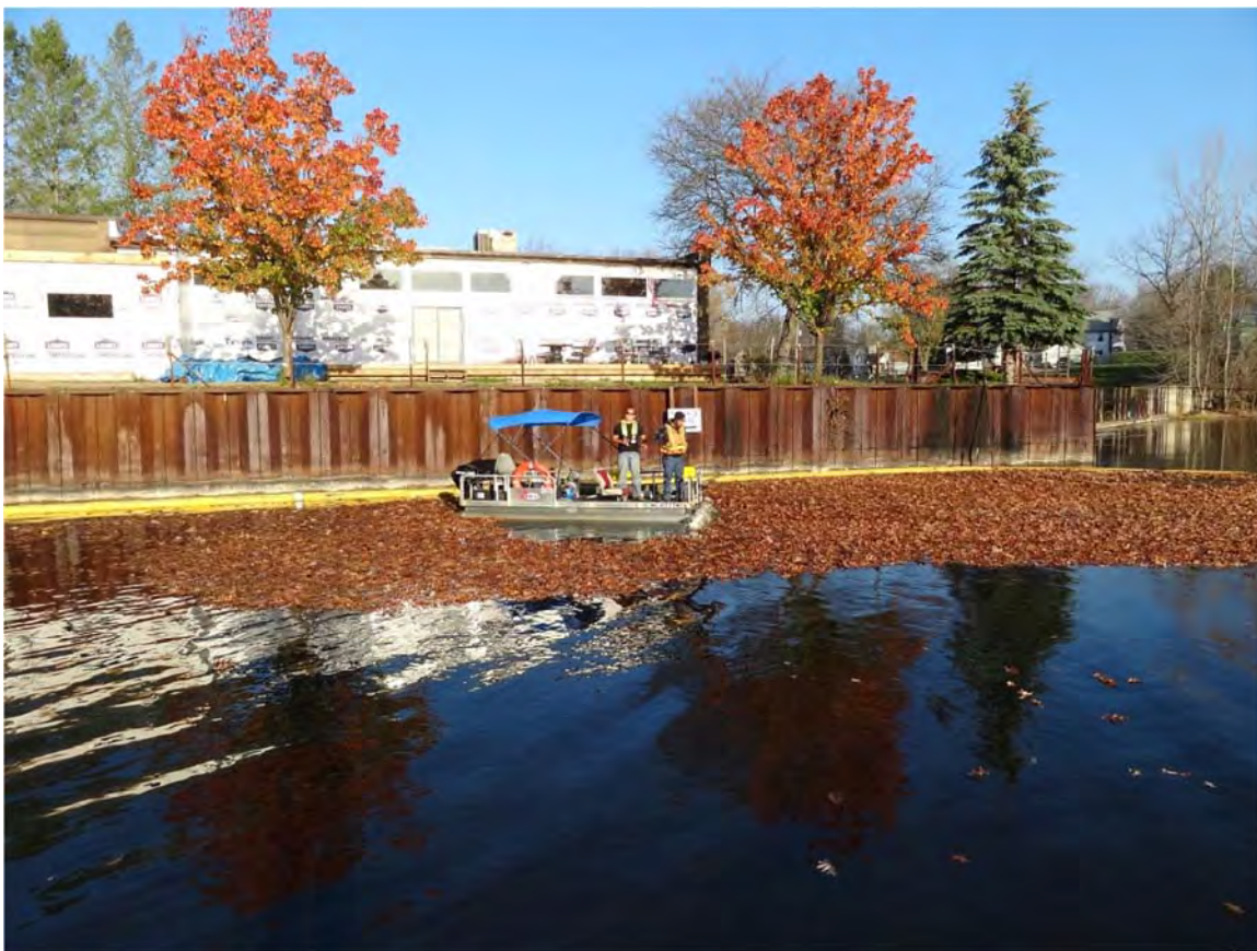
9. Ceresco Dam observed a crew preparing to remove debris from the control point boom.
