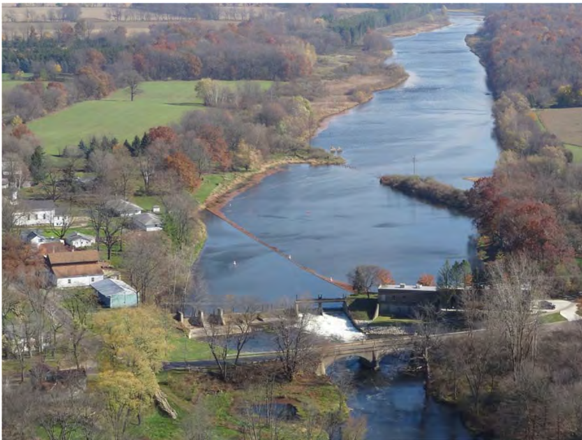
4. Ceresco Dam overview.
