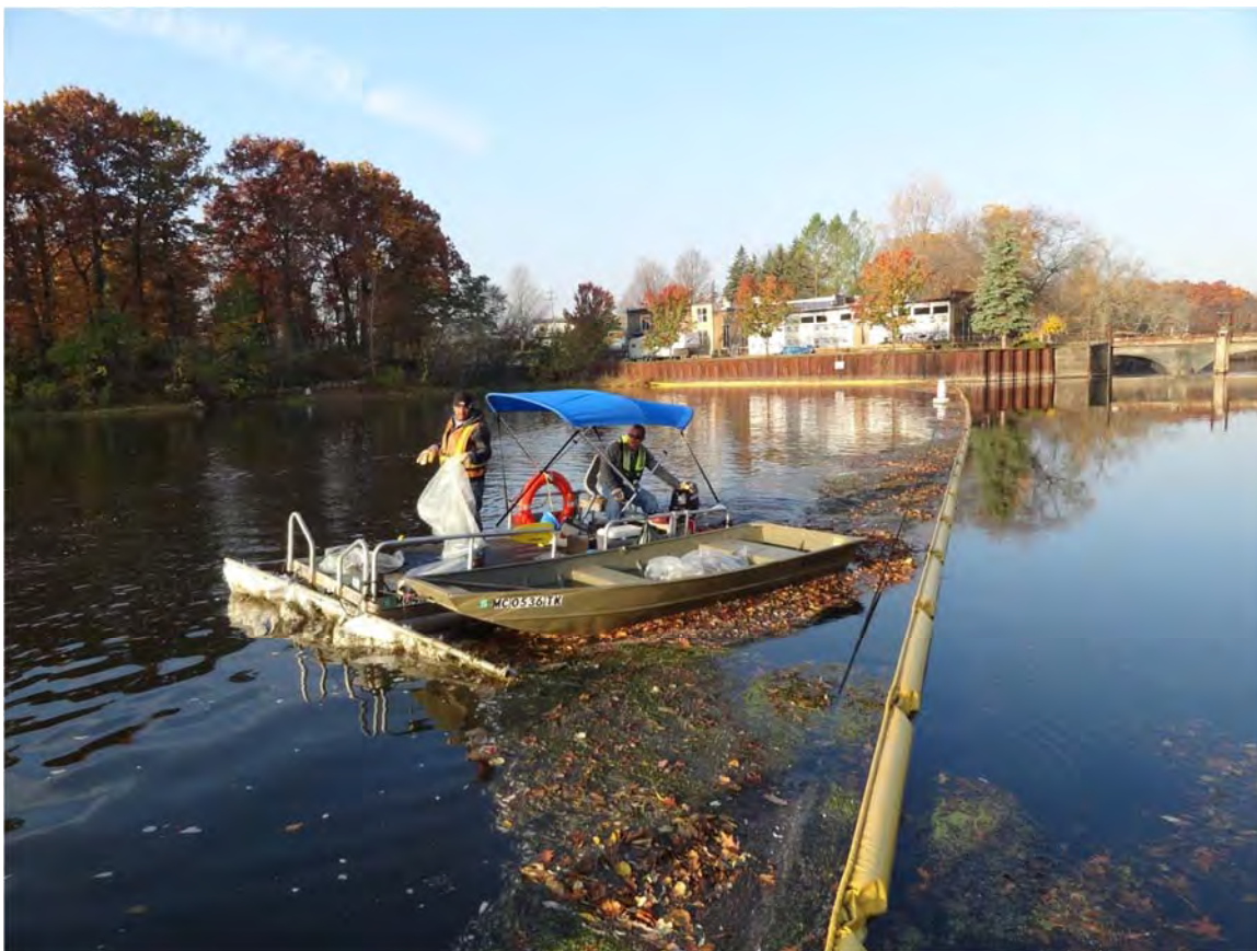
10. Ceresco Dam control point boom observed a crew removing debris from the control point boom.
