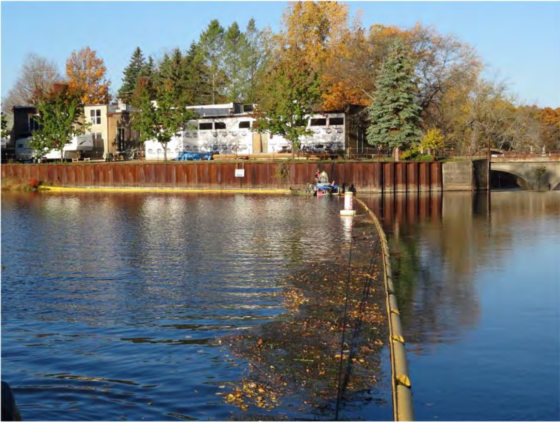
3. Ceresco Dam Control Point Boom observed a crew removing debris from the boom.
