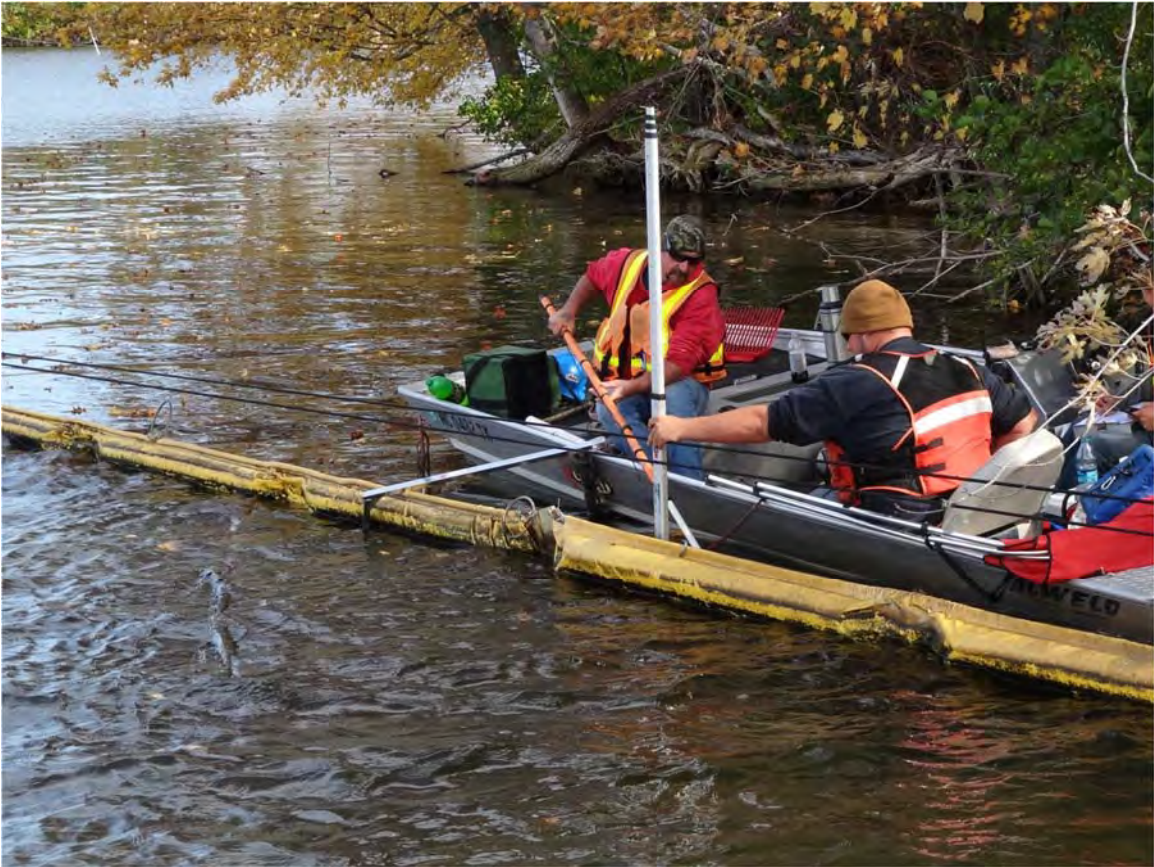
21. Morrow Lake Delta Gate F observed a crew performing curtain monitoring and adjustments.
