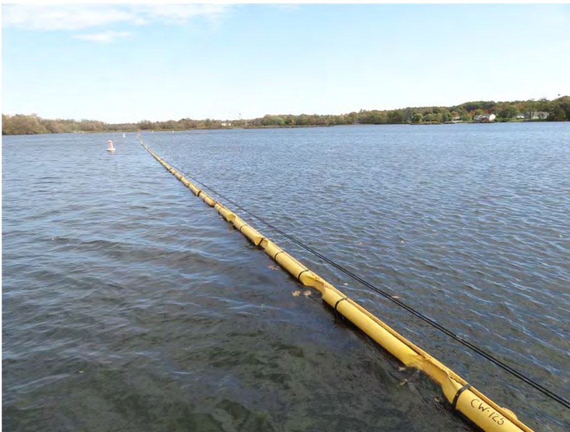
21. Morrow Lake Delta Gate C no sheen observed, extremely windy conditions were experienced
