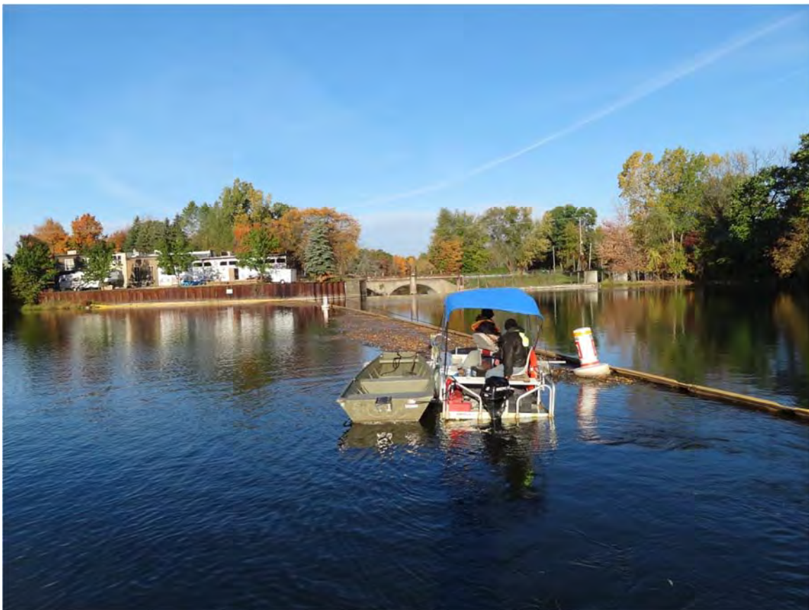
6. Ceresco Dam Control Point observed the boom maintenance crew operating.
