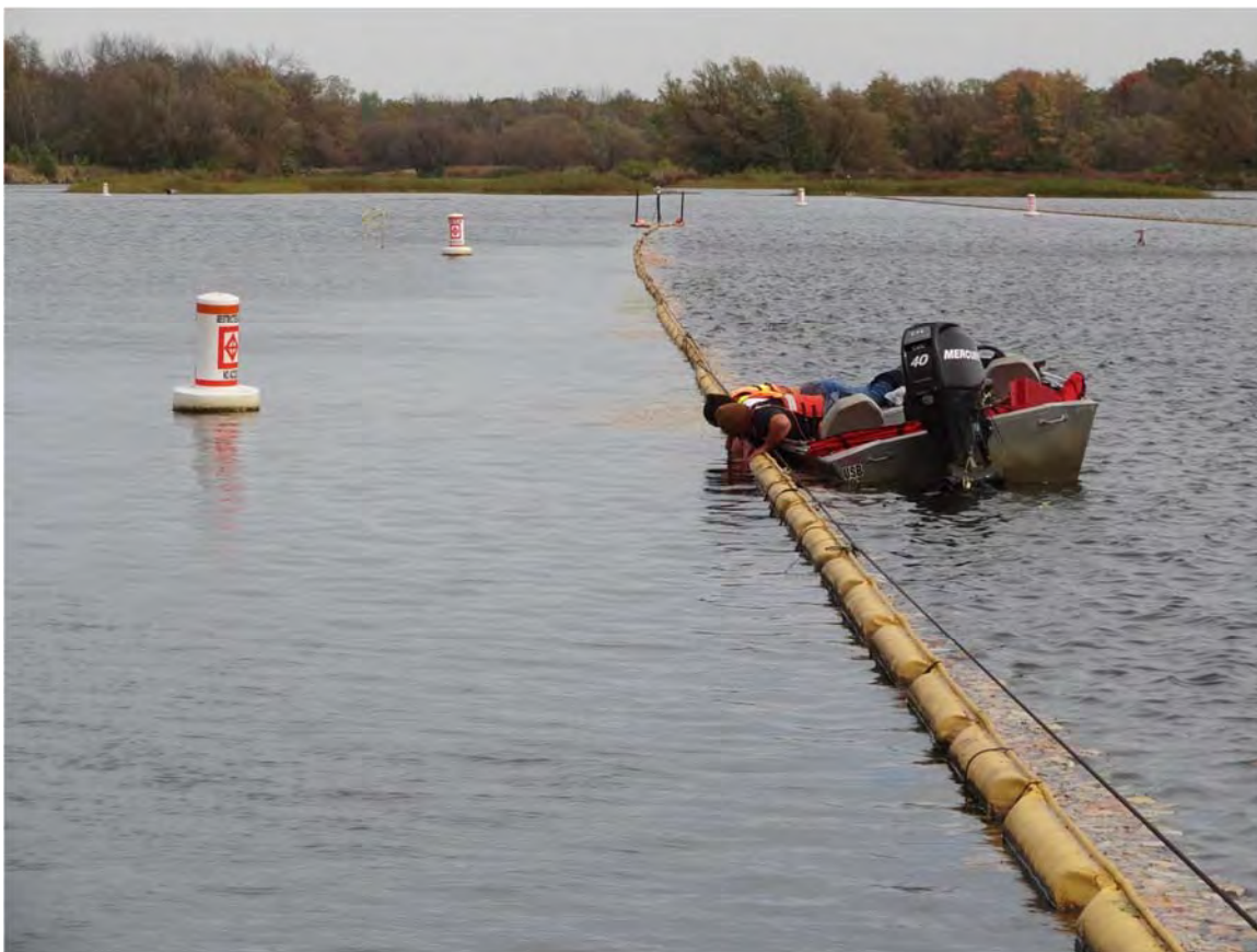
21. Morrow Lake Delta Gate C observed a crew performing curtain maintenance.
