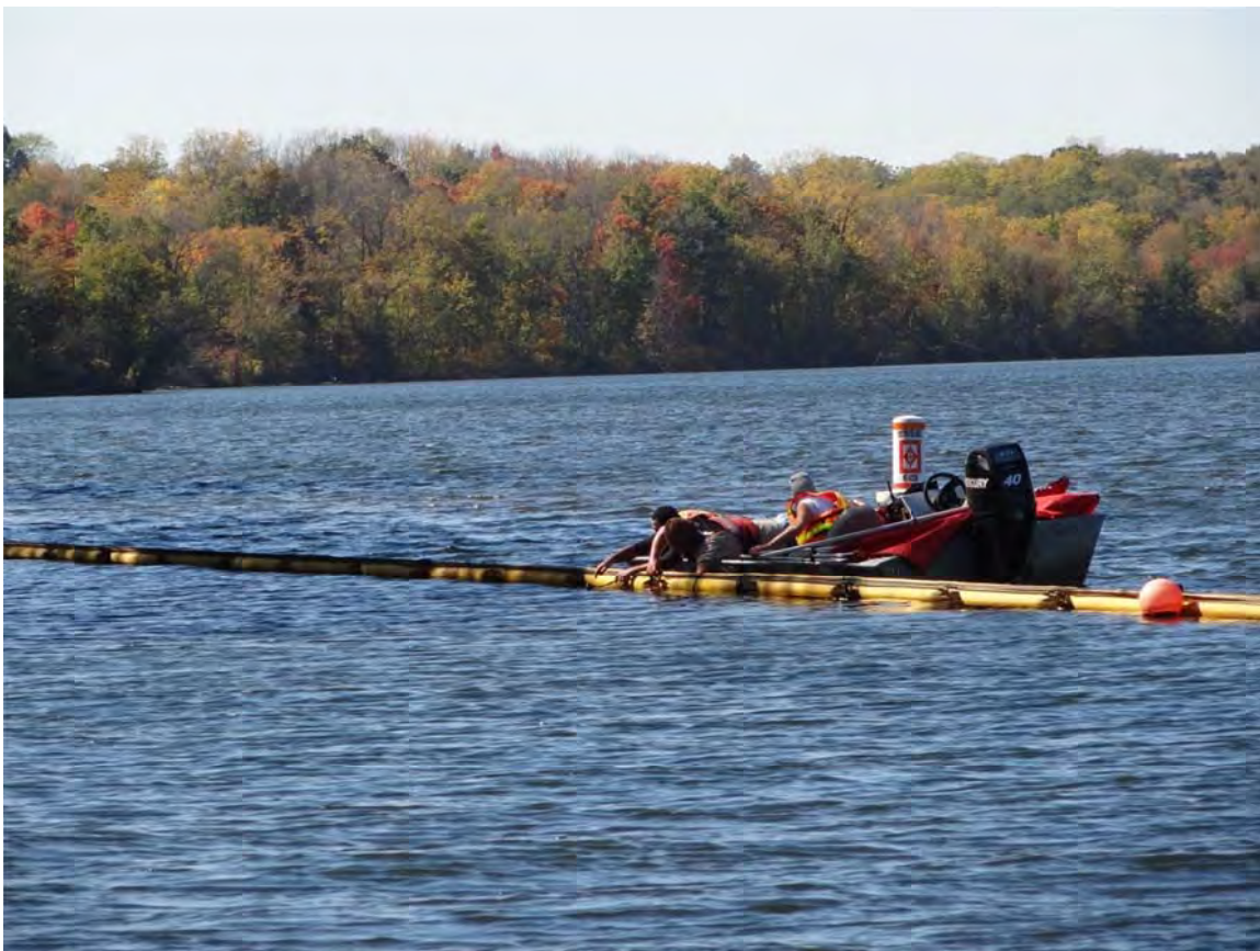
14. Morrow Lake Delta Gate F observed a crew performing adjustments to the curtain.
