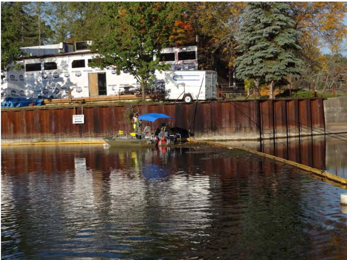
4. Ceresco Dam control point observed the boom maintenance crew.
