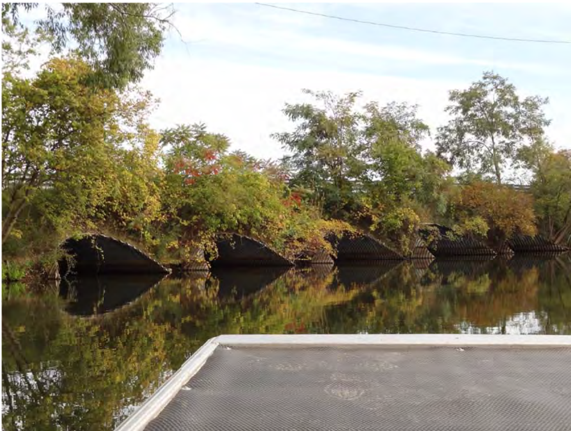
10. View of culverts at MP 15.75 in North Mill Pond. No sheen observed.
