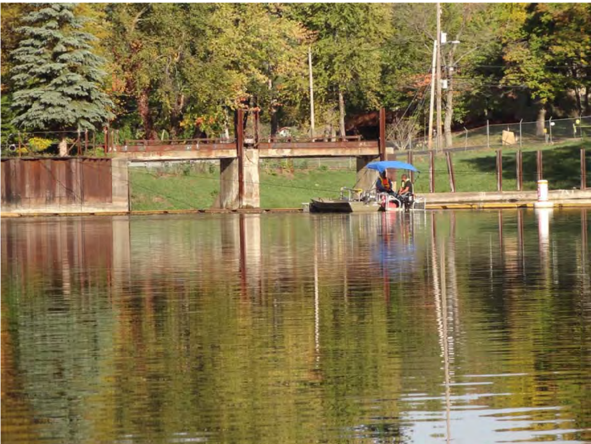
2. Crews removing debris from Ceresco Dam control point.
