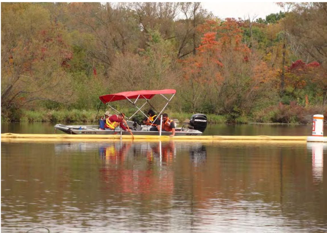
14. Curtain inspection crew observed working along boom E2.
