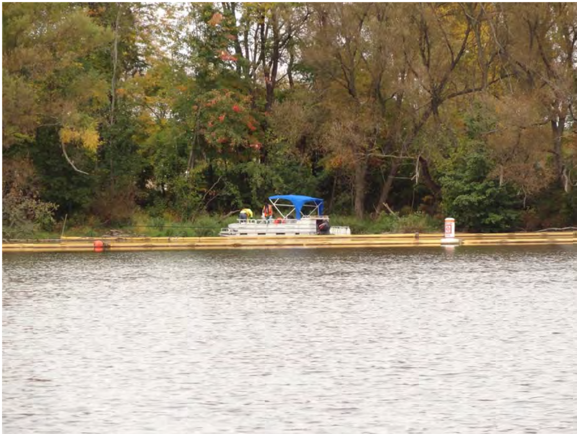
15. Crews removing debris from E2 control point boom in Morrow Lake Delta.
