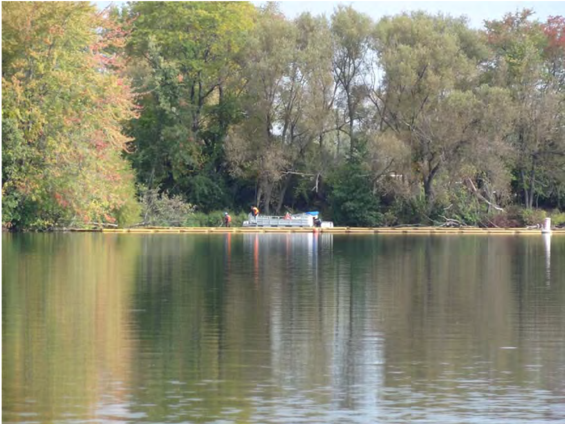
13. Crews removing debris from E4.0 control point in Morrow Lake Delta.
