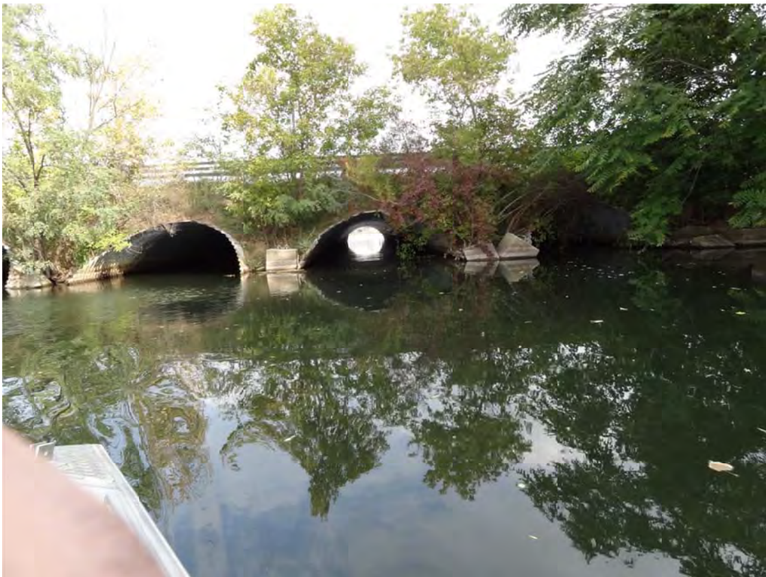
10. Culverts at MP 15.75 (North Mill Pond). No sheen observed.
