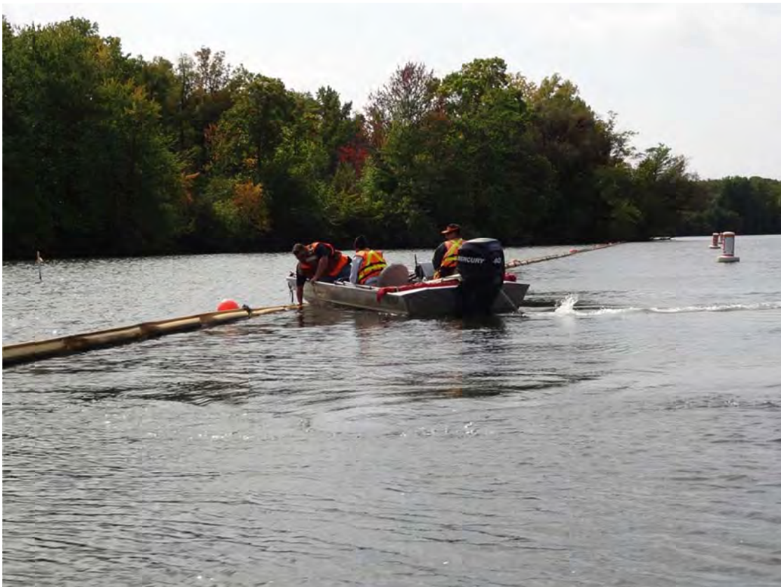
12. Crews inspecting and adjusting sediment curtain boom in Morrow Lake Delta.
