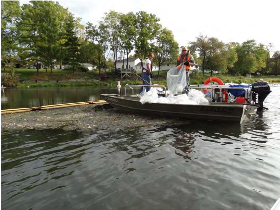
5. Crews removing debris from Ceresco Dam control point.
