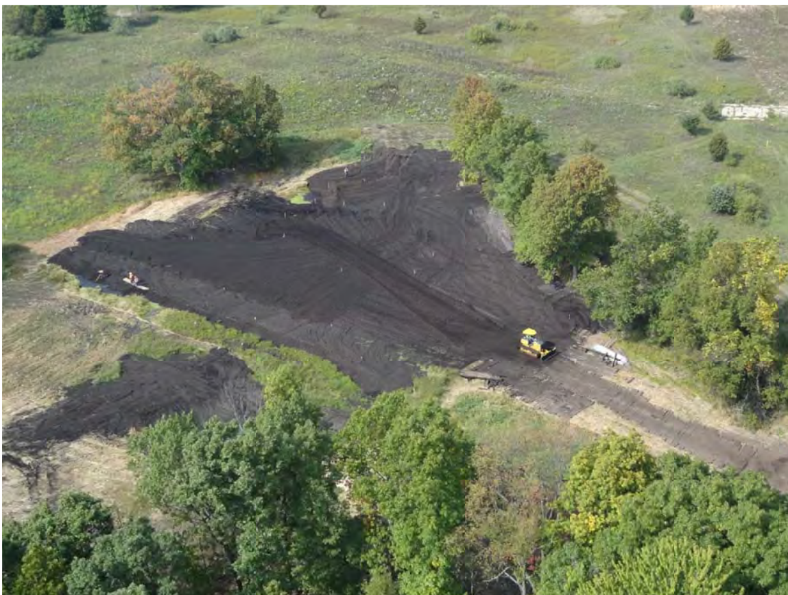
1. Source Area, crews observed grading cover material.
