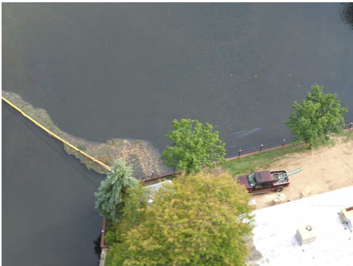
9. Ceresco Dam, sheen observed along impoundment behind containment boom during afternoon overflight.
