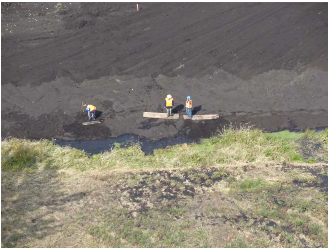
2. Source area, crews observed along southern edge of backfilled area.
