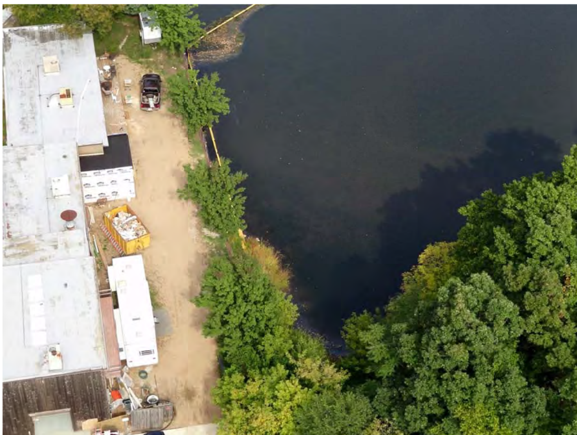
10. Ceresco Dam, observed sheen along impoundment and in southwest corner above dam.
