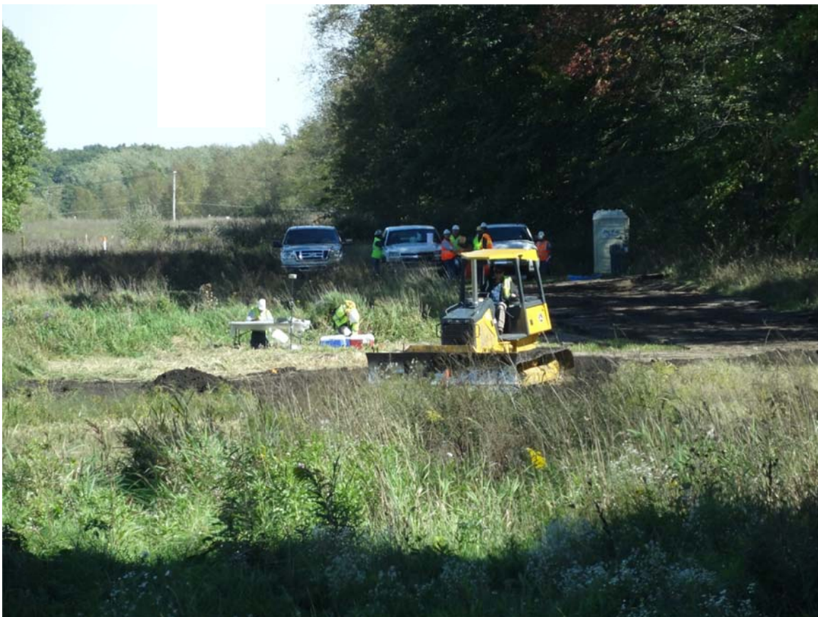
18. Source Area, backfilling activities continue.
