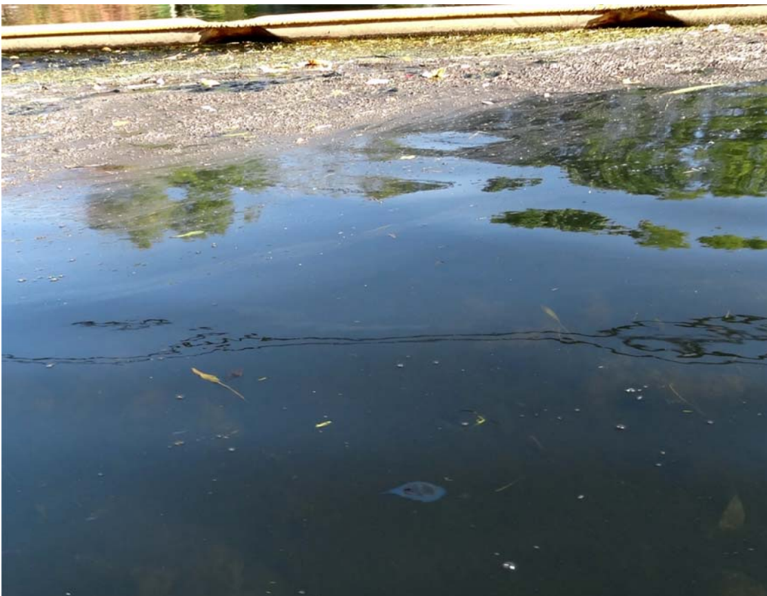
6. Sheen and tar globules observed within Ceresco Dam containment.
