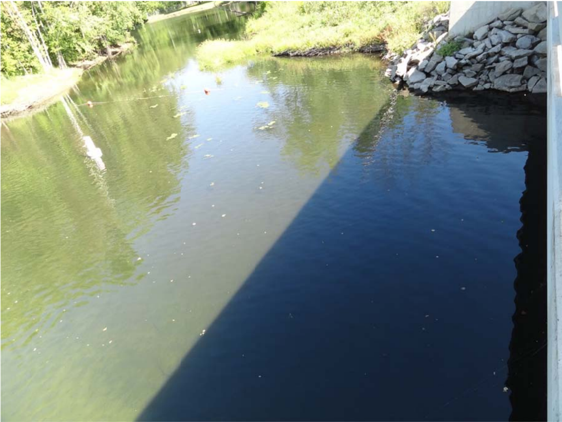
13. MP21.5 Custer Bridge no sheen observed.
