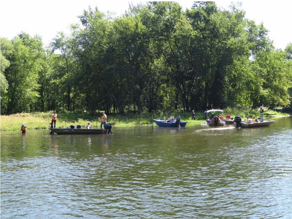
14. MP26.0 RDB observed crews working on the installation of the sediment trap.
