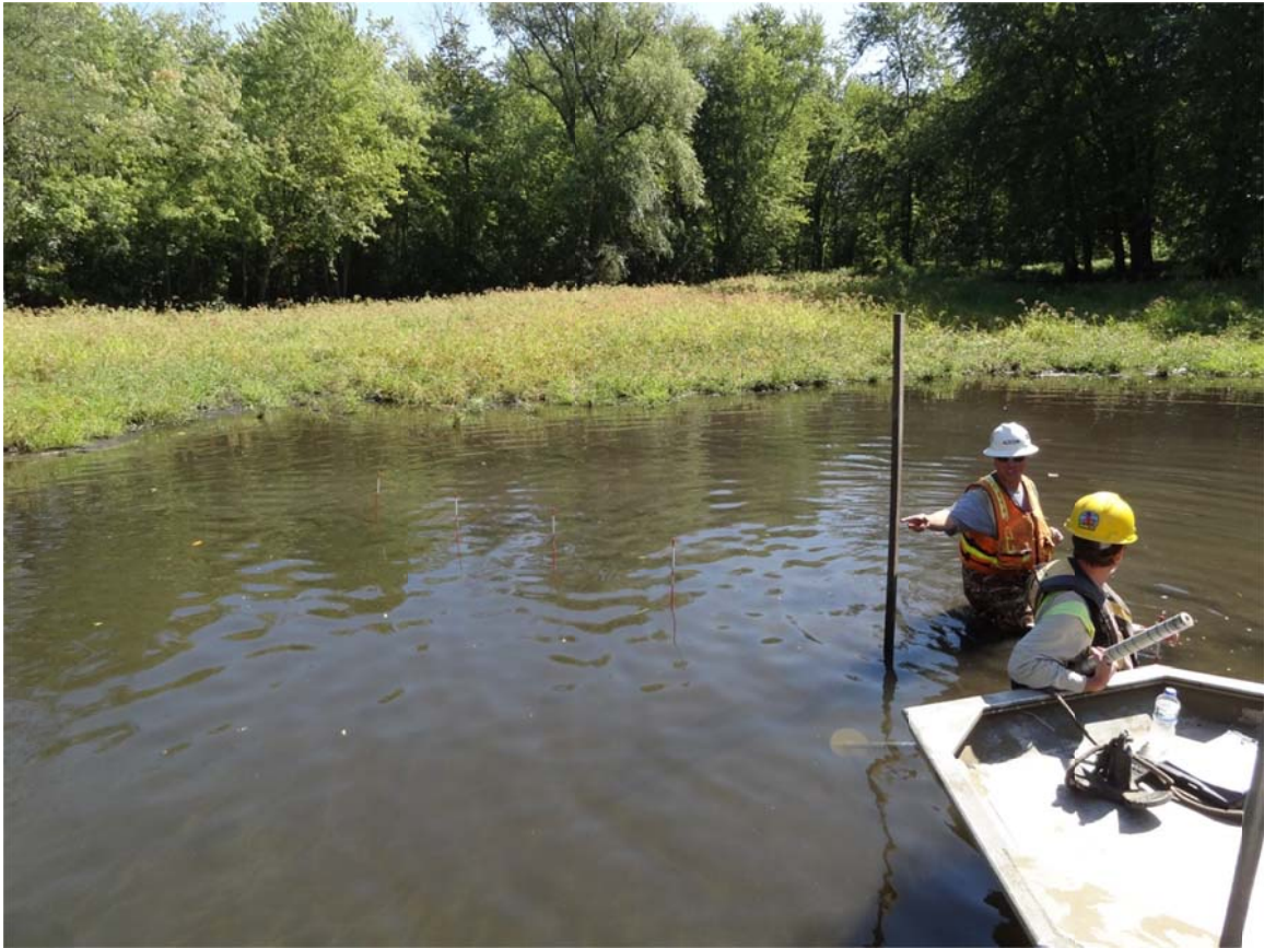
15. MP26.0 RDB observed crews working on the installation of the sediment trap.
