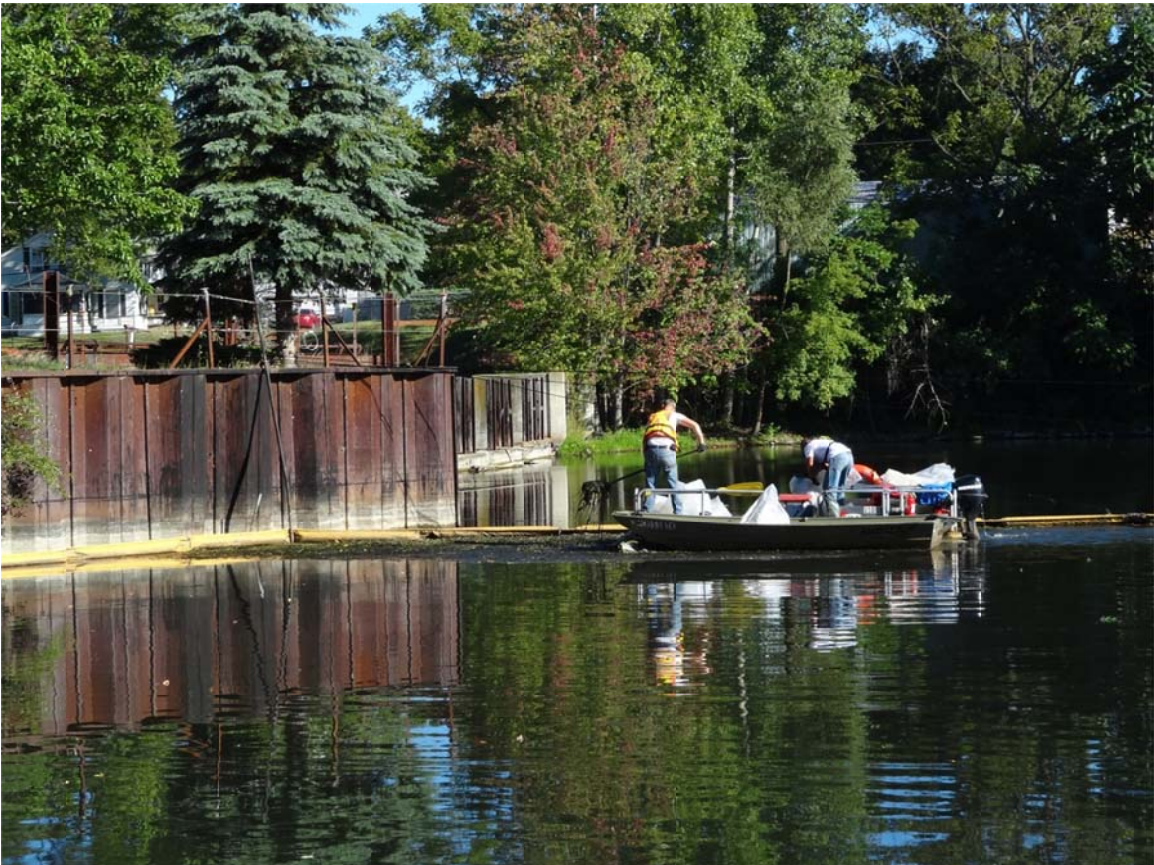
4. Ceresco Dam observed crew removing debris from boom.
