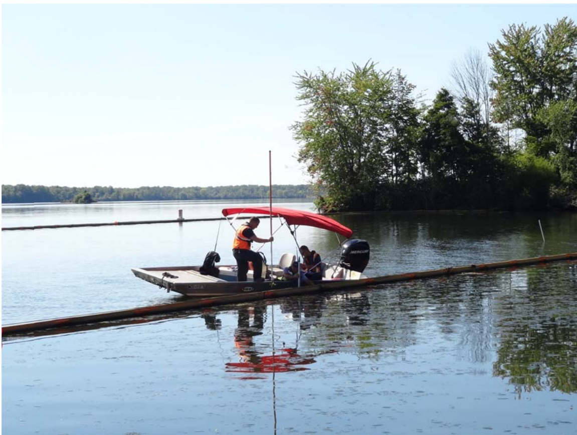
16. Observed a crew performing curtain inspections along Boom E of the Morrow Lake Delta.
