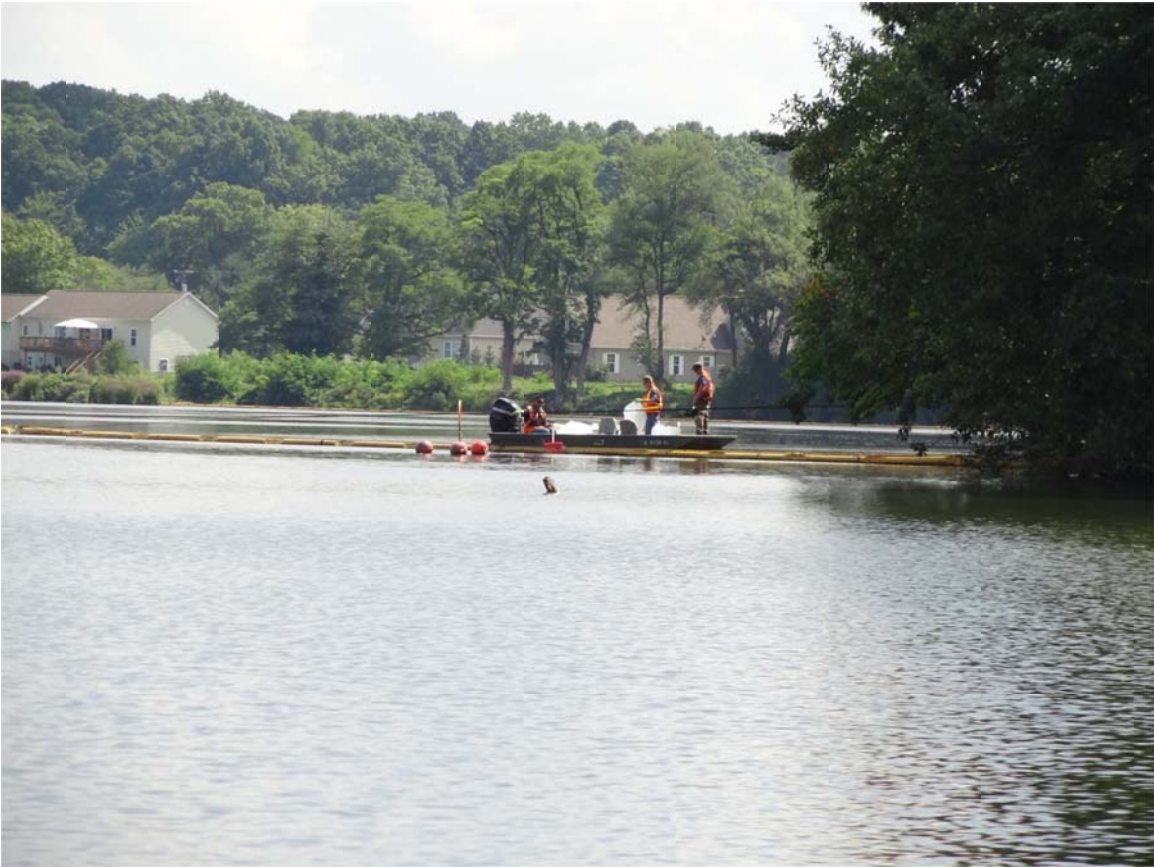
11. Crews observed removing debris from containment configuration C in southwest portion of Morrow Lake Delta.
