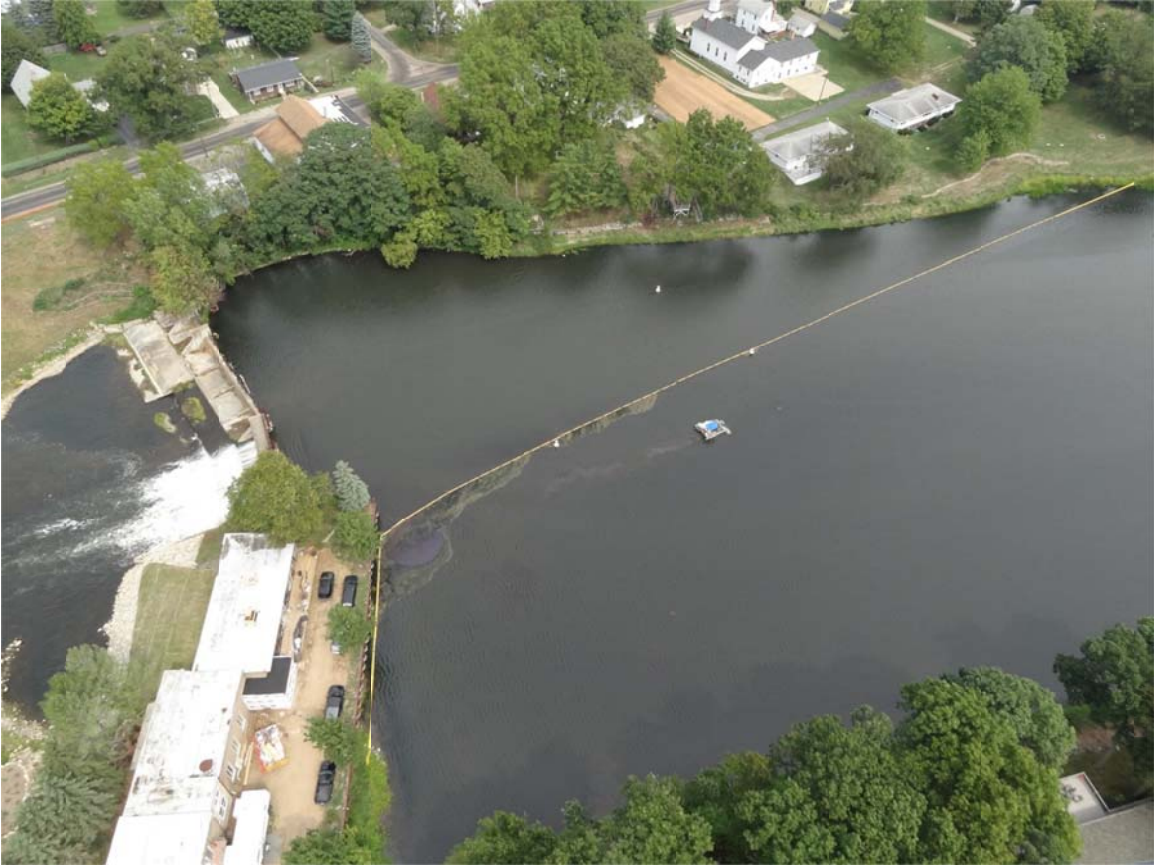
9. Ceresco Dam, observed sheen sweeper observed collecting sheen within containment.
