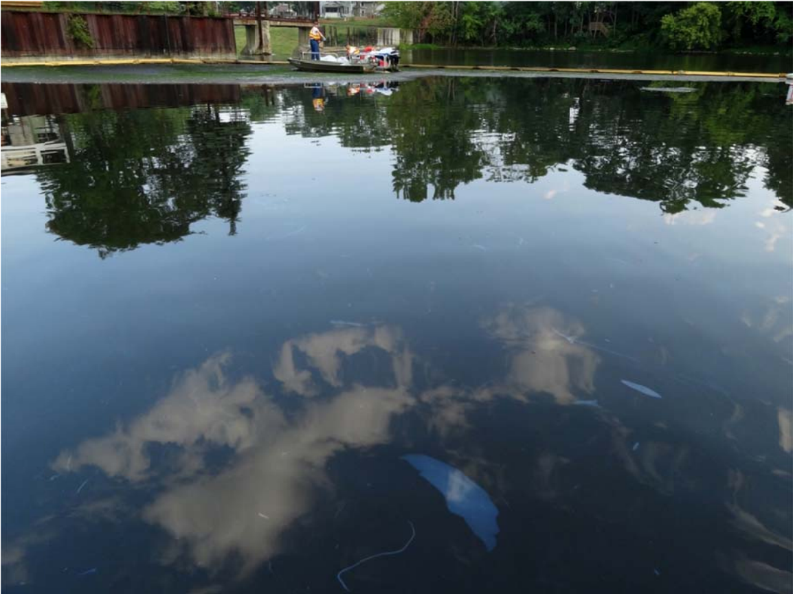
7. Ceresco Dam, observed sheen and crew removing debris from the control point.
