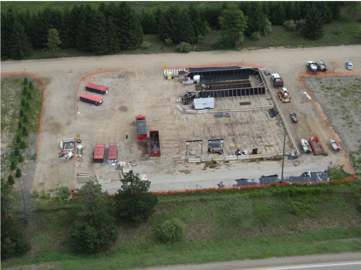
2. Frac Tank City decontamination pad, containment boom staged in decon pad.
