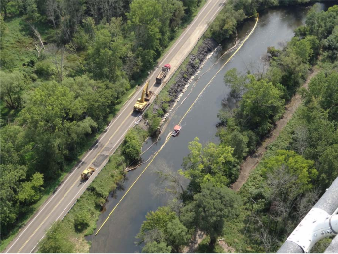
11. Shoreline restoration work observed along west side of Raymond Road.
