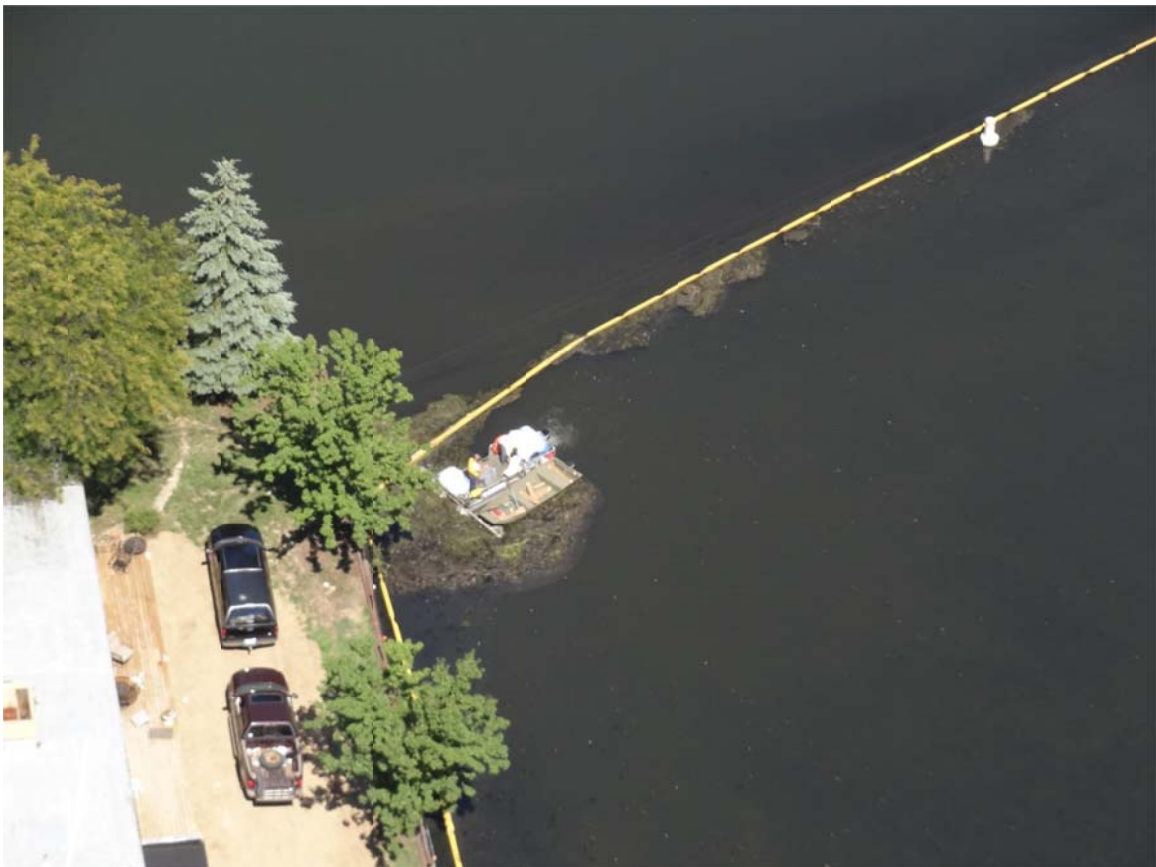
16. Ceresco Dam observed crew removing debris from the control point.
