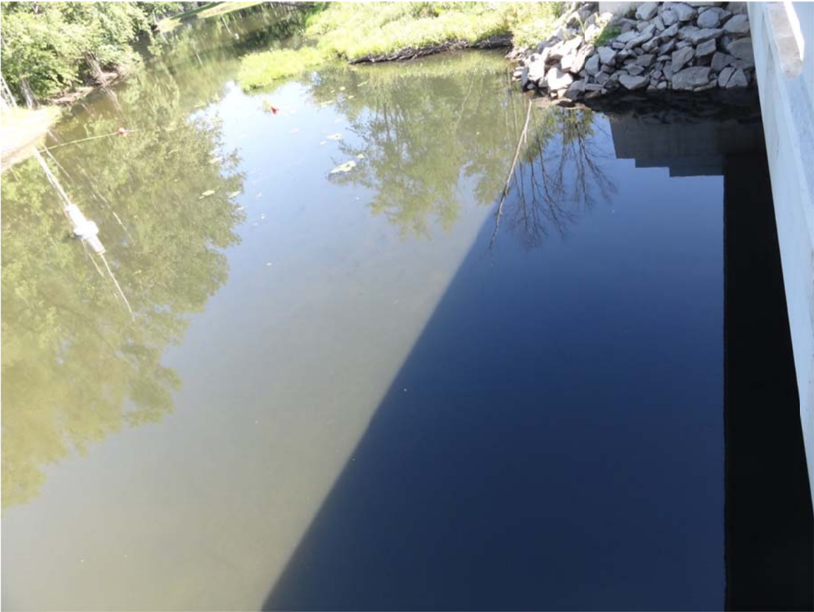
13. MP 21.5 Custer Bridge no sheen observed.
