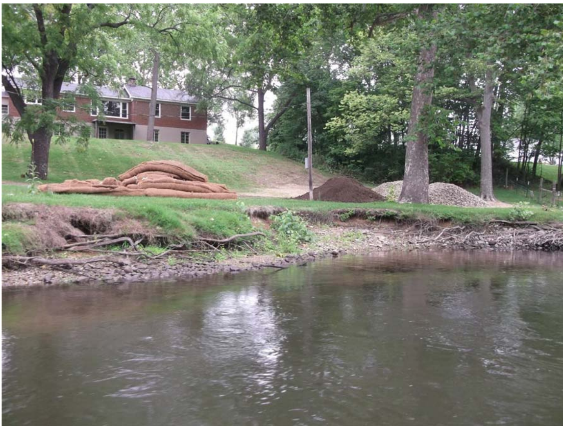
17. MP27.0 RDB observed shoreline restoration.
