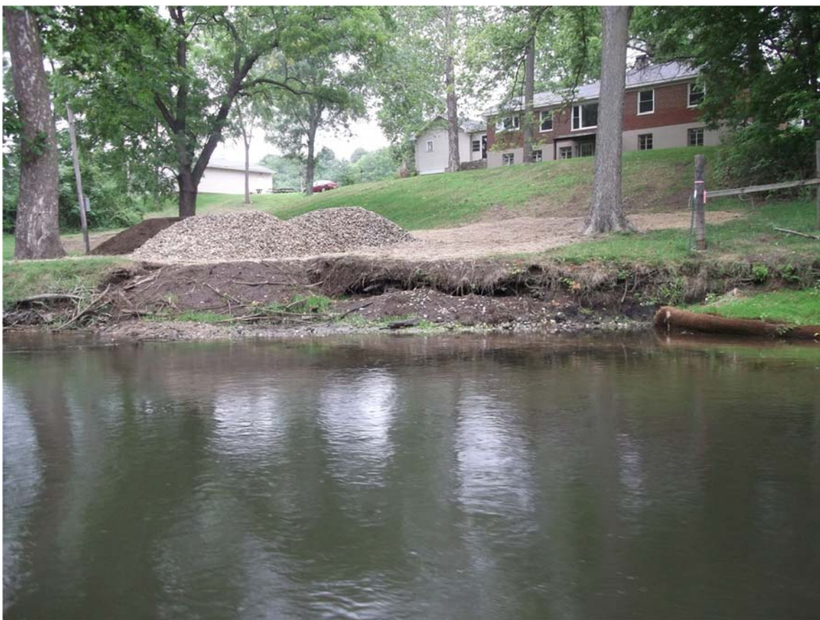
18. MP27.0 RDB observed shoreline restoration.
