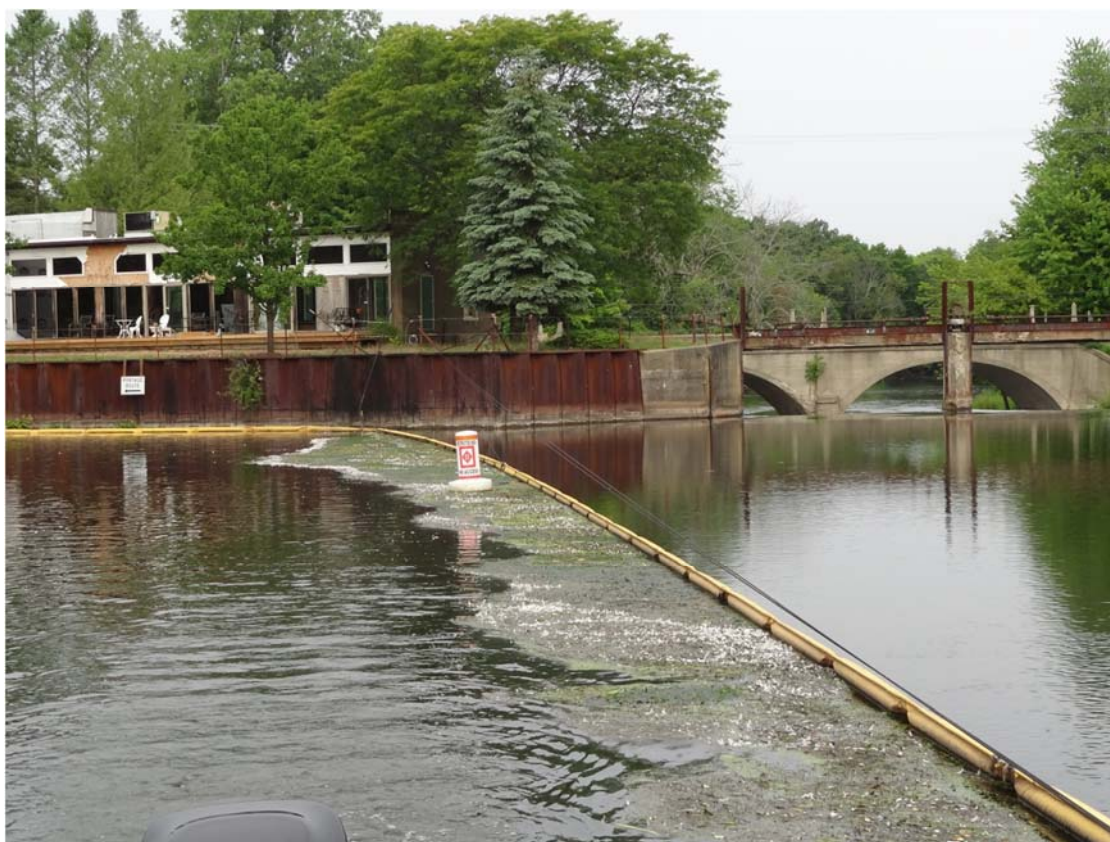
6. Ceresco Dam control point boom, observed sheen and debris collecting along the boom.
