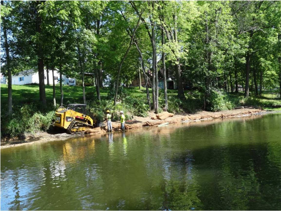
11. MP27.0 RDB observed river bank erosion restoration work.
