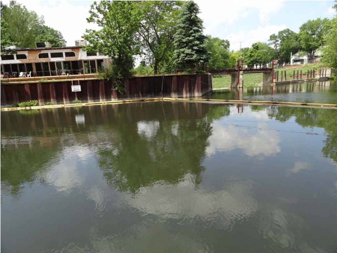
23. Ceresco Dam control point boom, observed the debris removed from the boom.
