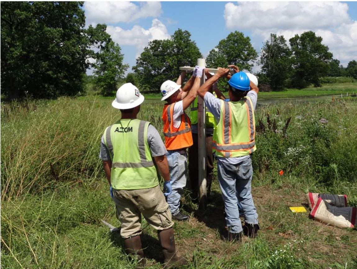
26. Source area observed crew pulling well casing.
