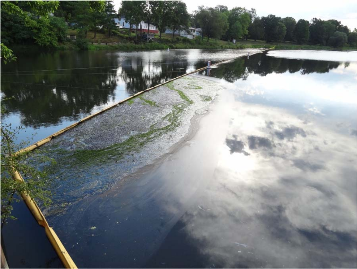
1. Ceresco Dam Control Point Boom, debris observed prior to boom maintenance crew arriving.
