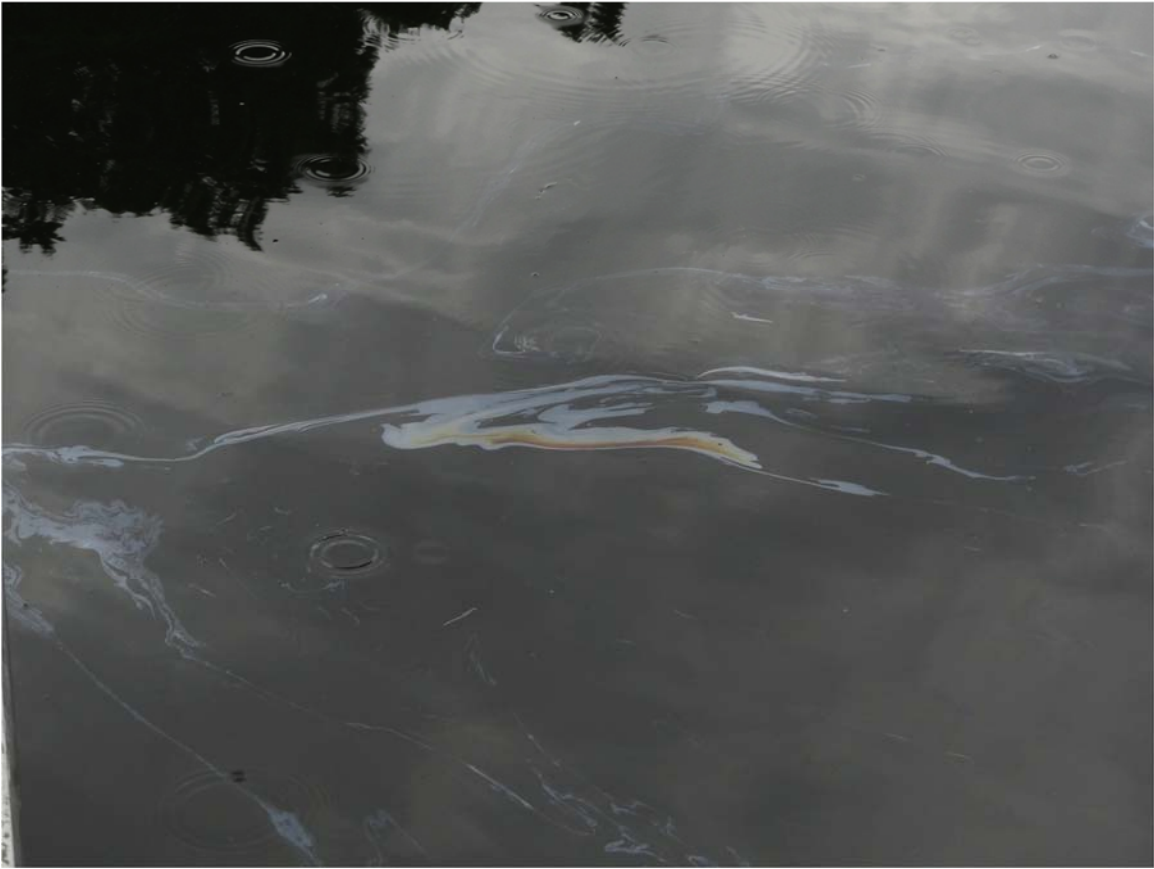
5. Ceresco Dam sheen observed.
